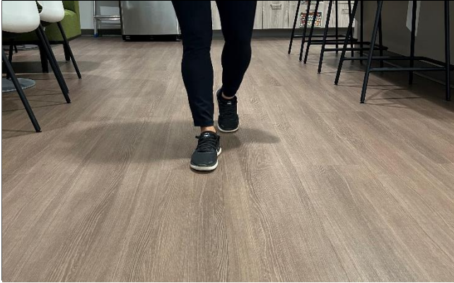
Fig. 1: Example of slip-resistant flooring
