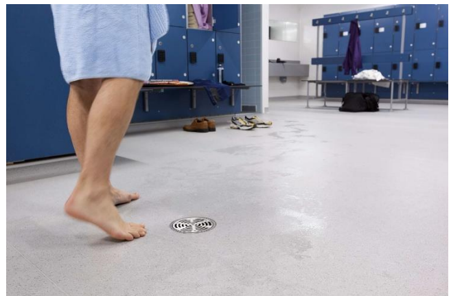
Fig. 2: Slip-resistant flooring example from Altro
