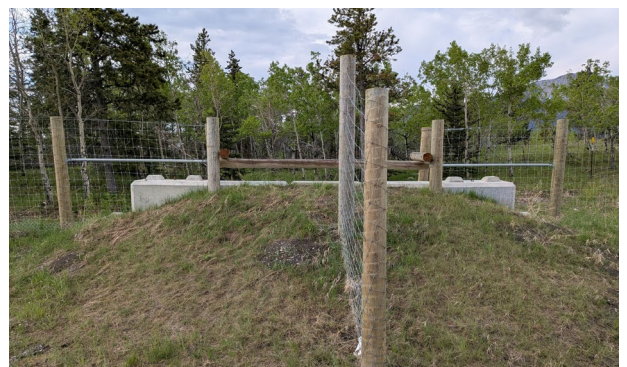
Animals can use the ramp to get back over the fence, while the concrete block side helps keep them from getting back onto the highway.
