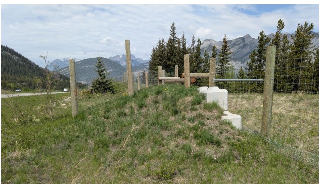
Jump outs are designed and constructed to allow animals trapped between the highway and wildlife fence to safely leave the area.
