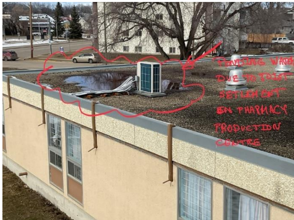
Fig. 3 (Above): Roof water ponding, Barrhead Healthcare Centre
