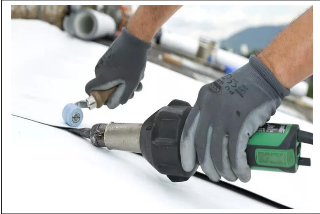
Fig. 1: PVC membrane being detailed with hot air welder (Used with permission by Sika).
