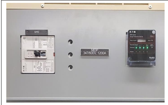
Fig. 1: 347/600V 1200A Main Distribution Panel with Type 2 SPD
