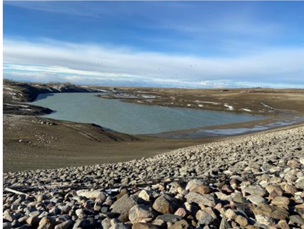
View from the top of the dam
