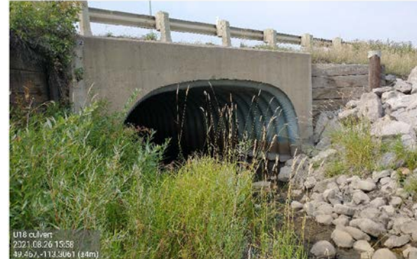
PHOTO 2 LEFT BANK UPSTREAM LOOKING AT CULVERT
