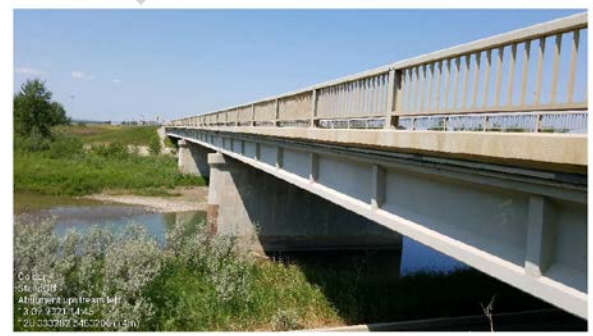
PHOTO 2 RIGHT BANK UPSTREAM LOOKING AT BRIDGE
