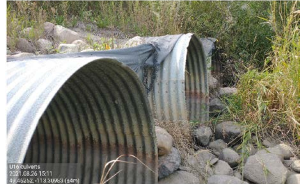
PHOTO 2 RIGHT BANK DOWNSTREAM LOOKING AT CULVERT
