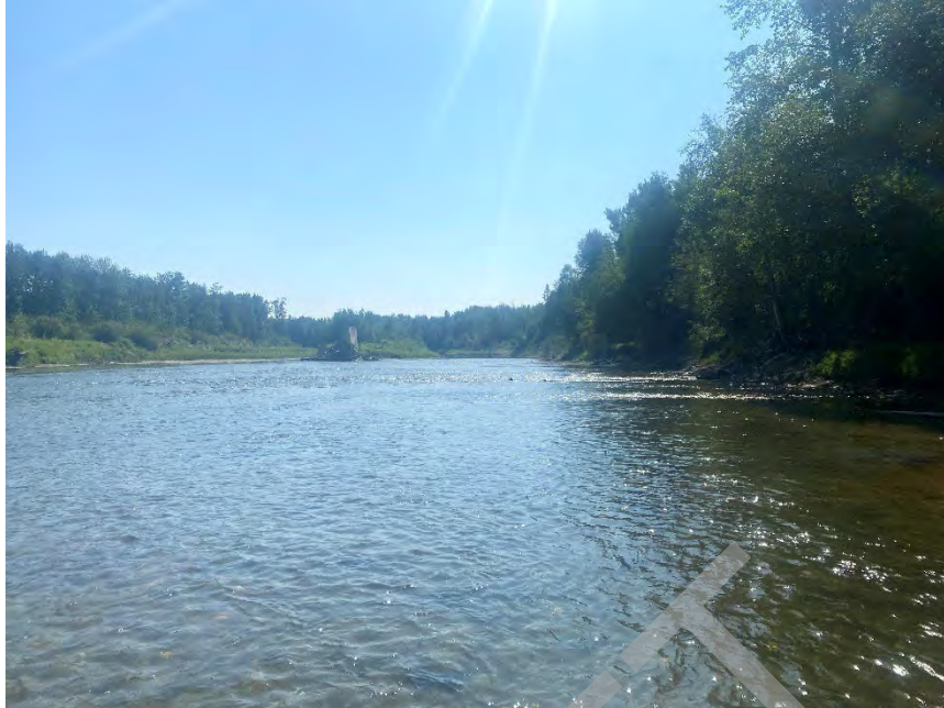
Pembina River (downstream view) looking at the CN Rail abandoned pier near River Station 3,367 m.
