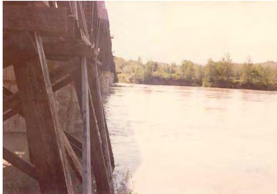
1980 Flood at CN Railway Bridge near Sangudo
