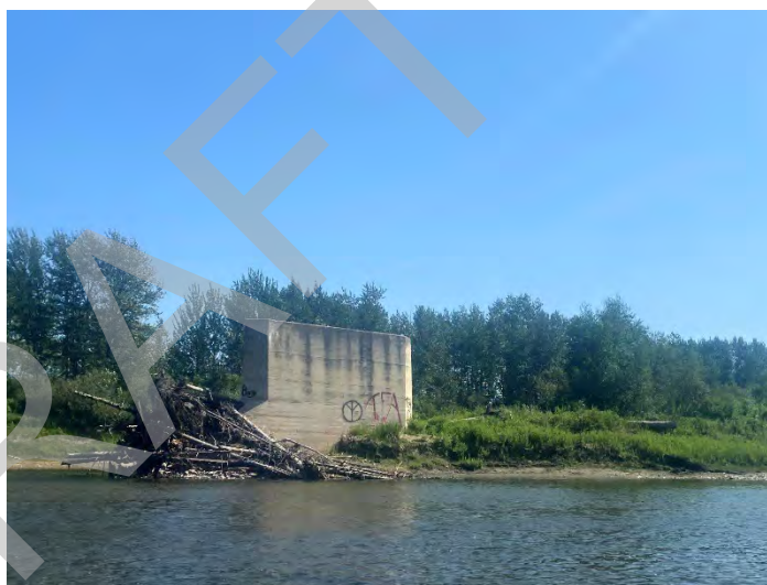
Looking at the pier from the right bank of the river
