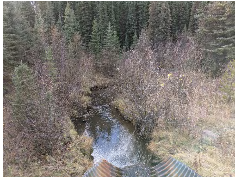
1) Looking upstream on Bryan creek from Highway 47 Culvert.
