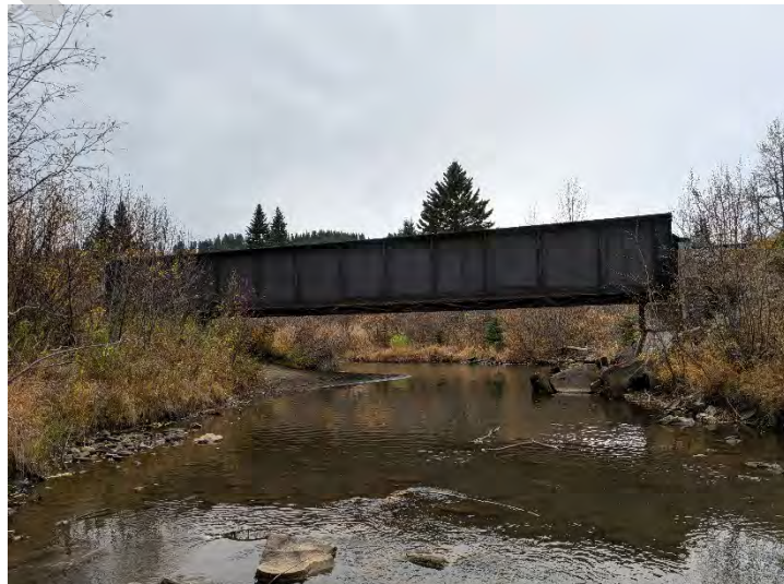
Looking upstream at the downstream side of the bridge
