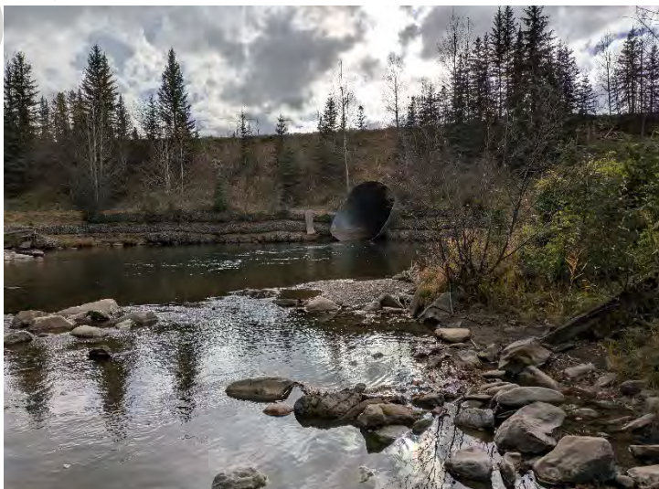
Looking upstream on the downstream side of the culvert
