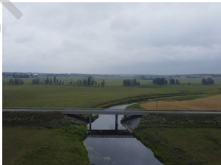
Looking upstream on the downstream side of the bridge
