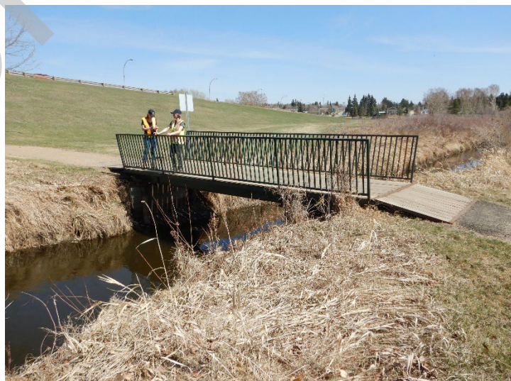
Looking upstream on downstream side of the bridge
