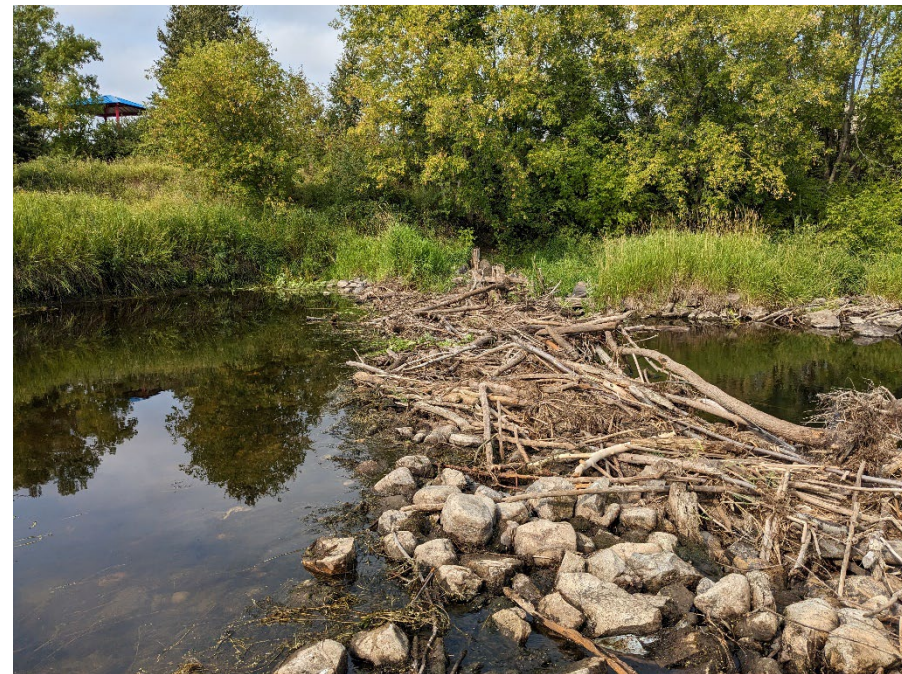
4) Looking along alignment of old dam on Battle River near RS 9228.
