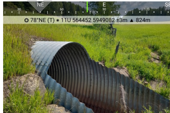
PHOTO 2 CULVERT 2, LOOKING DOWNSTREAM
