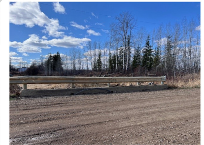
PHOTO 3 TOP OF THE DECK
