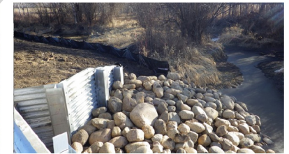
PHOTO 3 TOP OF DECK, LOOKING DOWNSTREAM
