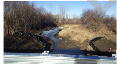
PHOTO 2 TOP OF DECK, LOOKING UPSTREAM
