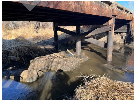
PHOTO 2 RIGHT BANK, LOOKING UPSTREAM
