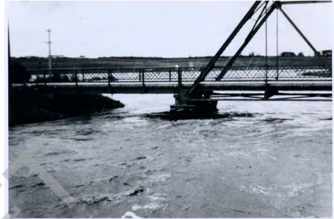
1948 Flood: Looking downstream at old Highway 4 bridge (June 18, 1948)
