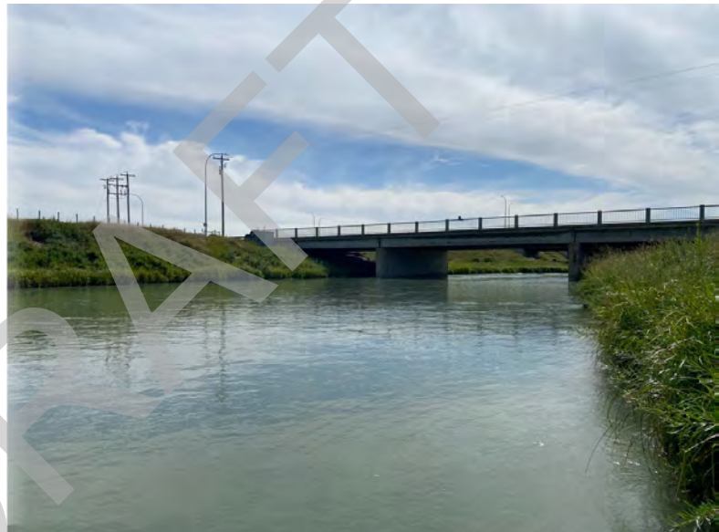
Looking downstream portion of the bridge from left bank
