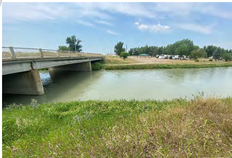
Looking downstream portion of the bridge from right bank
