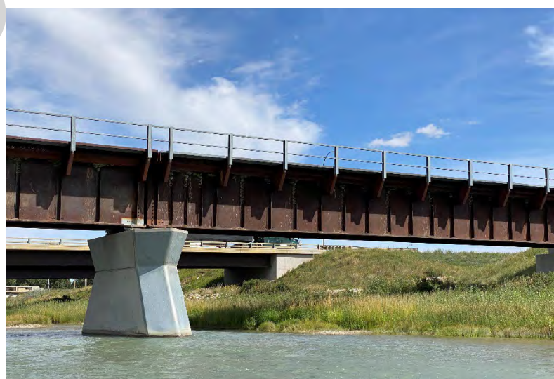
Looking at bridge pier from upstream side and left bank
