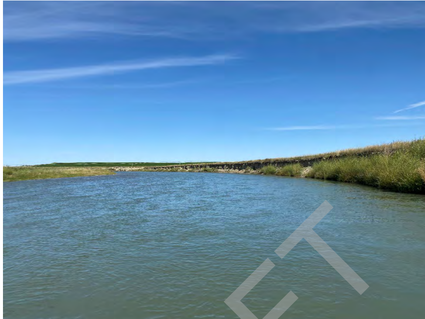
Milk River (downstream view) from middle of channel near River Station 7,476.10 m (XS-53).
