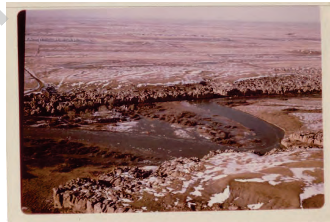
1965 Flood: Looking north over Writing-on-Stone campground showing irrigation pump house surrounded and water upto camp shelter
