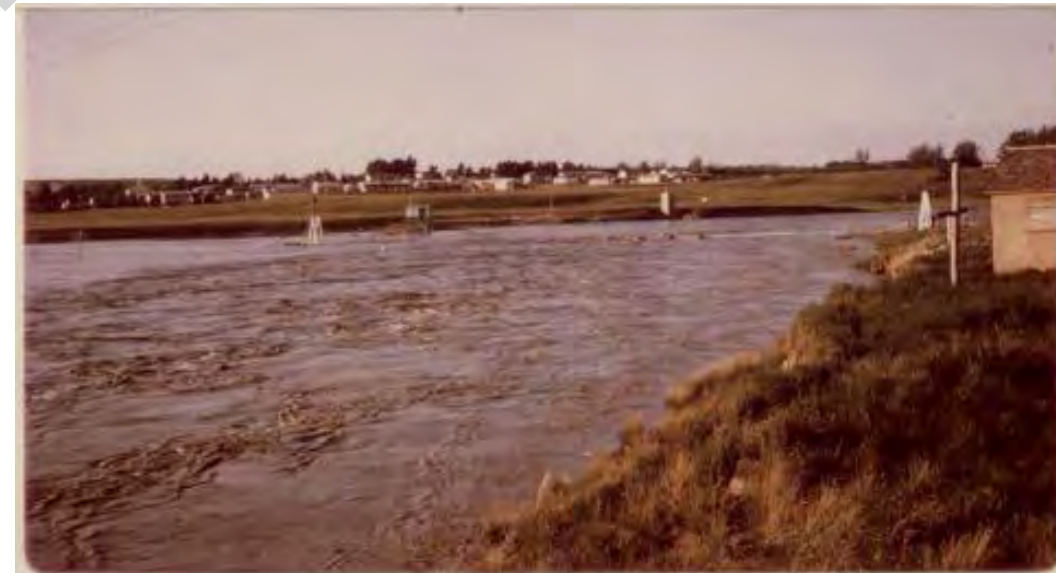
1964 Flood: Pipeline under water at Milk River
