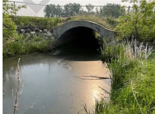
PHOTO 2 VIEW OF BRIDGE FROM DOWNSTREAM
