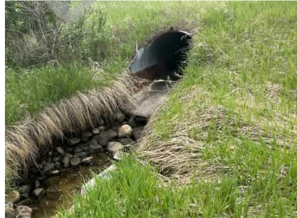
PHOTO 2 VIEW UPSTREAM TO CULVERT
