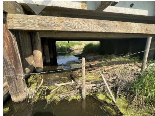
PHOTO 2 VIEW OF BRIDGE FROM DOWNSTREAM
