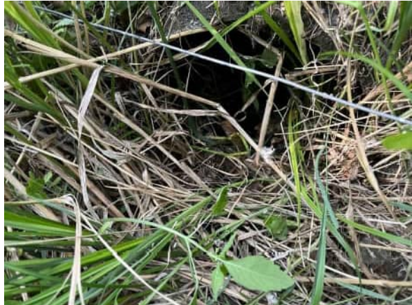
PHOTO 1 VIEW OF CULVERT FROM UPSTREAM
