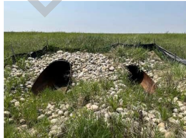
PHOTO 2 VIEW OF CULVERT FROM DOWNSTREAM
