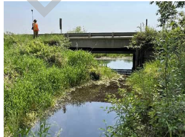
PHOTO 2 VIEW OF BRIDGE FROM DOWNSTREAM
