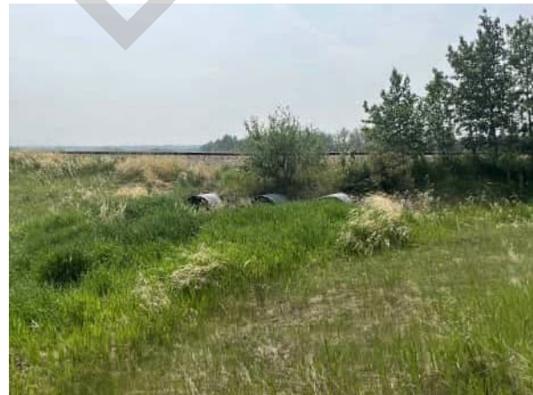
PHOTO 2 VIEW UPSTREAM TO CULVERTS
