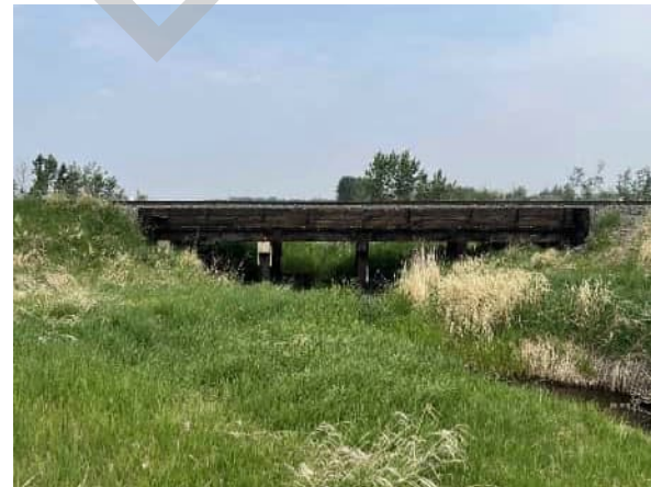
PHOTO 2 VIEW UPSTREAM TO BRIDGE
