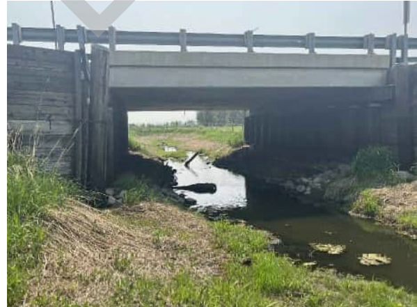
PHOTO 2 VIEW OF BRIDGE FROM DOWNSTREAM
