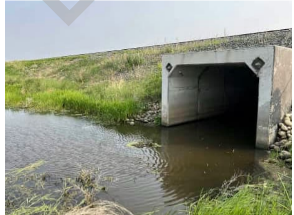
PHOTO 2 VIEW FROM DOWNSTREAM
