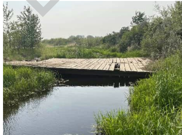
PHOTO 2 VIEW OF BRIDGE FROM DOWNSTREAM
