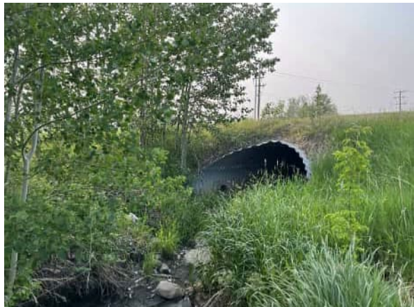
PHOTO 1 VIEW FROM UPSTREAM
