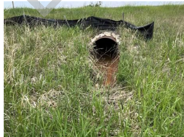
PHOTO 2 VIEW UPSTREAM (NORTH) TO EAST CULVERT
