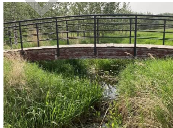
PHOTO 2 VIEW OF BRIDGE FROM DOWNSTREAM
