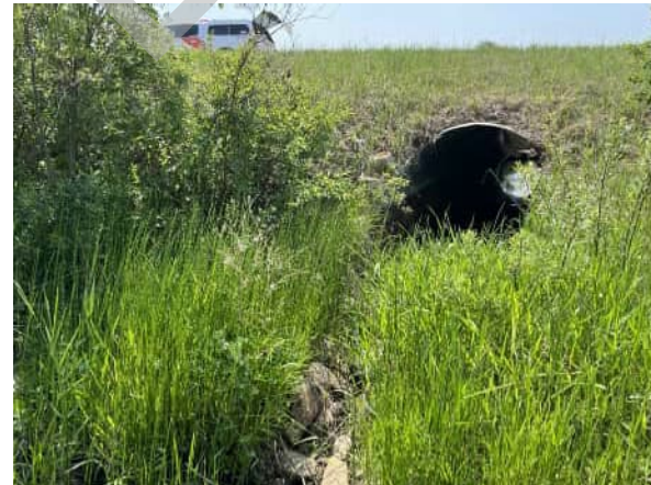
PHOTO 2 WEST CULVERT VIEW FROM DOWNSTREAM
