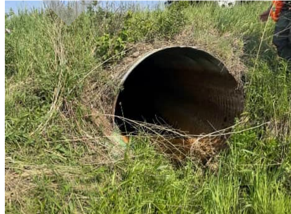
PHOTO 2 VIEW UPSTREAM TO SOUTH CULVERT
