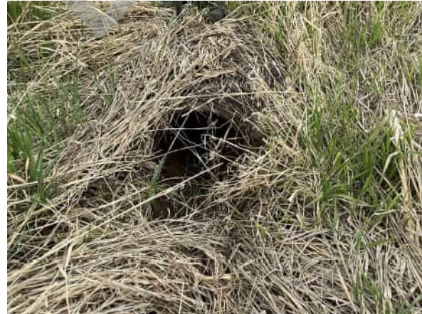
PHOTO 2 VIEW UPSTREAM (EAST) TO CULVERT OUTLET
