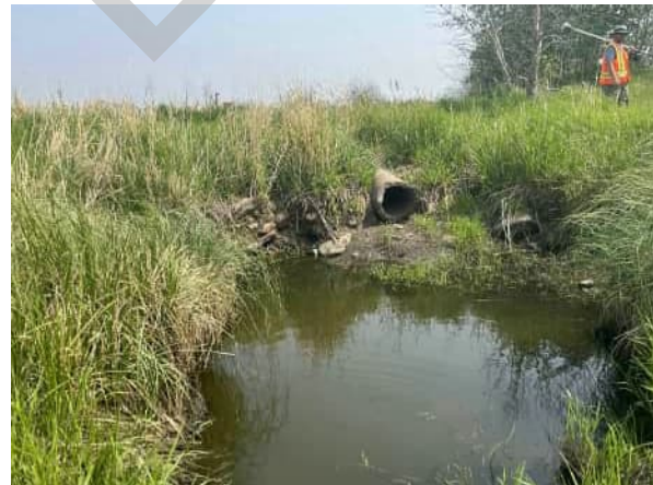
PHOTO 2 VIEW FROM DOWNSTREAM
