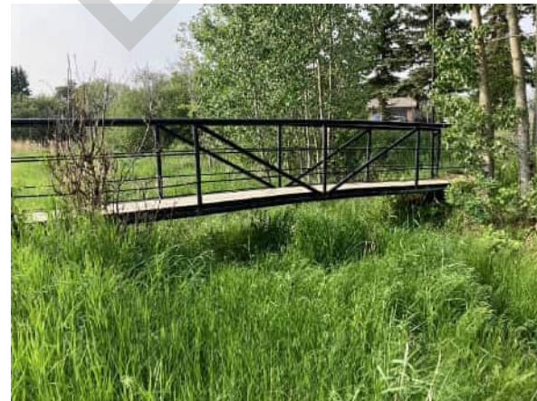
PHOTO 2 VIEW OF BRIDGE FROM DOWNSTREAM
