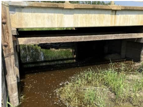
PHOTO 1 VIEW OF BRIDGE FROM UPSTREAM
