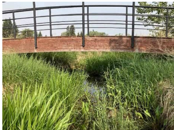
PHOTO 1 VIEW OF BRIDGE FROM UPSTREAM
