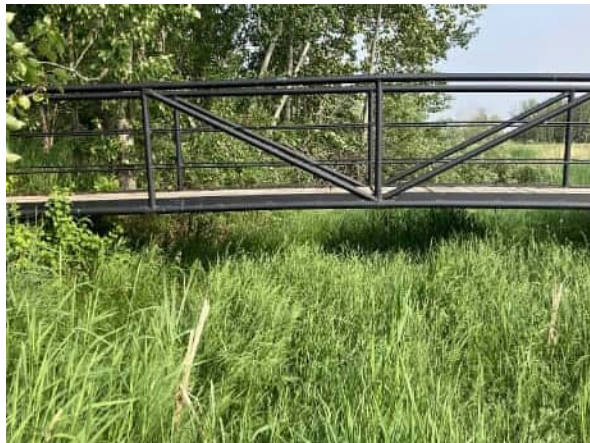
PHOTO 1 VIEW OF BRIDGE FROM UPSTREAM
