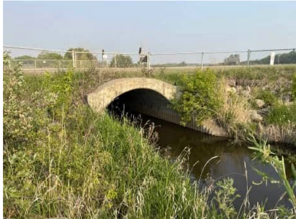
PHOTO 1 VIEW OF BRIDGE FROM UPSTREAM
