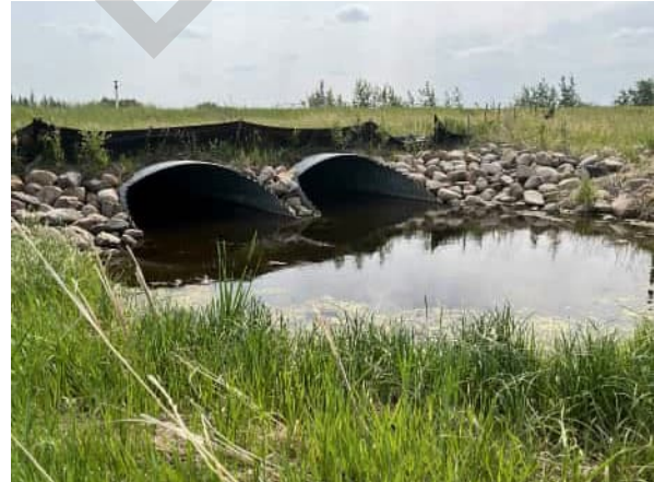
PHOTO 2 VIEW OF CULVERTS FROM DOWNSTREAM
