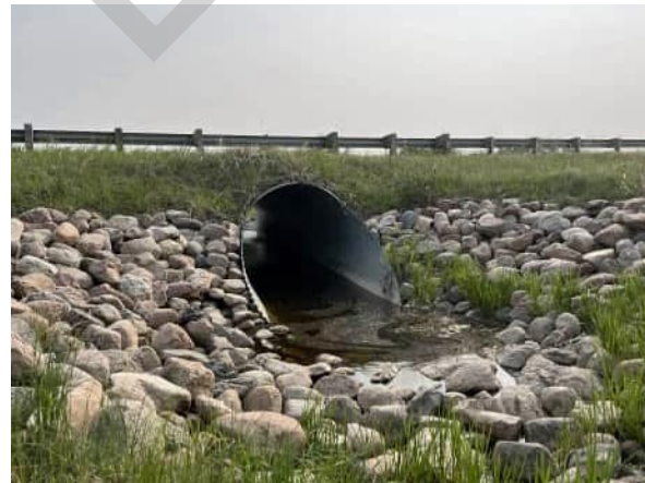
PHOTO 2 VIEW FROM DOWNSTREAM
