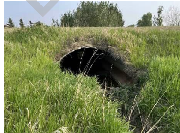
PHOTO 2 VIEW FROM DOWNSTREAM
