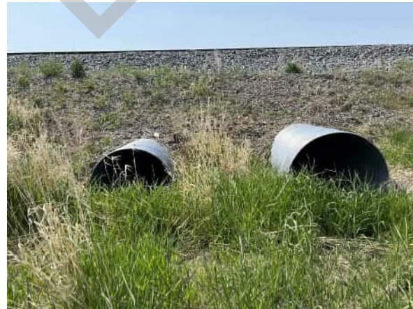
PHOTO 2 VIEW OF CULVERTS FROM DOWNSTREAM
