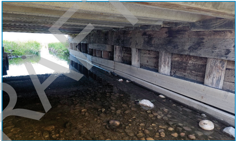
Left abutment looking upstream:
