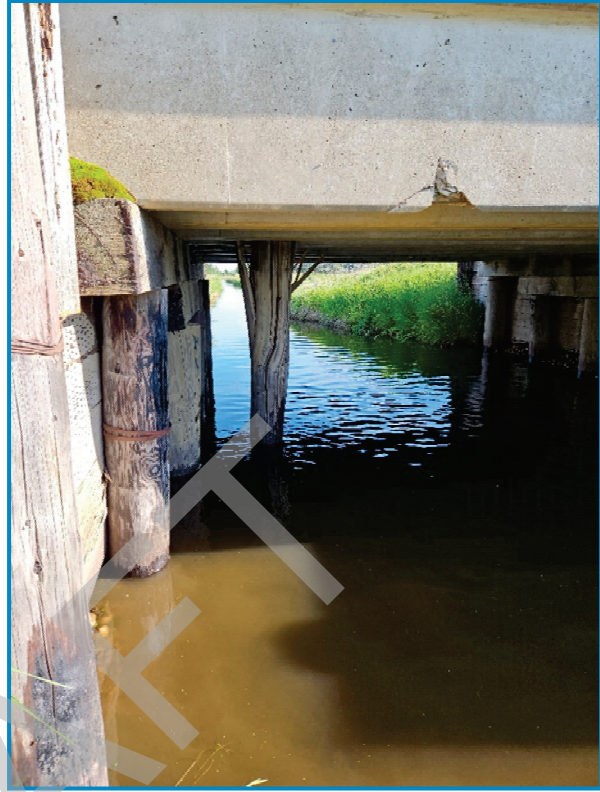
Random pile from downstream right bank:
