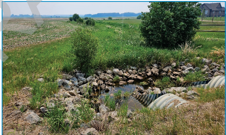
Looking upstream from right shoulder:
