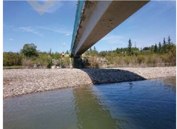
PHOTO 2 LEFT BANK, ABUTMENT
