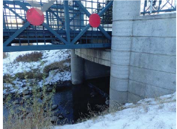
PHOTO 2 RIGHT BANK, ABUTMENT
