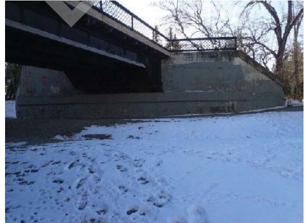
PHOTO 2 RIGHT BANK, ABUTMENT
