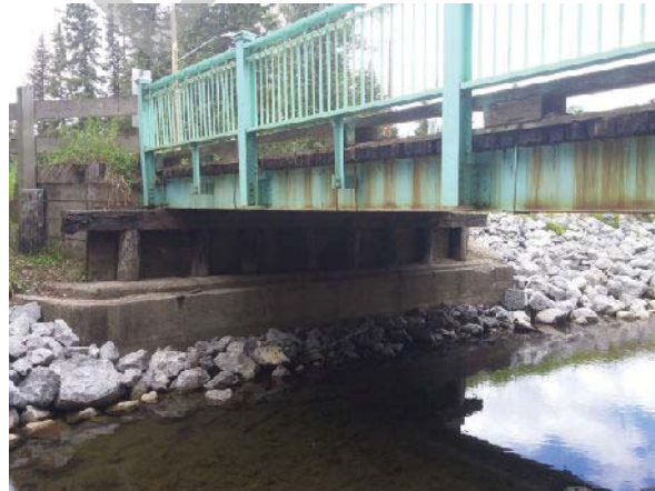
PHOTO 2 RIGHT BANK, ABUTMENT
