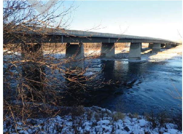
PHOTO 2 LEFT BANK, LOOKING DOWNSTREAM
