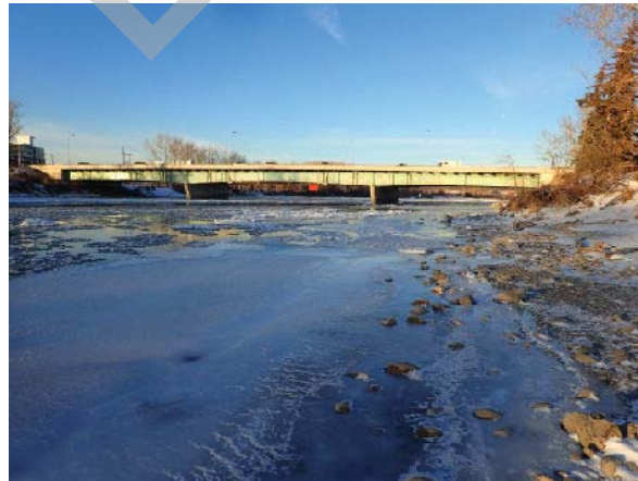
PHOTO 2 LEFT BANK, LOOKING UPSTREAM
