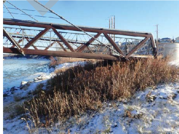
PHOTO 2 LEFT BANK, LOOKING UPSTREAM
