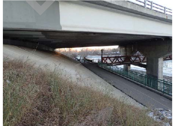
PHOTO 2 LEFT BANK, ABUTMENT
