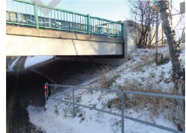
PHOTO 2 RIGHT BANK, ABUTMENT
