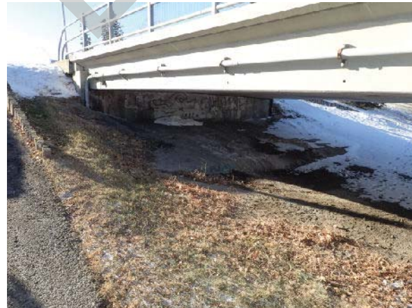
PHOTO 2 RIGHT BANK, ABUTMENT
