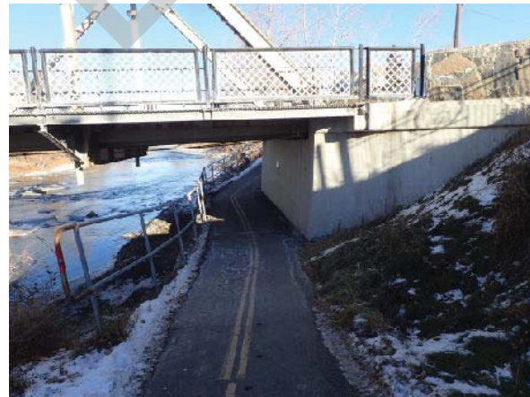
PHOTO 2 RIGHT BANK, ABUTMENT
