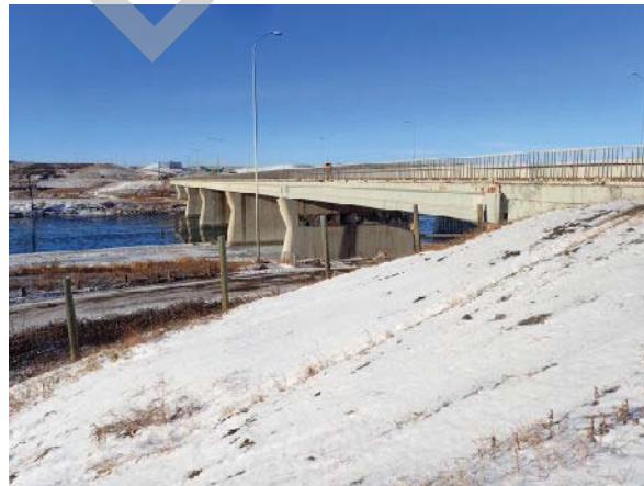
PHOTO 2 LEFT BANK, LOOKING UPSTREAM
