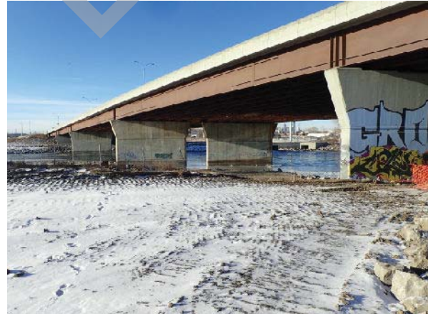
PHOTO 2 LEFT BANK, LOOKING UPSTREAM
