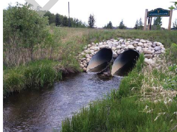
PHOTO 2 LEFT BANK, LOOKING DOWNSTREAM
