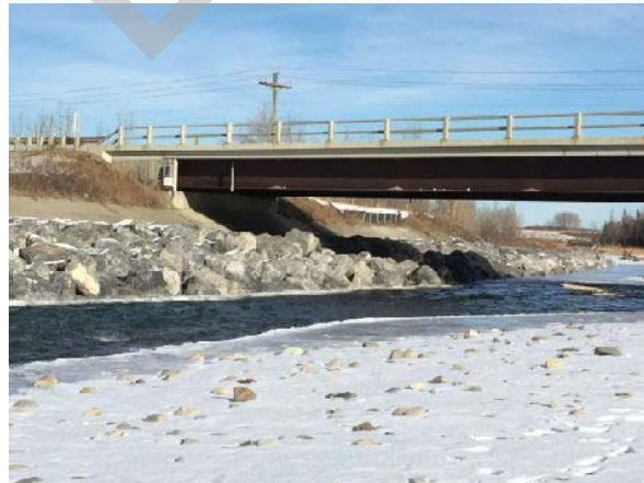
PHOTO 2 LEFT BANK, ABUTMENT
