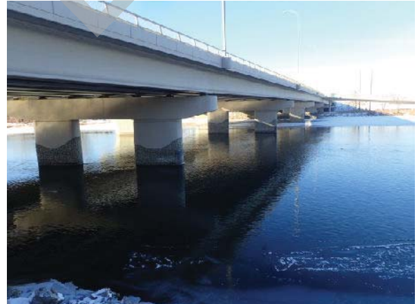
PHOTO 2 LEFT BANK, LOOKING DOWNSTREAM
