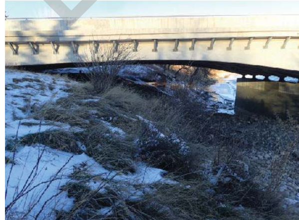
PHOTO 2 RIGHT BANK, ABUTMENT
