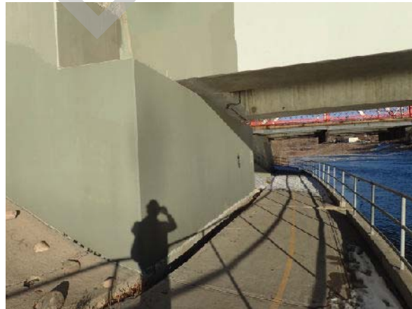
PHOTO 2 RIGHT BANK, ABUTMENT
