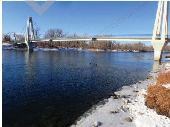
PHOTO 2 LEFT BANK, LOOKING UPSTREAM
