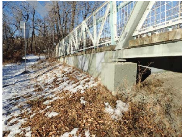
PHOTO 2 LEFT BANK, ABUTMENT
