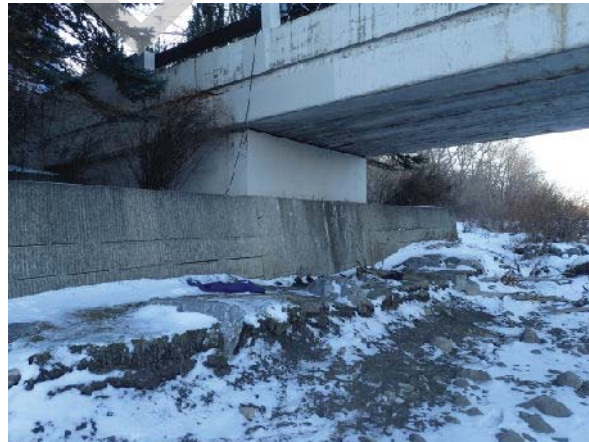
PHOTO 2 RIGHT BANK, ABUTMENT
