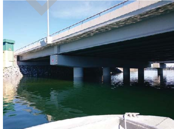
PHOTO 2 LEFT BANK, ABUTMENT
