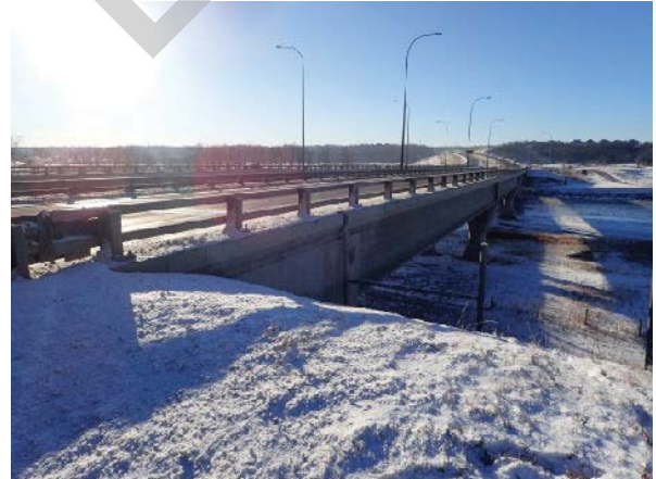
PHOTO 2 LEFT BANK, LOOKING DOWNSTREAM
