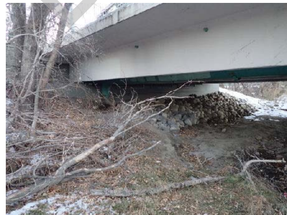
PHOTO 2 LEFT BANK, ABUTMENT
