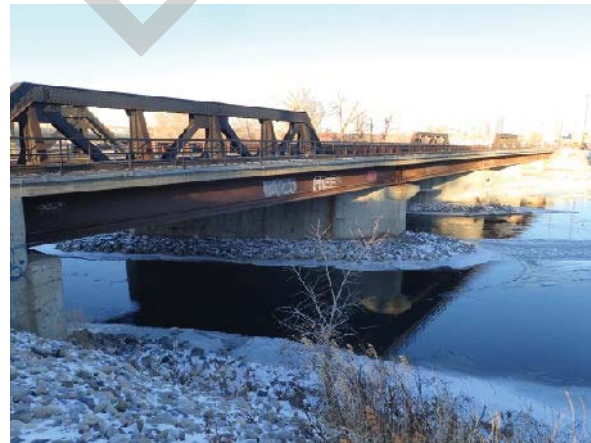
PHOTO 2 LEFT BANK, LOOKING DOWNSTREAM
