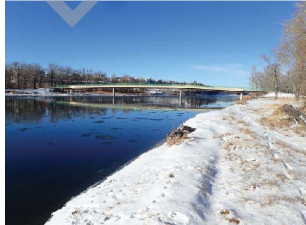
PHOTO 2 LEFT BANK, LOOKING UPSTREAM
