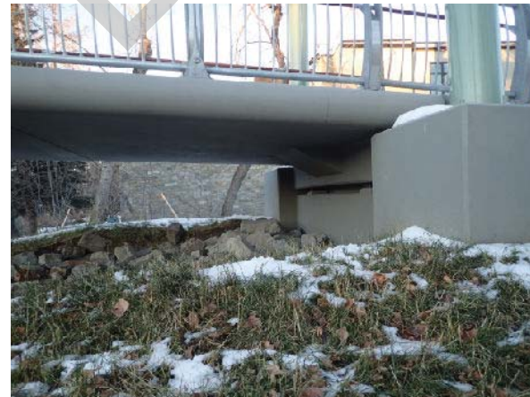
PHOTO 2 RIGHT BANK, ABUTMENT
