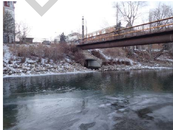
PHOTO 2 LEFT BANK, ABUTMENT
