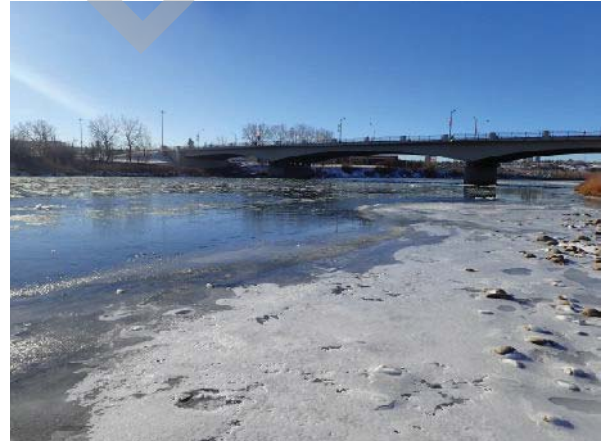
PHOTO 2 LEFT BANK, LOOKING UPSTREAM
