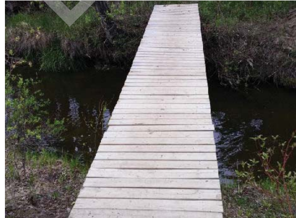
PHOTO 2 LOOKING ACROSS BRIDGE
