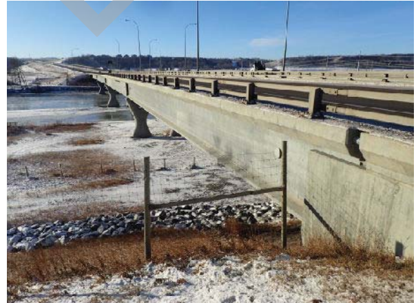
PHOTO 2 LEFT BANK, LOOKING UPSTREAM
