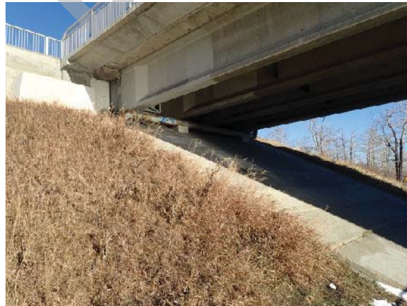
PHOTO 2 LEFT BANK, ABUTMENT
