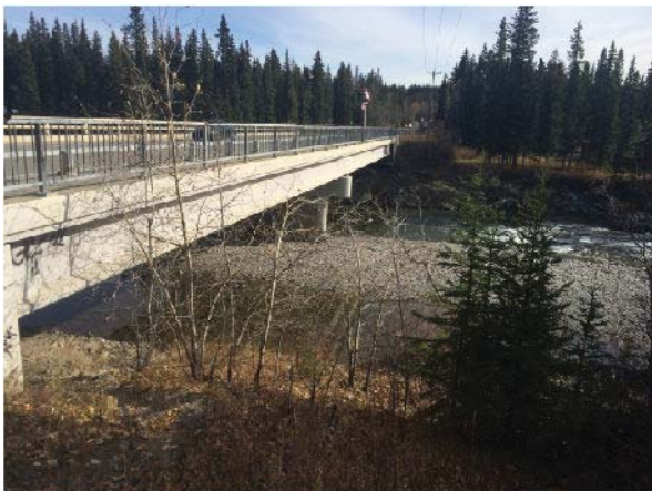
PHOTO 1 LEFT BANK, LOOKING DOWNSTREAM
