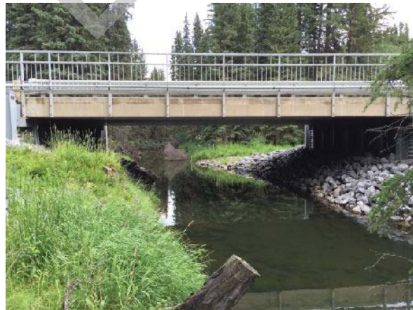
PHOTO 2 LEFT BANK, LOOKING DOWNSTREAM
