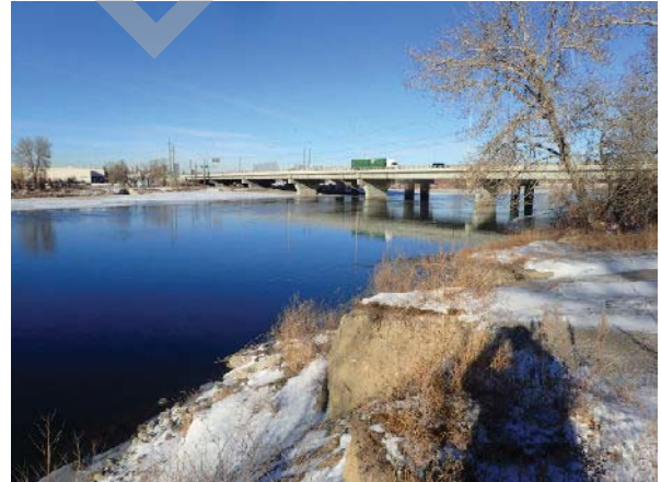
PHOTO 2 LEFT BANK, LOOKING UPSTREAM
