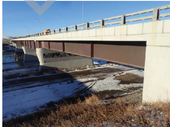
PHOTO 2 LEFT BANK, LOOKING UPSTREAM
