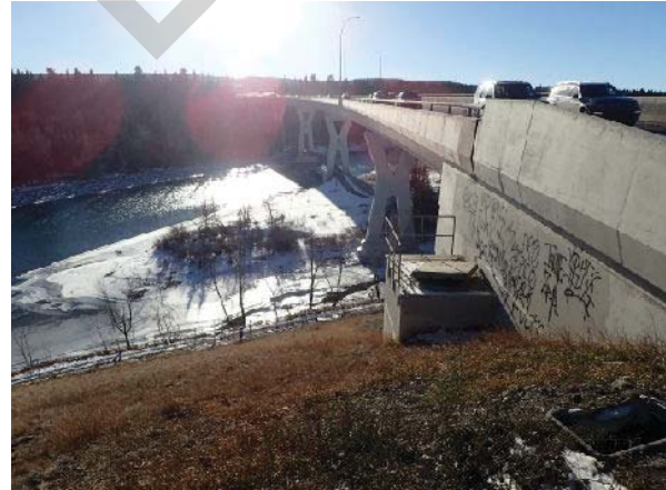
PHOTO 2 LEFT BANK, LOOKING UPSTREAM
