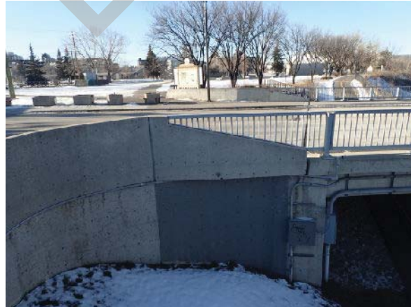
PHOTO 2 RIGHT BANK, ABUTMENT
