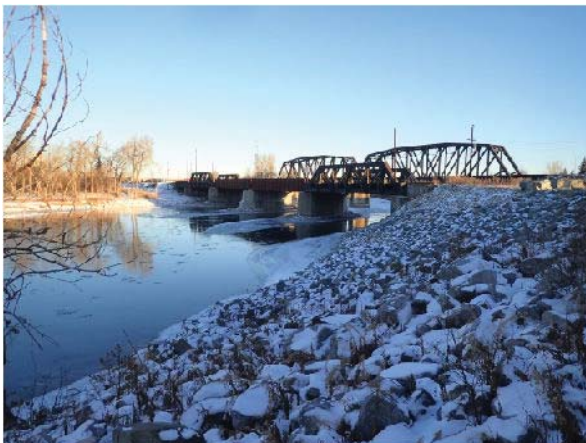
PHOTO 1 LEFT BANK, LOOKING UPSTREAM
