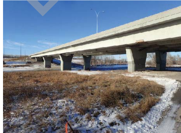
PHOTO 2 LEFT BANK, LOOKING UPSTREAM
