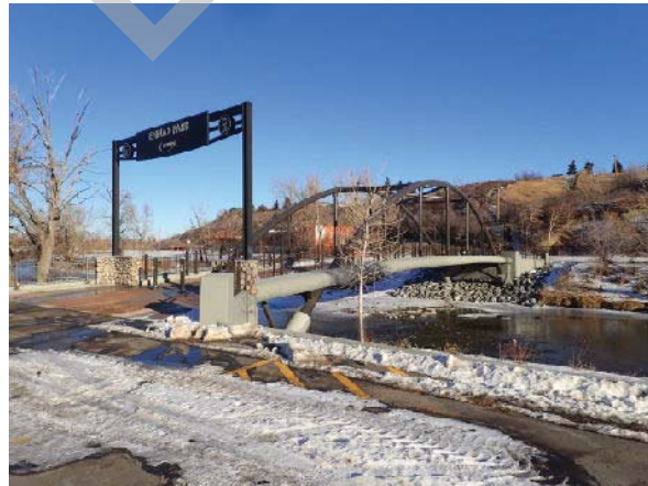
PHOTO 2 LEFT BANK, LOOKING DOWNSTREAM
