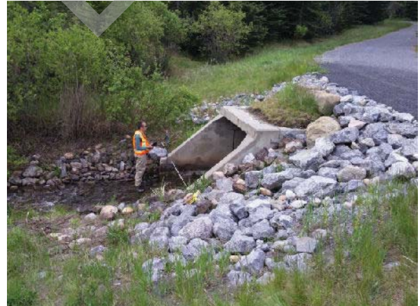
PHOTO 2 LEFT BANK, LOOKING UPSTREAM
