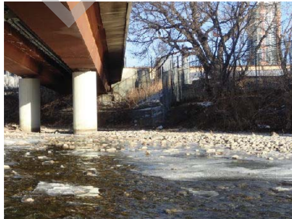
PHOTO 2 LEFT BANK, ABUTMENT
