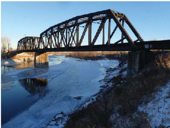
PHOTO 1 LEFT BANK, LOOKING UPSTREAM
