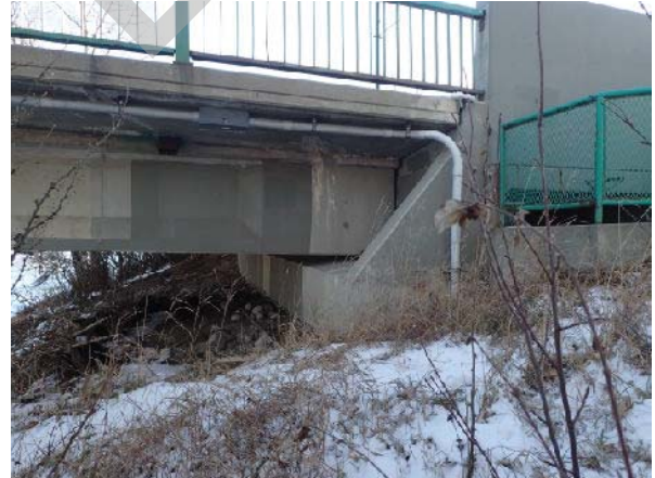
PHOTO 2 LEFT BANK, ABUTMENT
