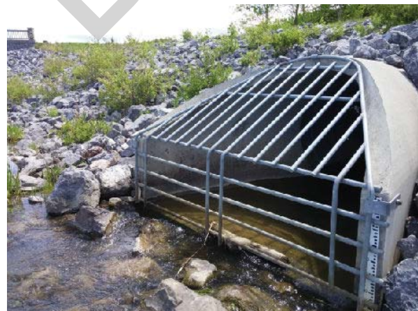
PHOTO 2 LEFT BANK, LOOKING UPSTREAM
