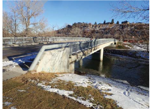
PHOTO 2 LEFT BANK, LOOKING DOWNSTREAM
