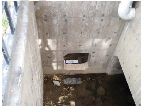
PHOTO 2 STRUCTURE INSIDE VIEW
