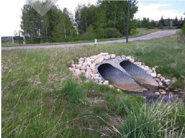
PHOTO 2 LEFT BANK, LOOKING DOWNSTREAM
