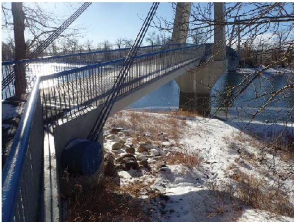
PHOTO 1 LEFT BANK, LOOKING DOWNSTREAM
