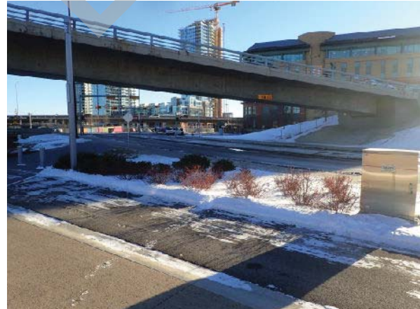
PHOTO 2 RIGHT BANK, ABUTMENT
