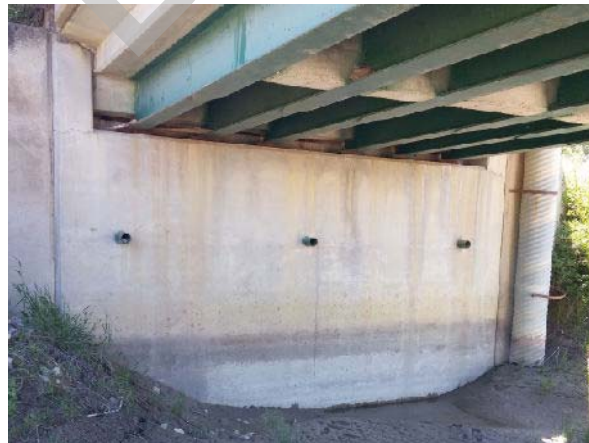
PHOTO 2 LEFT BANK, ABUTMENT
