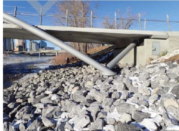
PHOTO 2 LEFT BANK, ABUTMENT
