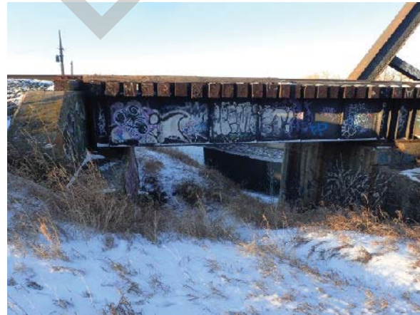
PHOTO 2 LEFT BANK, ABUTMENT
