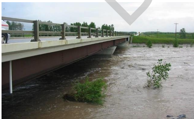
Photo 17: Highway 22 Bridge over the Elbow River on June 7, 2005 (Provided by RVC)
