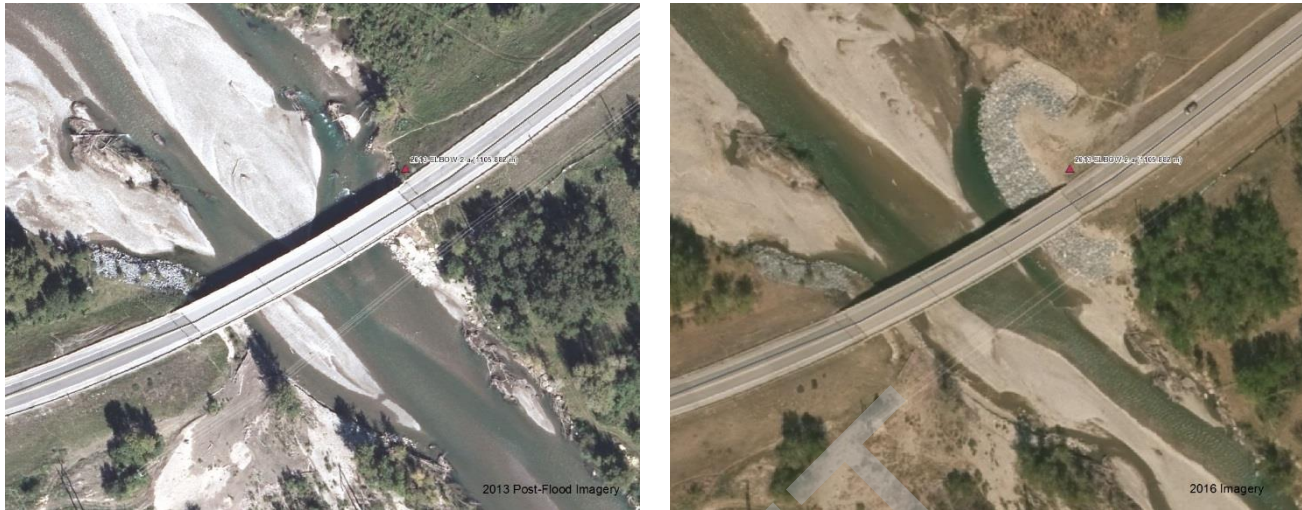
Figure 16: Highway 8 Bridge over the Elbow River after the 2013 Flood and in 2016
