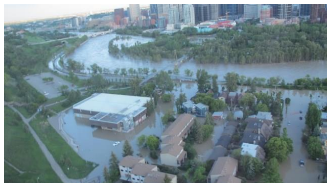
Photo 12: Flooding in Sunnyside on June 21, 2013 (Provided by the City of Calgary)
