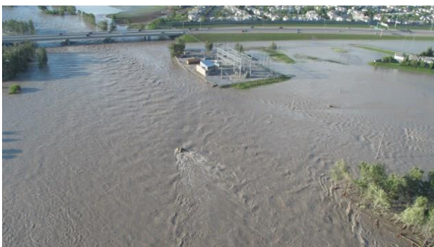
Photo 11: Enmax Substation 32 Downstream of Deerfoot Trail on June 21, 2013 (Provided by the City of Calgary)
