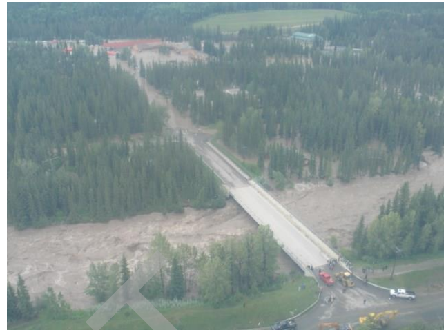
Photo 2: Balsam Avenue Bridge at Bragg Creek on June 20, 2013 (Provided by Rocky View County)
