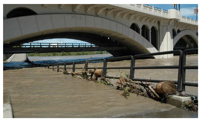
Photo 18: Centre Street Bridge in Calgary on June 8, 2005 (Provided by the City of Calgary)
