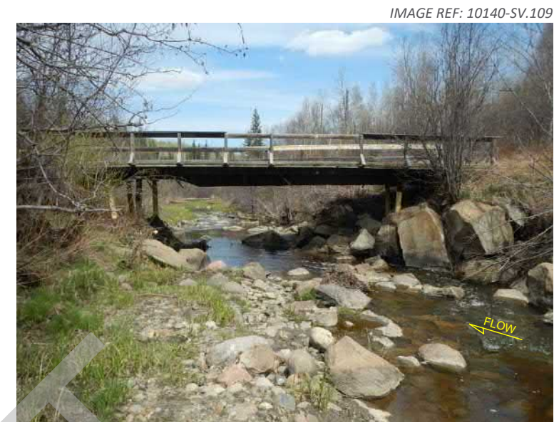
1. View looking downstream from the left bank.
