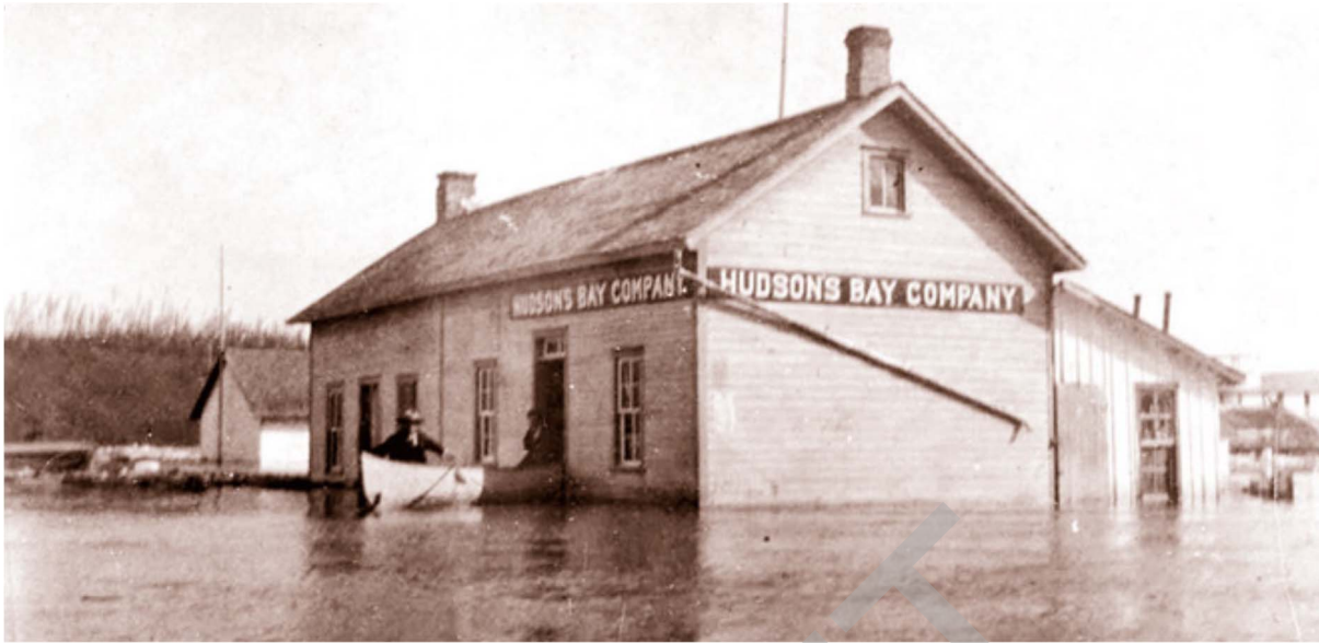
Figure I-5. HBC warehouse structure during 1904 ice jam flood. The location of this structure is unknown, but evidently it was dismantled after the flood. See Figure I-6 for its pre-flood condition.
