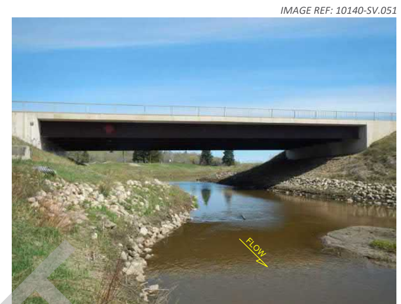
1. View looking downstream from the left bank.
