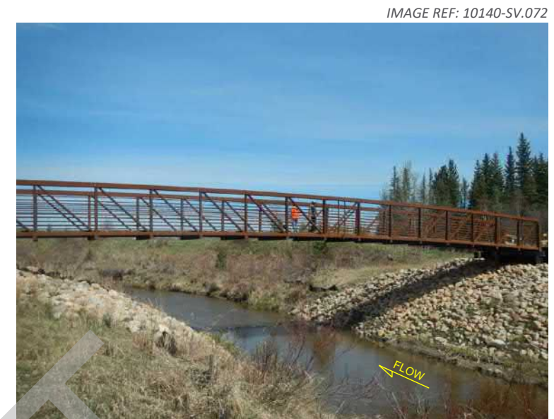
1. View looking downstream from the left bank.
