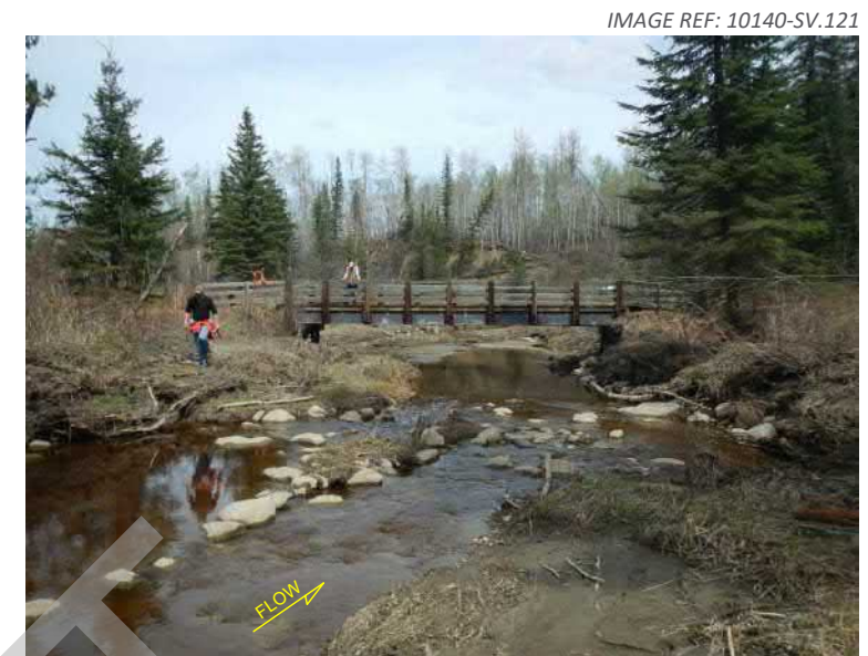
1. View looking downstream from the right bank.
