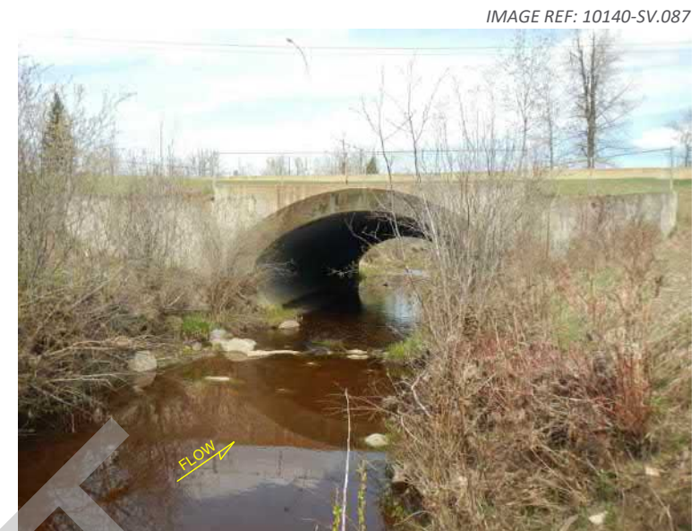
1. View looking downstream from the right bank.
