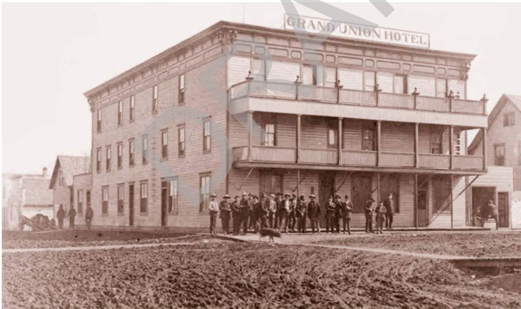
Figure I-12. The Grand Union Hotel before the fire of 1913. The original hotel was a two-storey structure. The third storey was added sometime prior to 1913. The front of the hotel is facing Strathcona Street.
