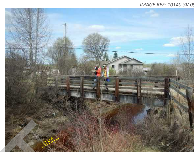
1. View looking downstream from the top of the right bank.
