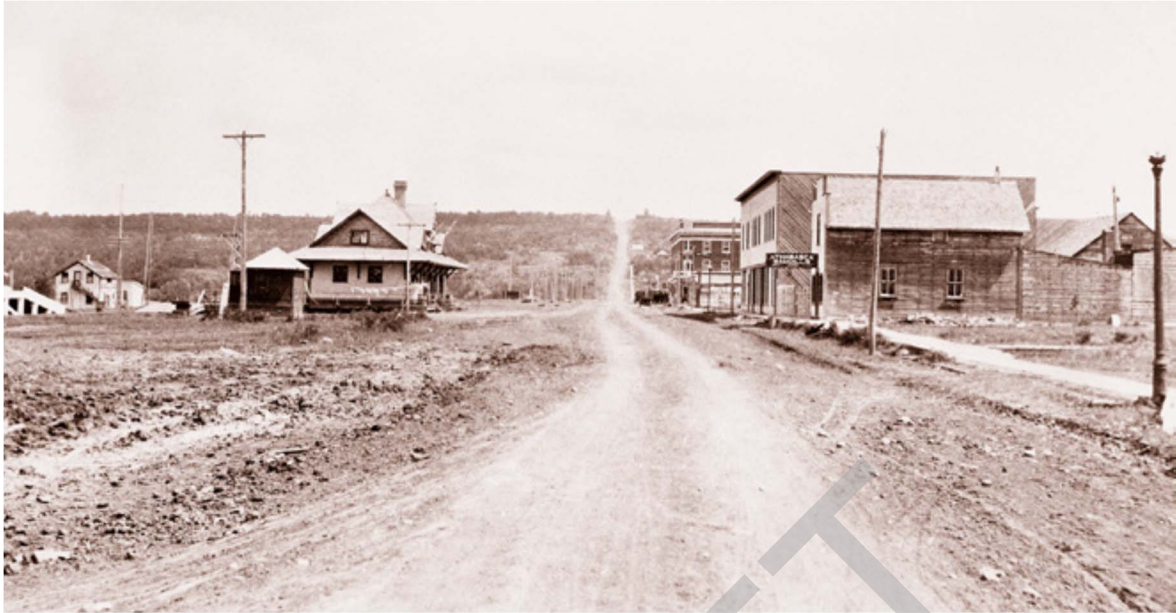
Figure I-11. Lichfield Street in the early 1920s, looking east with the NAR right-of-way on its left. The railway station is on the left, with the tracks located behind the station. The new post-fire Grand Union Hotel is in the background of the photo.
