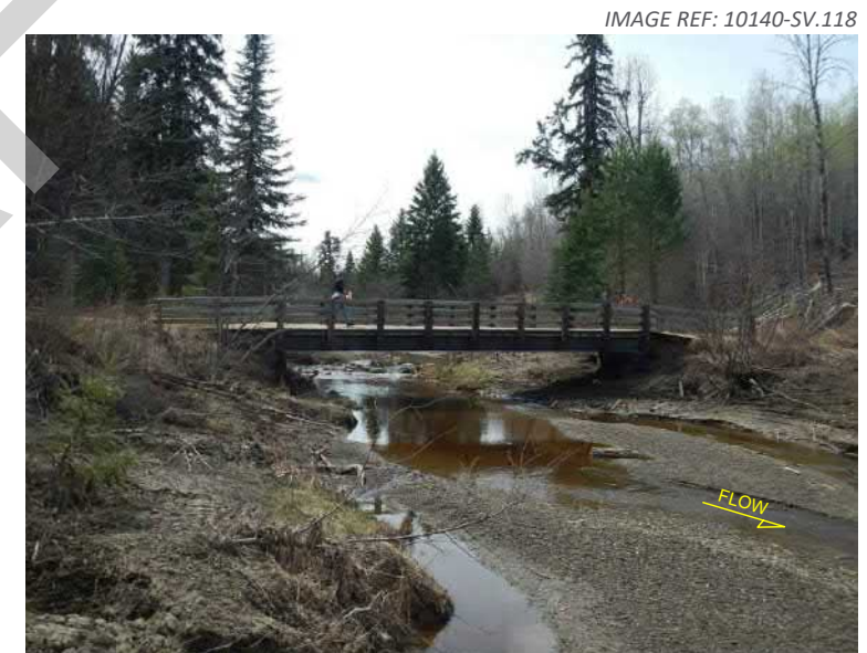
2. View looking upstream from the right bank.
