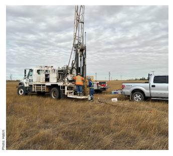
Standpipe Installation with protective steel casing riser and guards
