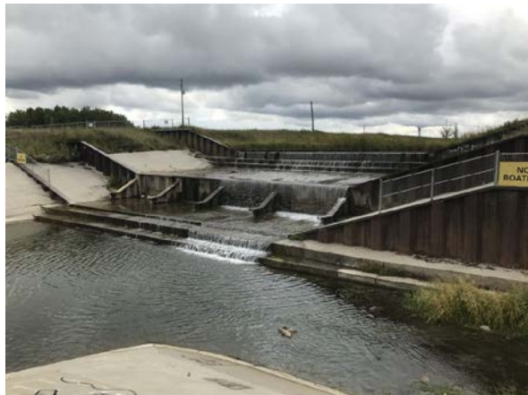
PHOTO 1 DOWNSTREAM LOOKING UPSTREAM
