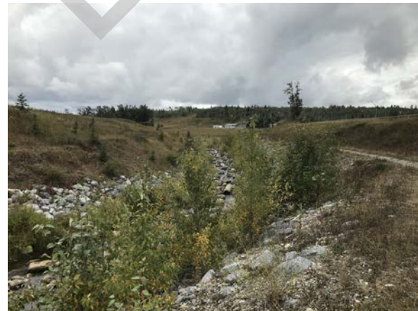
PHOTO 2 FISHWAY LOOKING UPSTREAM
