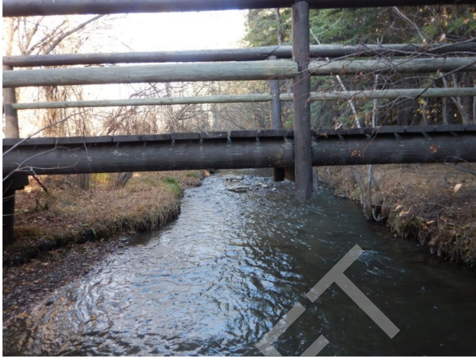
Bridge Photo 67. Bighill Creek, 4,360
