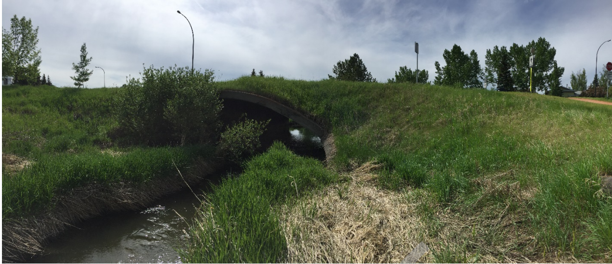
Culvert Photo 20. Bighill Creek, 2,498 (upstream)
