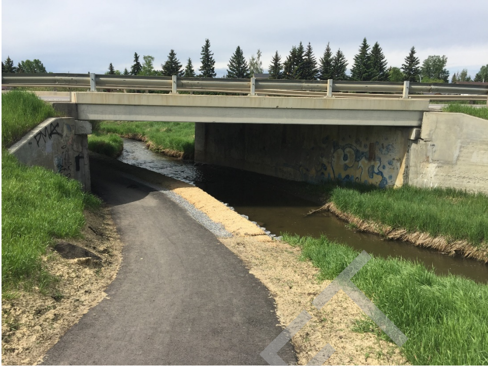
Bridge Photo 55. Bighill Creek, 2,814
