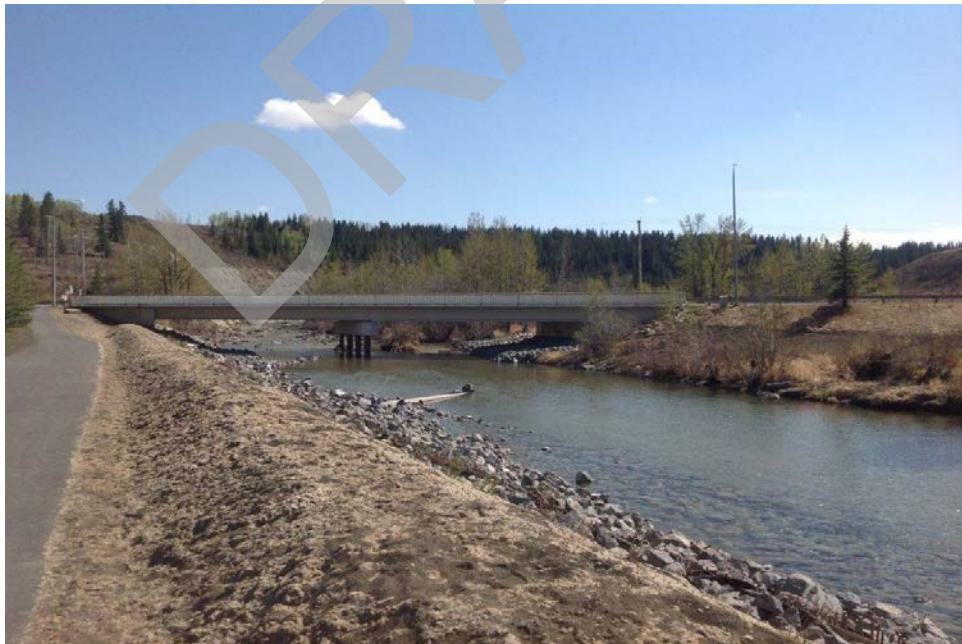
Bridge Photo 73. Jumpingpound Creek, 647
