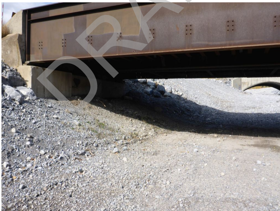
Bridge Photo 77. Exshaw Creek, 155
