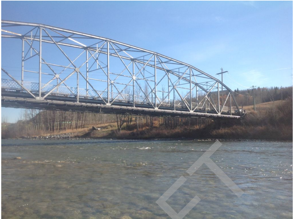
Bridge Photo 3. Bow River, 21,225
