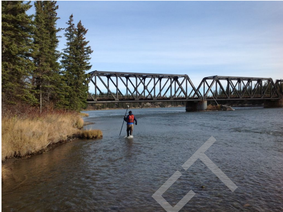
Bridge Photo 17. Bow River, 79,676
