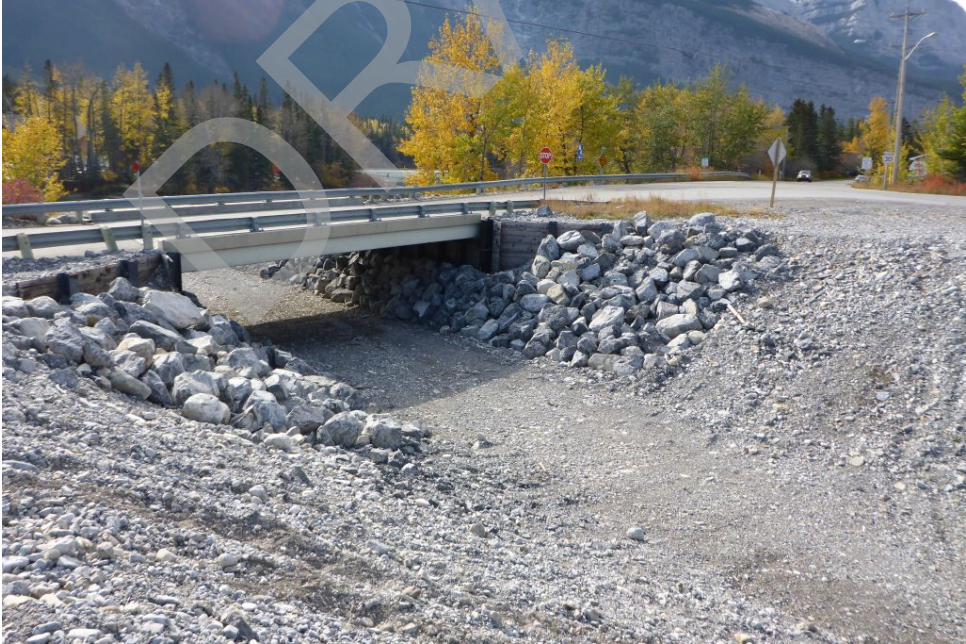
Bridge Photo 75. Exshaw Creek, 111
