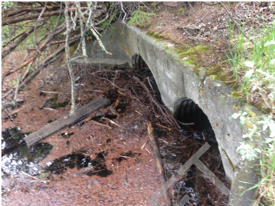
Culvert Photo 31. Side channel of Policeman Creek, 4,256
