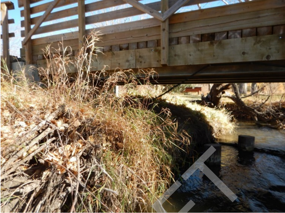
Bridge Photo 59. Bighill Creek, 3,385
