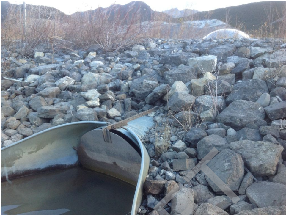
Culvert Photo 5. Bow River, 88,420
