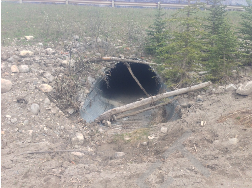
Culvert Photo 13. Side channel of Bow River, 105,880
