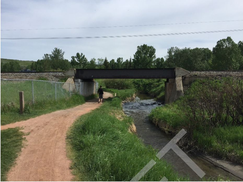
Bridge Photo 51. Bighill Creek, 2,754
