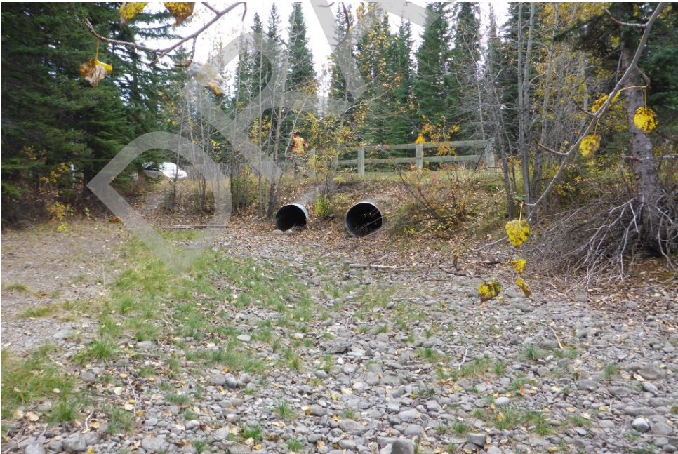
Culvert Photo 26. Policeman Creek, 5,003
