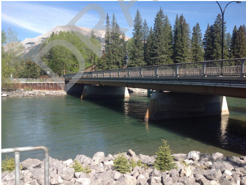
Bridge Photo 22. Bow River, 109,223
