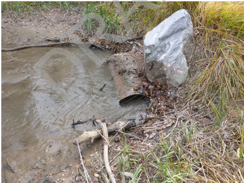
Culvert Photo 28. Policeman Creek, 6,435
