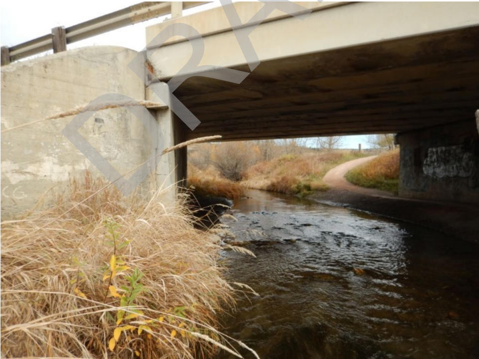
Bridge Photo 56. Bighill Creek, 2,814
