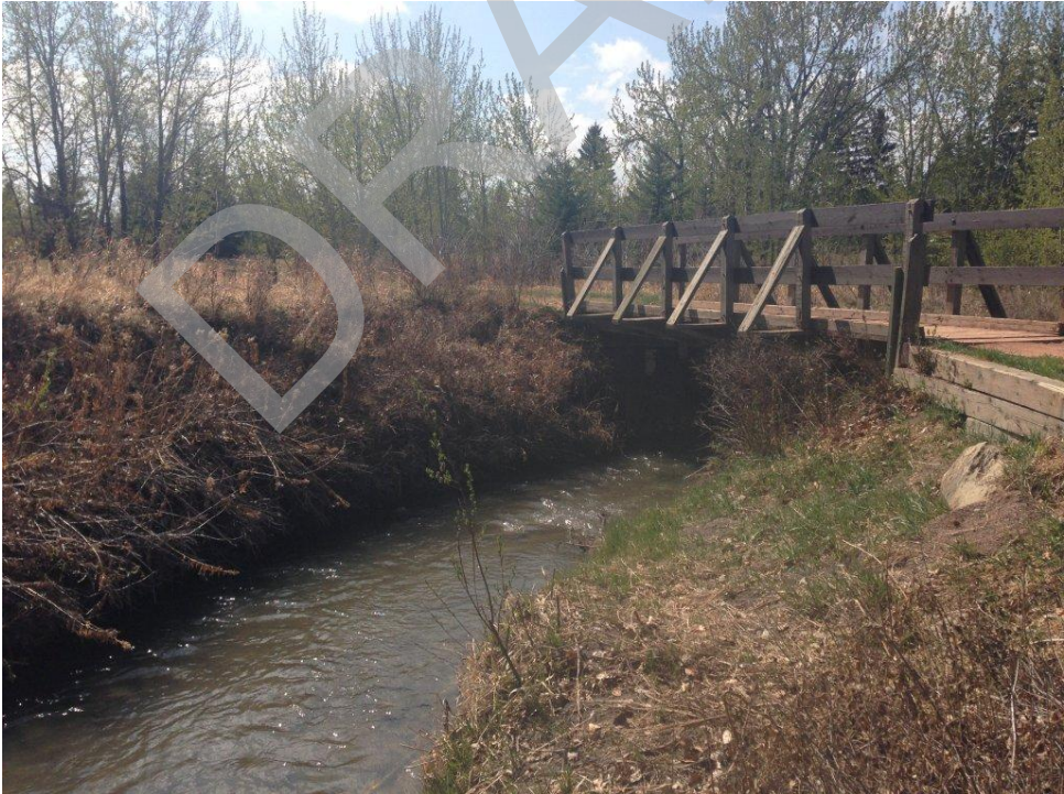
Bridge Photo 48. Bighill Creek, 1,812
