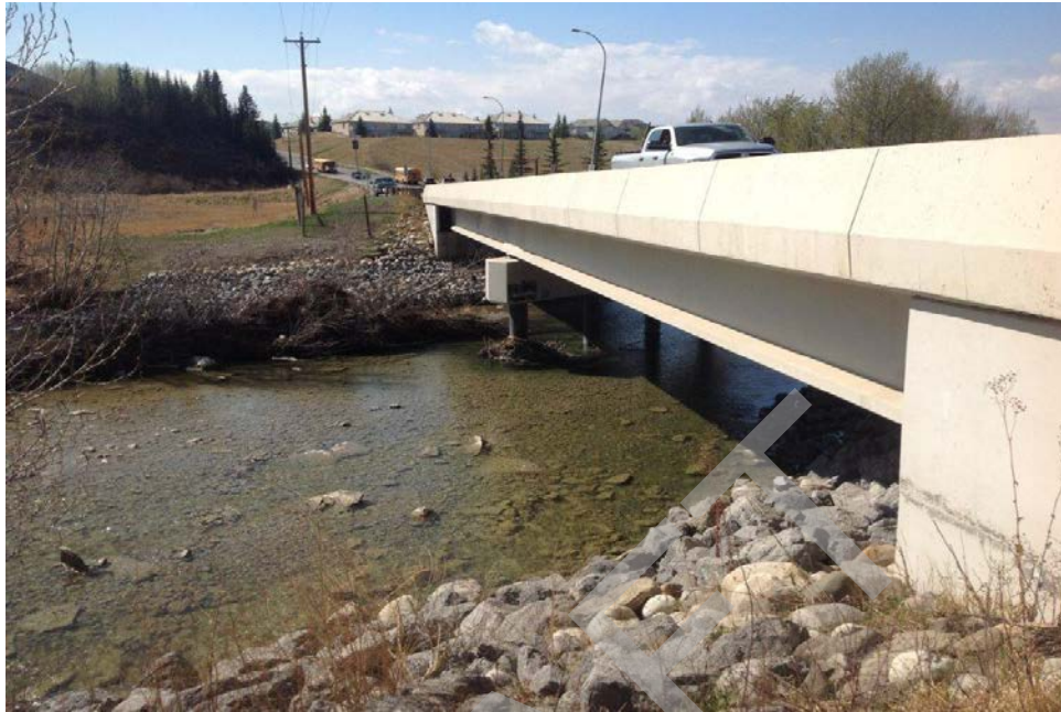
Bridge Photo 72. Jumpingpound Creek, 647
