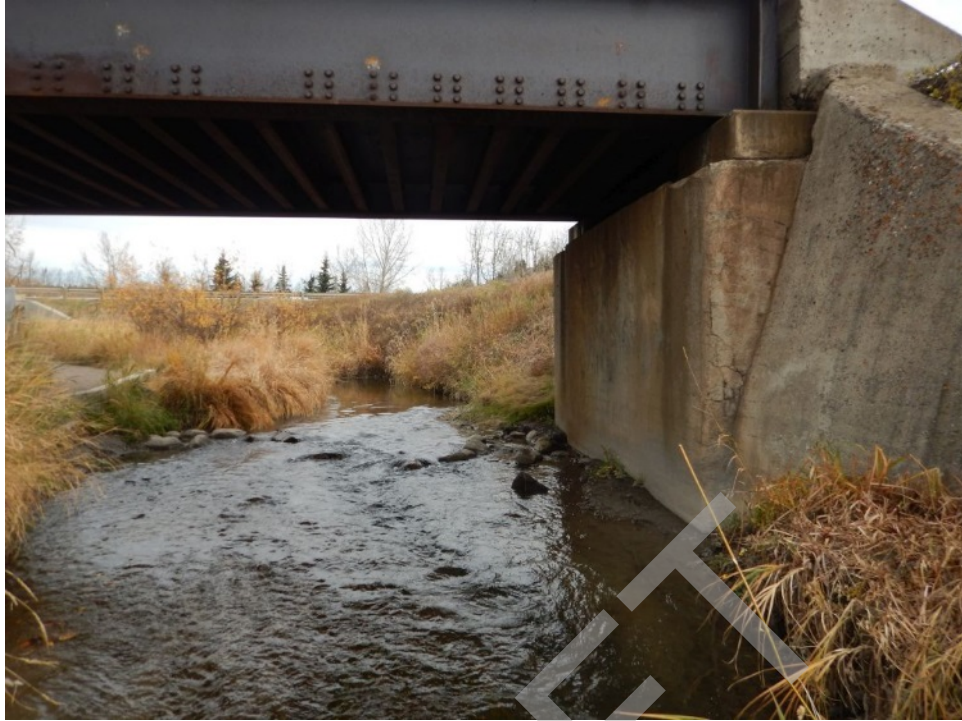
Bridge Photo 53. Bighill Creek, 2,754
