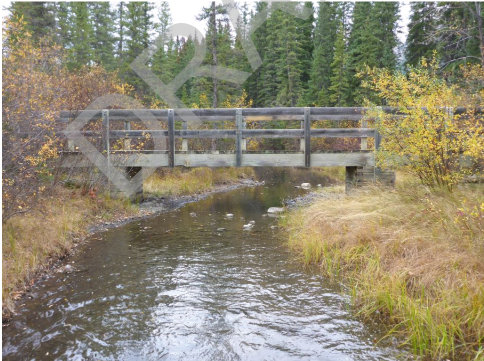
Bridge Photo 90. Policeman Creek, 4,717
