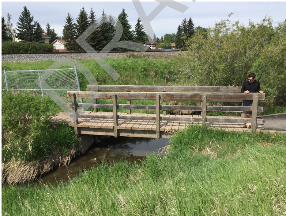
Bridge Photo 54. Bighill Creek, 2,786
