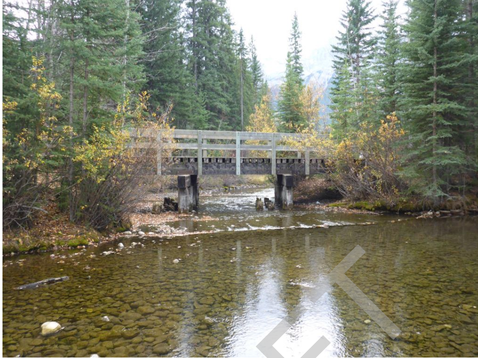
Bridge Photo 87. Policeman Creek, 4,328
