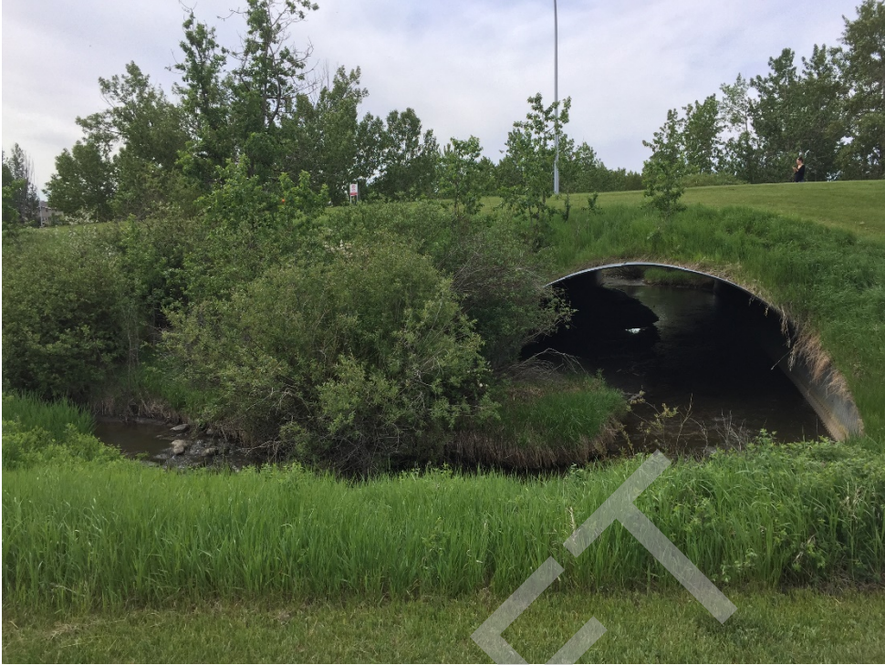
Culvert Photo 18. Bighill Creek, 1,519 (upstream)
