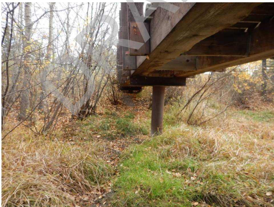
Bridge Photo 42. Bighill Creek, 992
