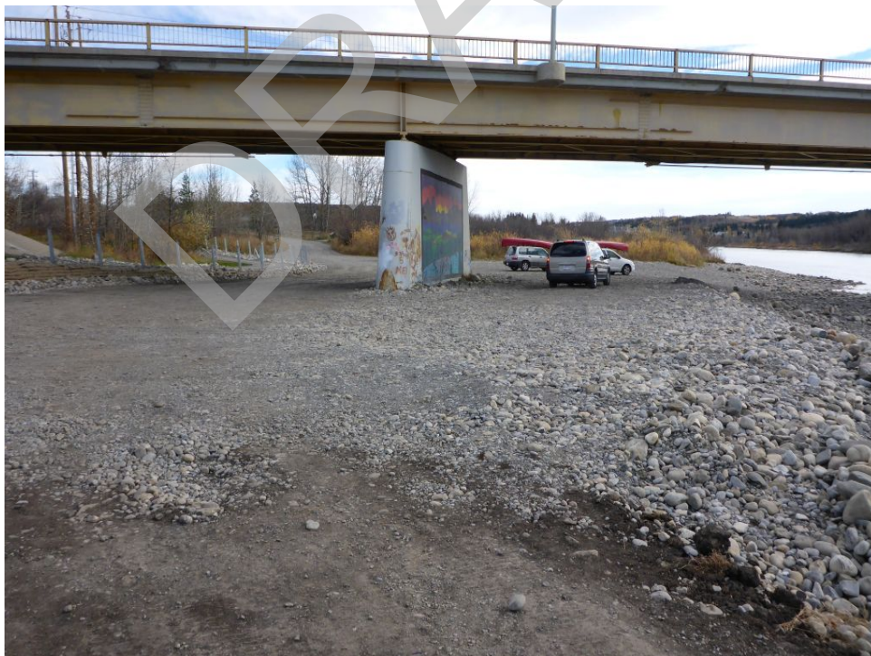
Bridge Photo 6. Bow River, 23,403
