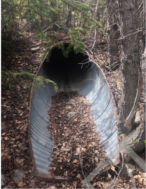
Culvert Photo 11. Side channel of Bow River, 105,661
