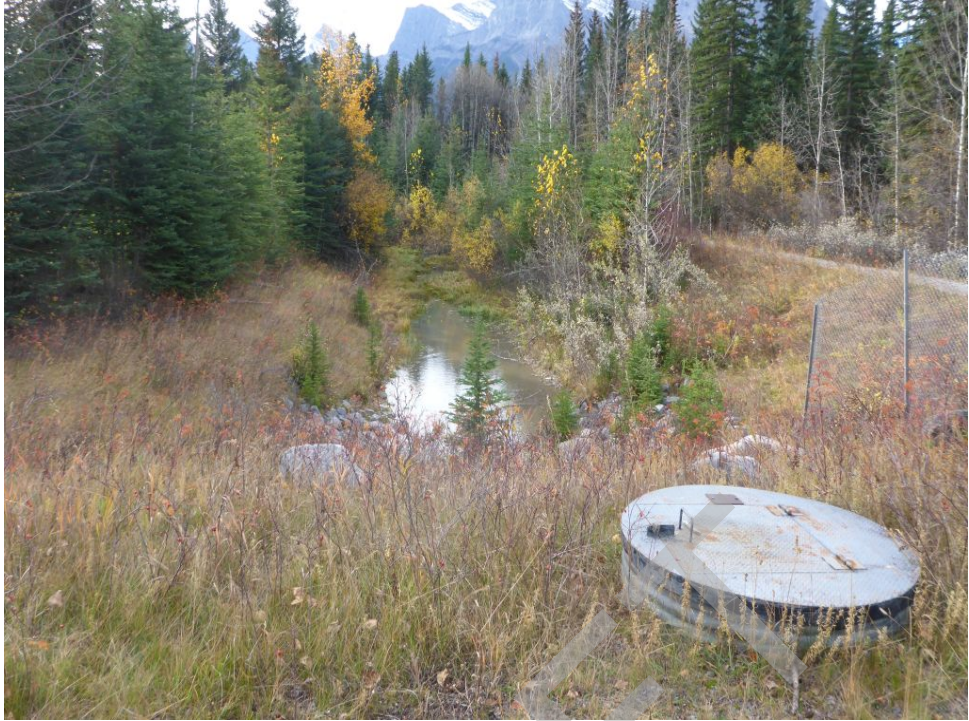
Culvert Photo 29. Policeman Creek, 6,435
