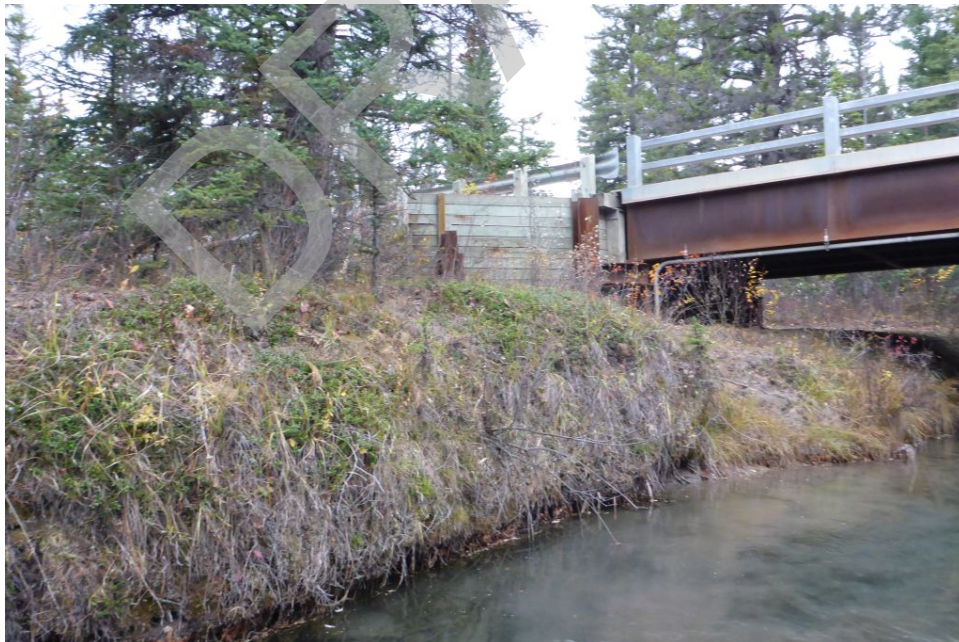
Bridge Photo 80. Policeman Creek, 1,552
