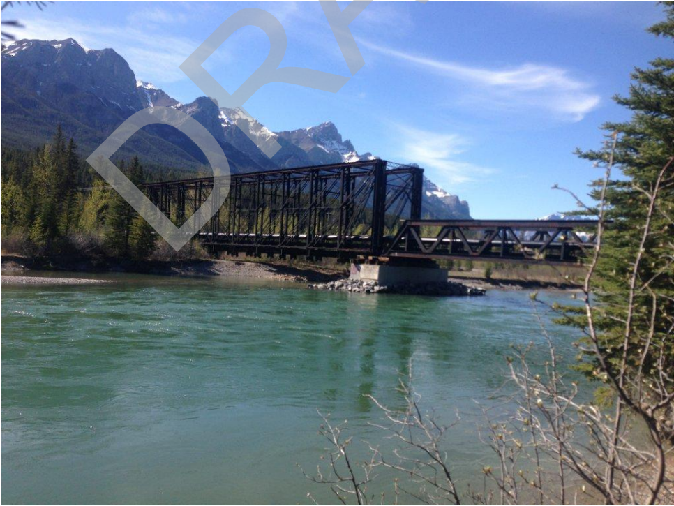
Bridge Photo 24. Bow River, 109,929
