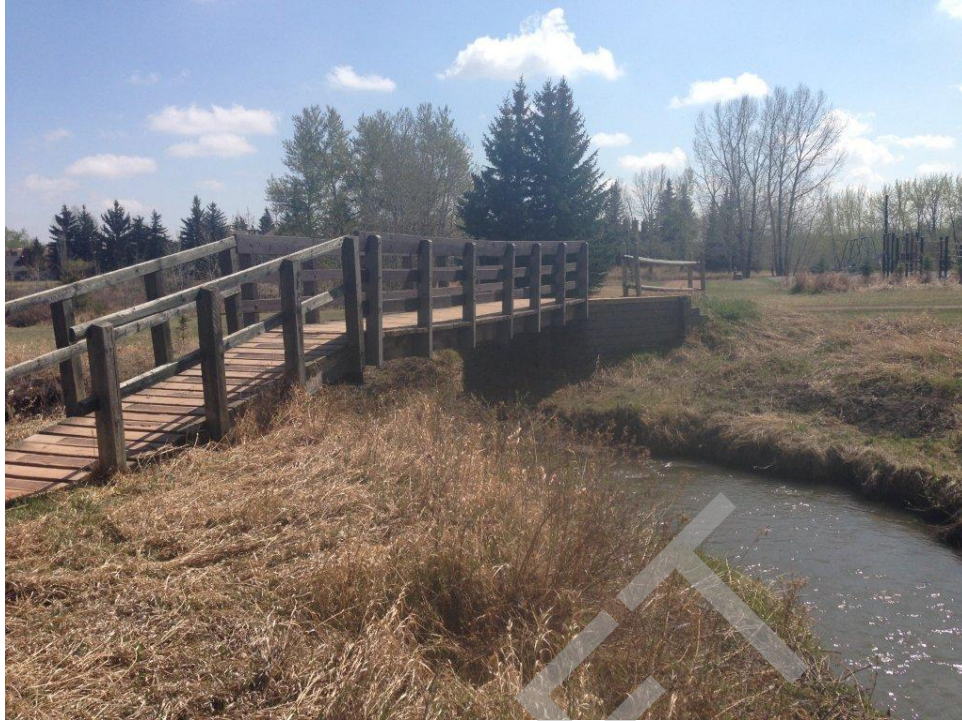
Bridge Photo 49. Bighill Creek, 2,158
