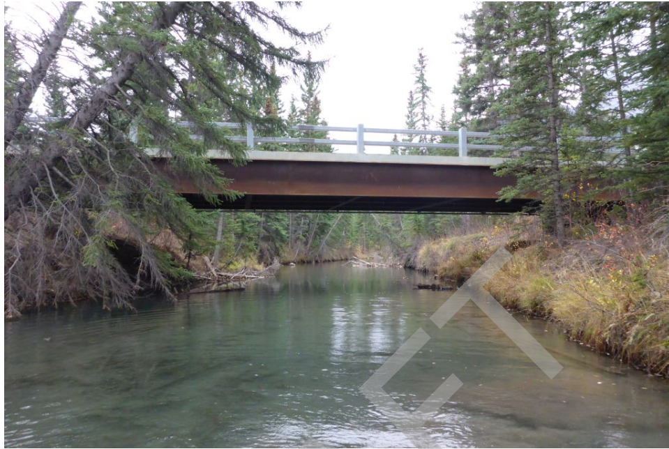
Bridge Photo 79. Policeman Creek, 1,552
