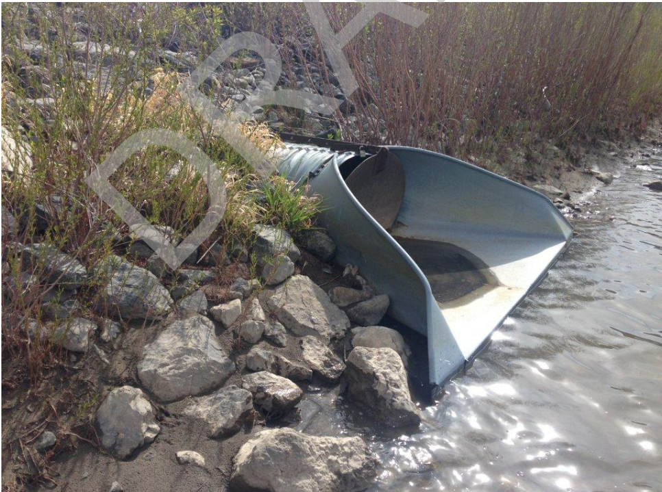
Culvert Photo 4. Bow River, 88,251
