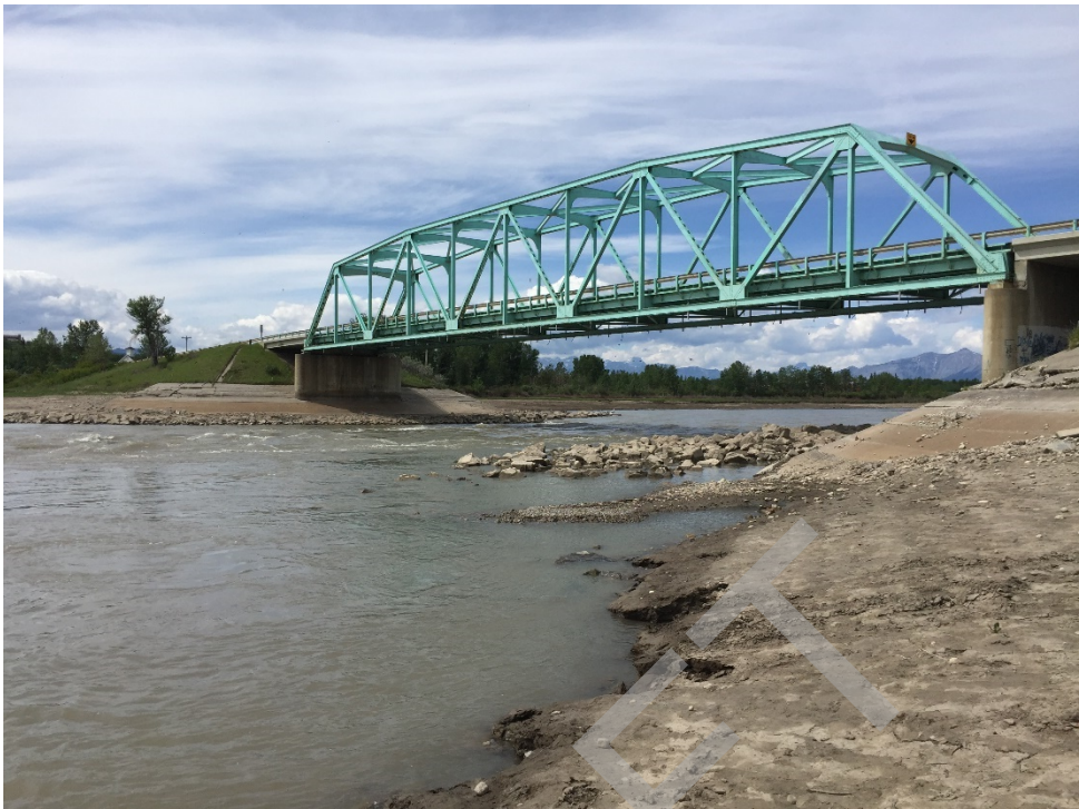
Bridge Photo 11. Bow River, 54,457
