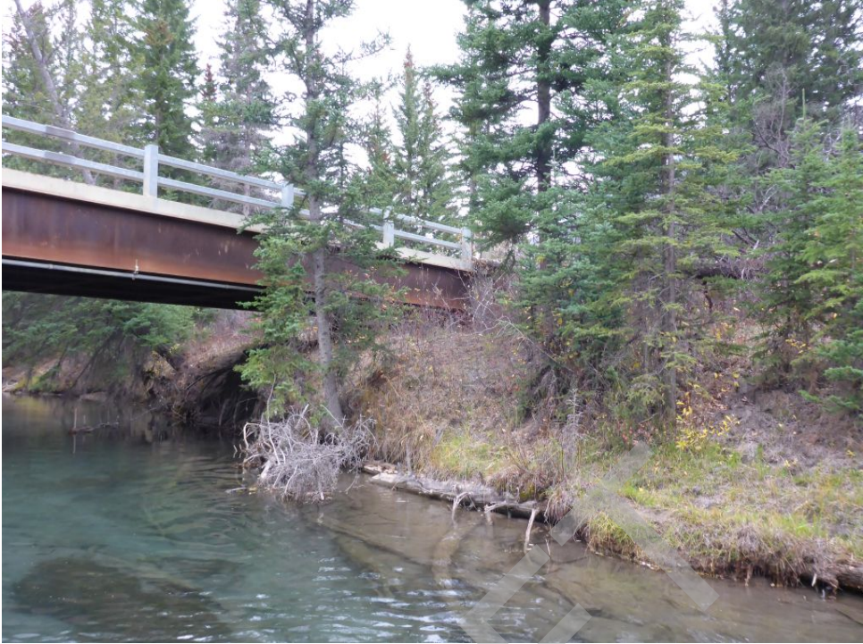
Bridge Photo 81. Policeman Creek, 1,552
