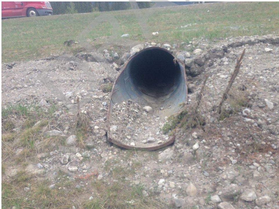
Culvert Photo 10. Side channel of Bow River, 105,661
