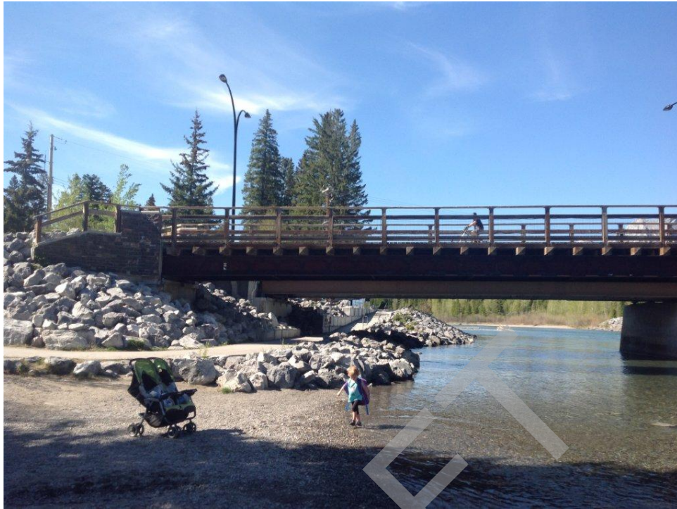
Bridge Photo 21. Bow River, 109,212
