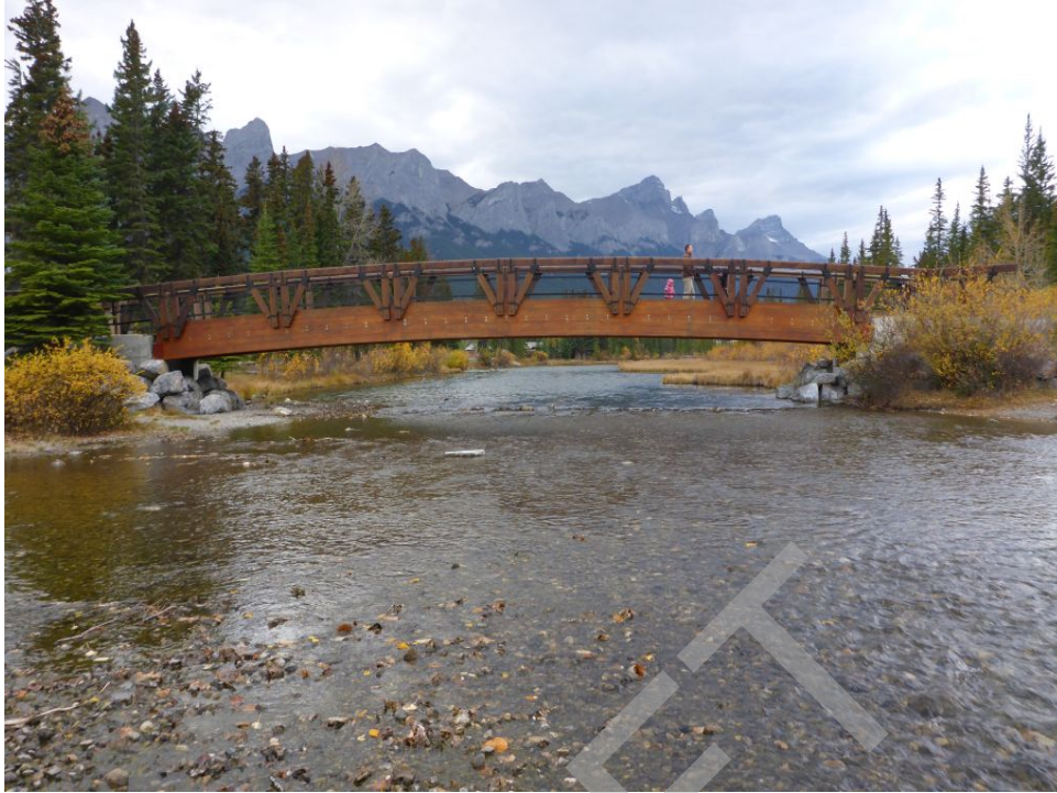
Bridge Photo 83. Policeman Creek, 3,147
