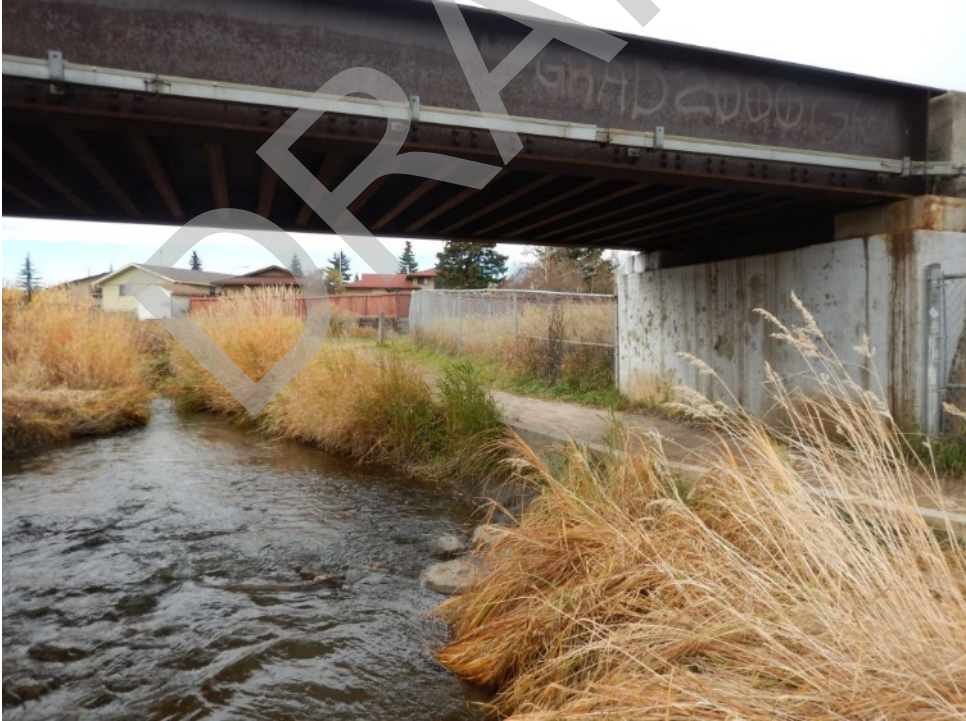
Bridge Photo 52. Bighill Creek, 2,754
