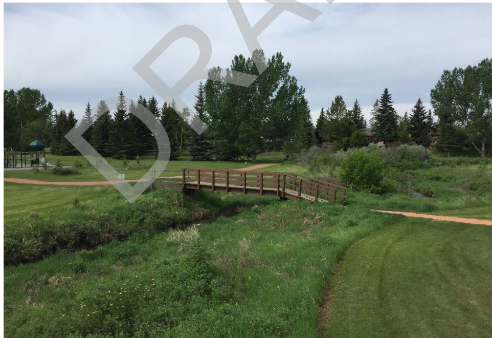
Bridge Photo 50. Bighill Creek, 2,158
