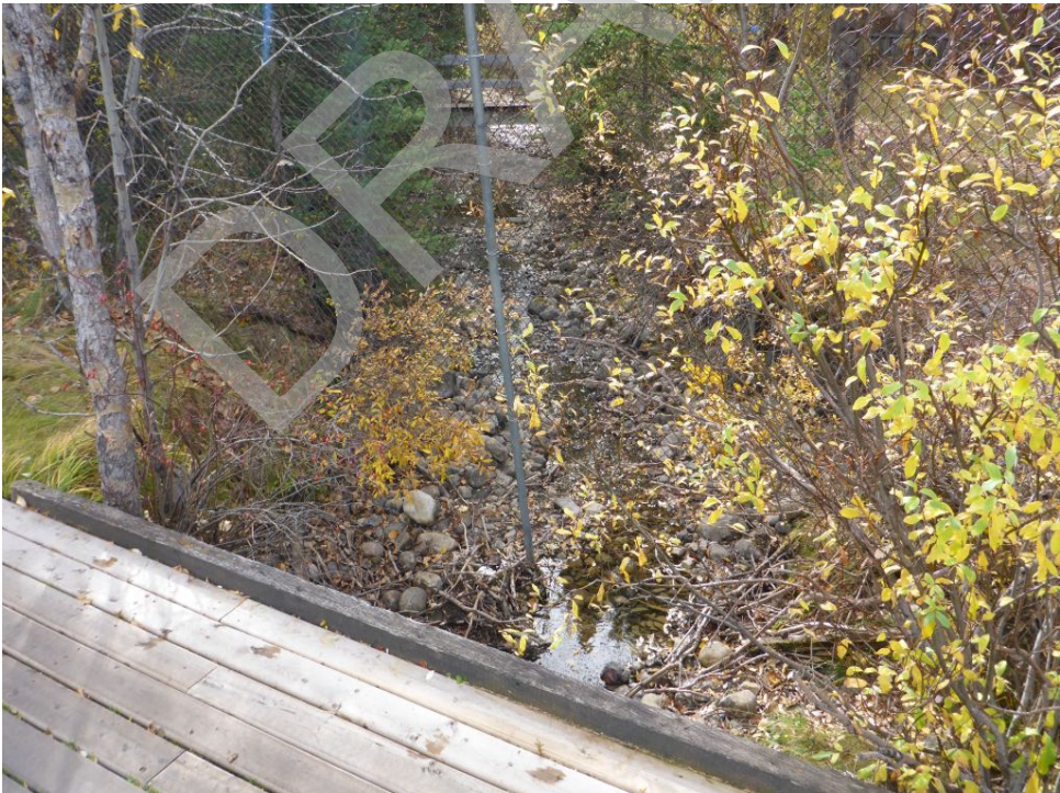
Bridge Photo 102. Policeman Creek, 5,668
