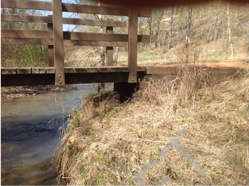
Bridge Photo 35. Bighill Creek, 372
