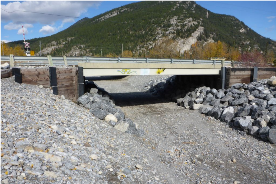
Bridge Photo 74. Exshaw Creek, 111
