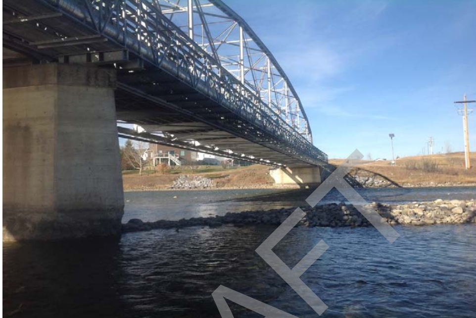
Bridge Photo 1. Bow River, 21,225
