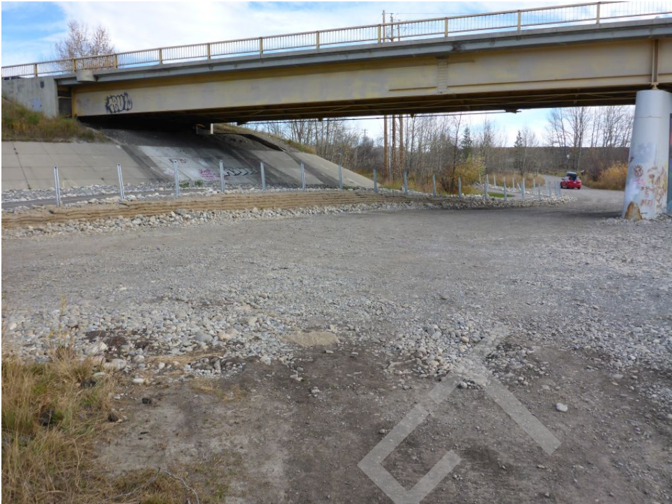
Bridge Photo 7. Bow River, 23,403
