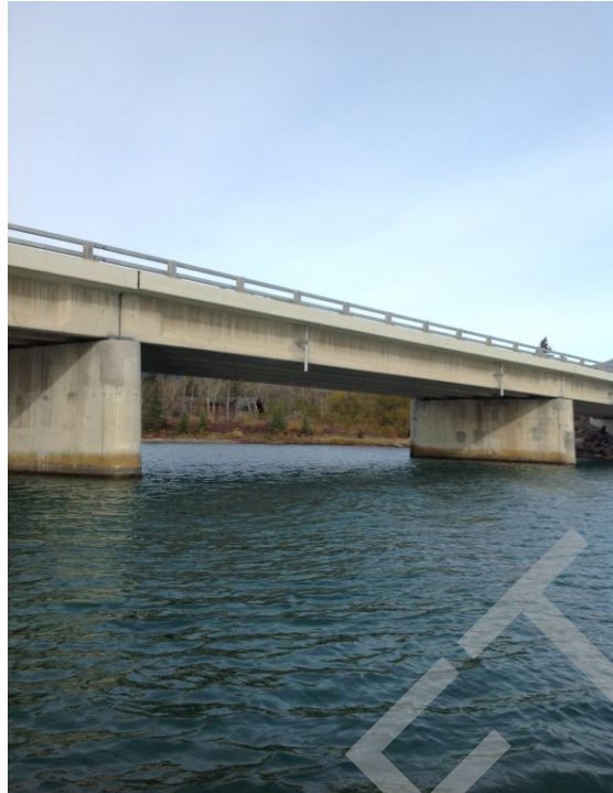
Bridge Photo 13. Bow River, 77,639
