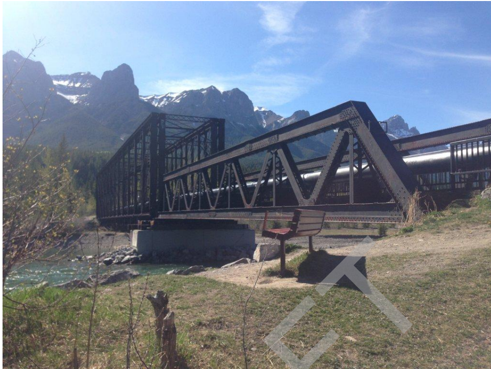
Bridge Photo 25. Bow River, 109,929
