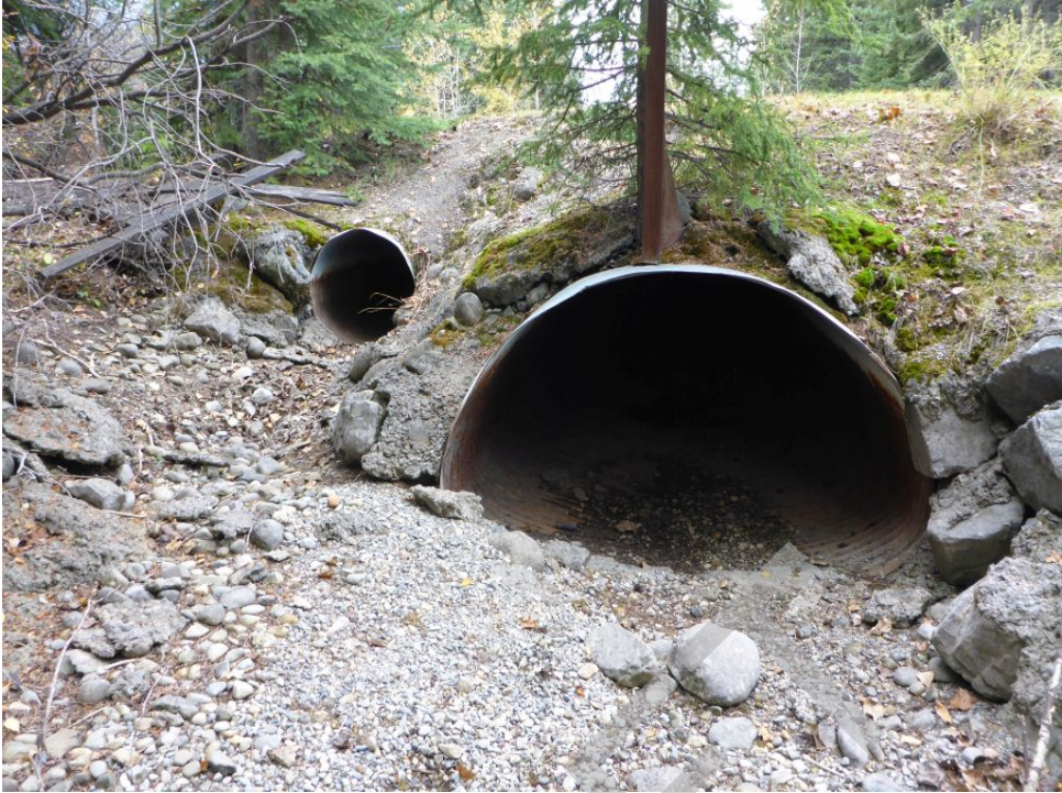
Culvert Photo 25. Policeman Creek, 5,003
