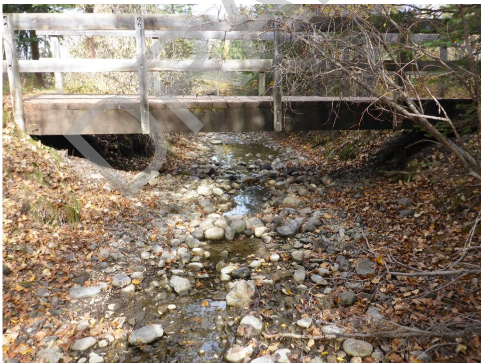
Bridge Photo 100. Policeman Creek, 5,648
