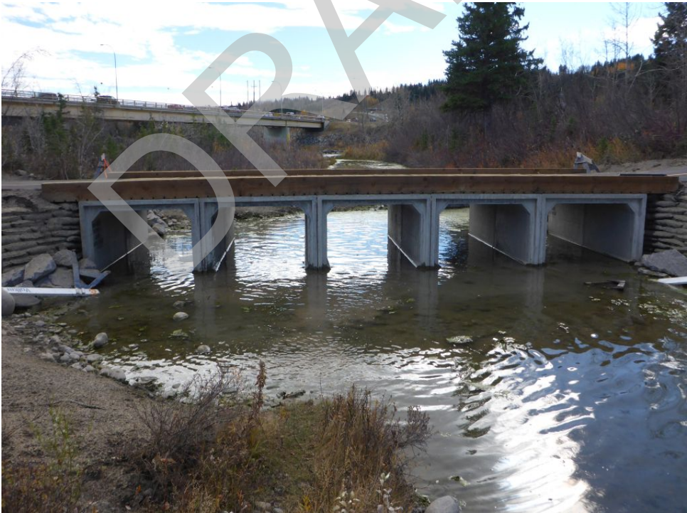
Culvert Photo 8. Side channel of Bow River, 23,505
