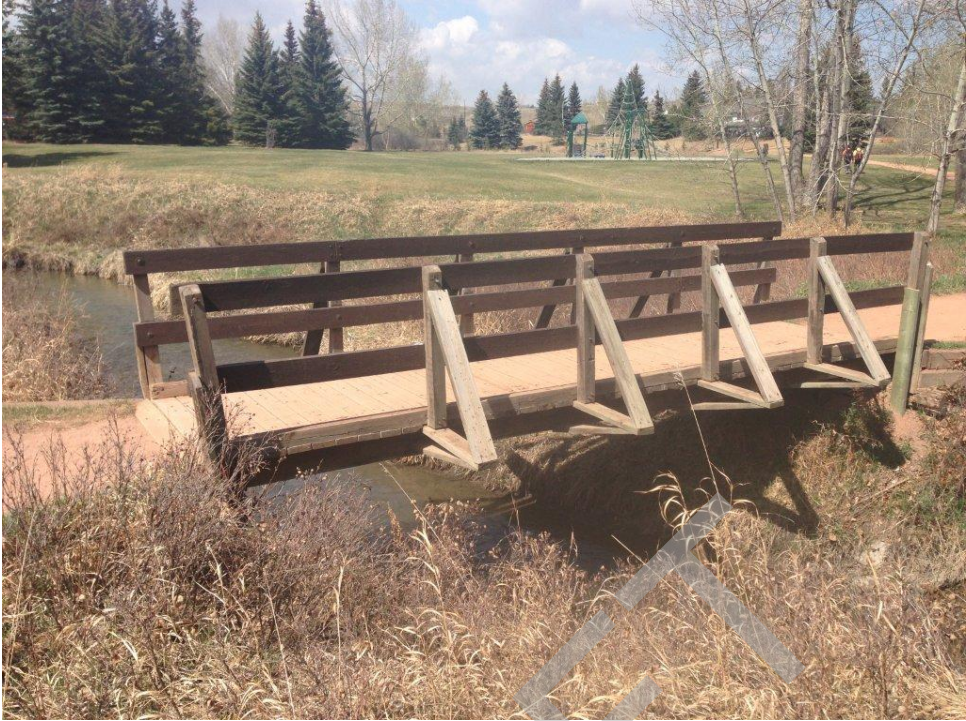
Bridge Photo 47. Bighill Creek, 1,812
