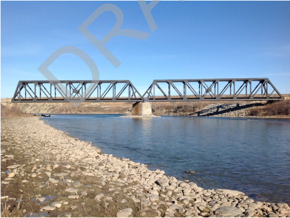
Bridge Photo 8. Bow River, 27,374
