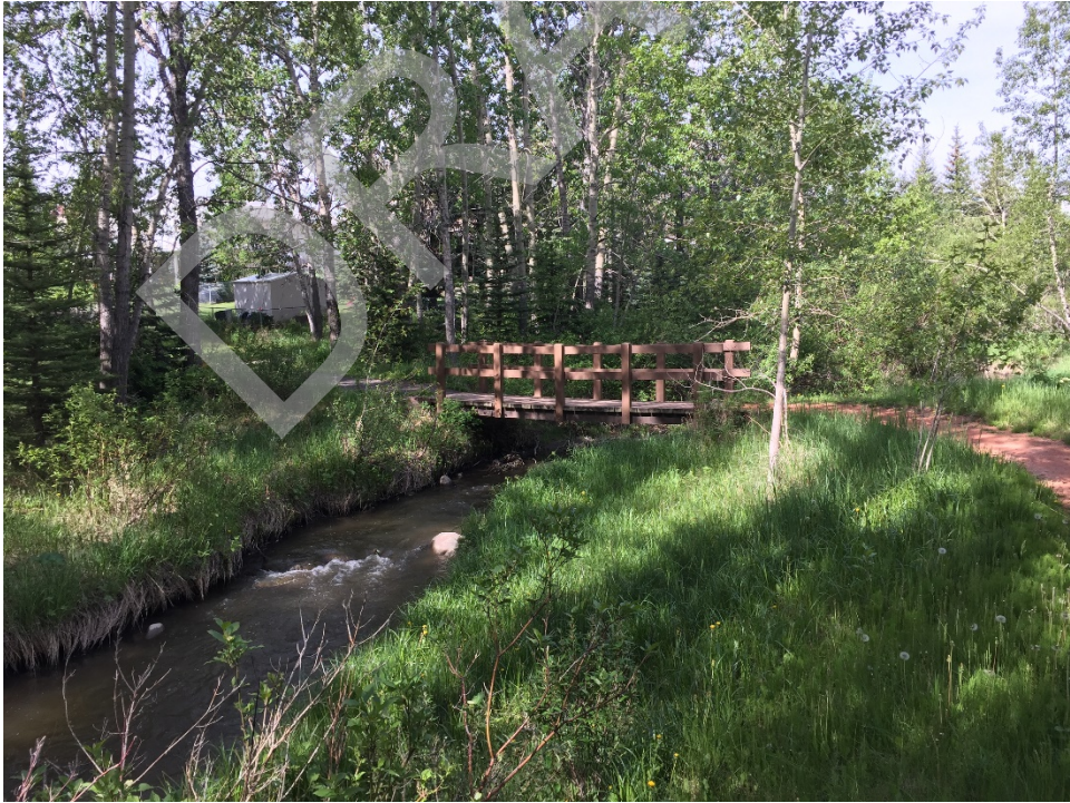
Bridge Photo 36. Bighill Creek, 372
