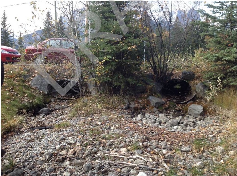
Culvert Photo 30. Side channel of Policeman Creek, 4,159
