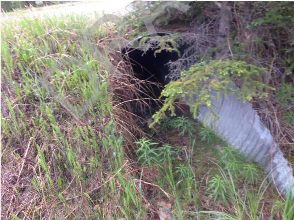
Culvert Photo 34. Side channel of Policeman Creek, 4,877
