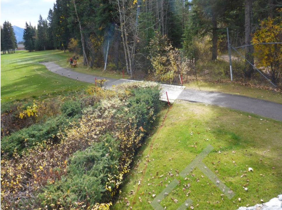
Bridge Photo 101. Policeman Creek, 5,668
