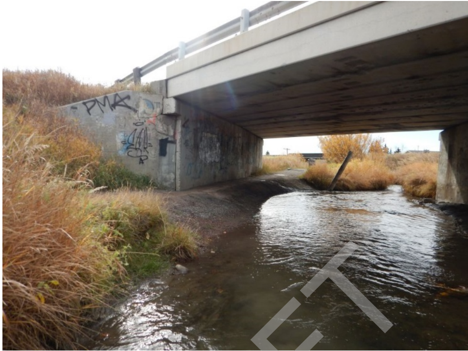
Bridge Photo 57. Bighill Creek, 2,814
