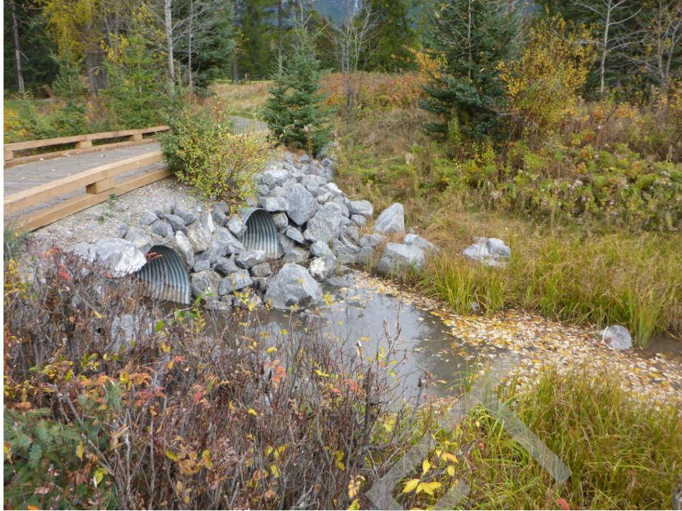
Culvert Photo 27. Policeman Creek, 5,957
