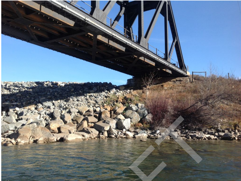
Bridge Photo 9. Bow River, 27,374
