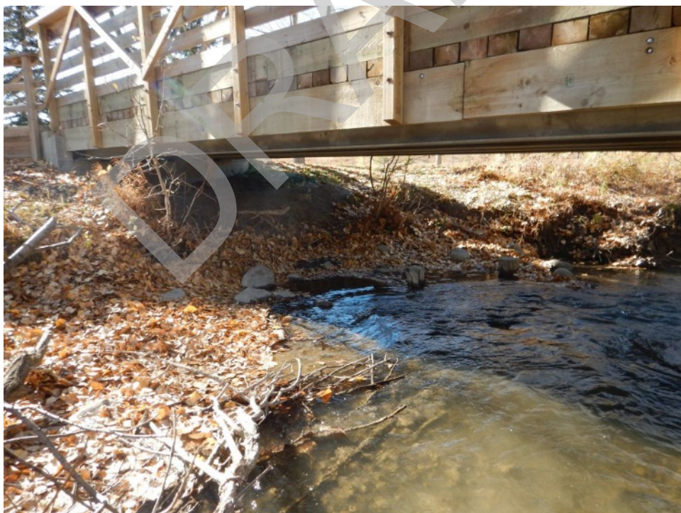
Bridge Photo 62. Bighill Creek, 3,385
