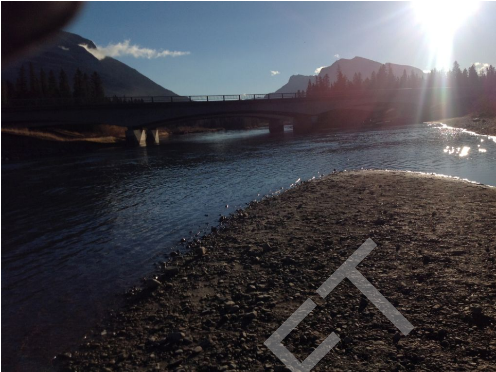
Bridge Photo 19. Bow River, 104,509 and 104,549 (upstream)
