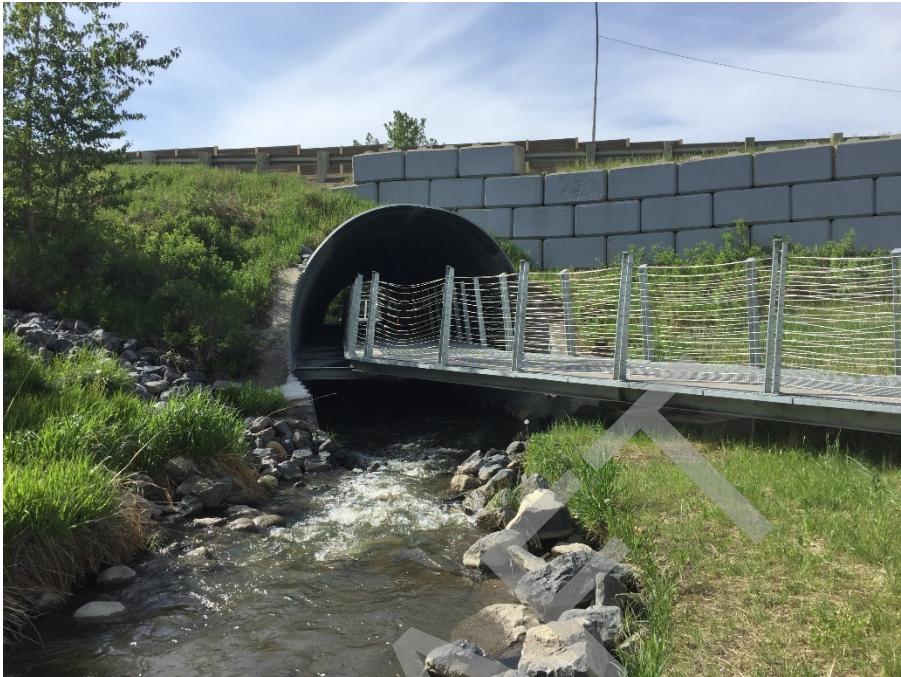
Culvert Photo 14. Bighill Creek, 480 (upstream)
