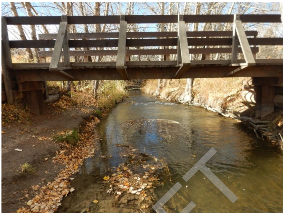
Bridge Photo 45. Bighill Creek, 1,722
