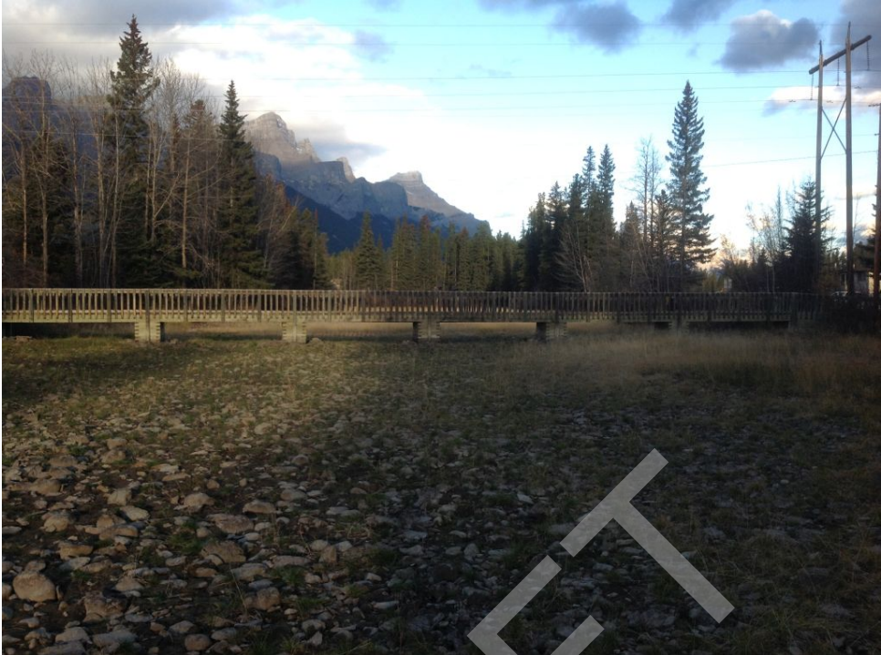
Bridge Photo 105. Side channel of Policeman Creek, 5,331
