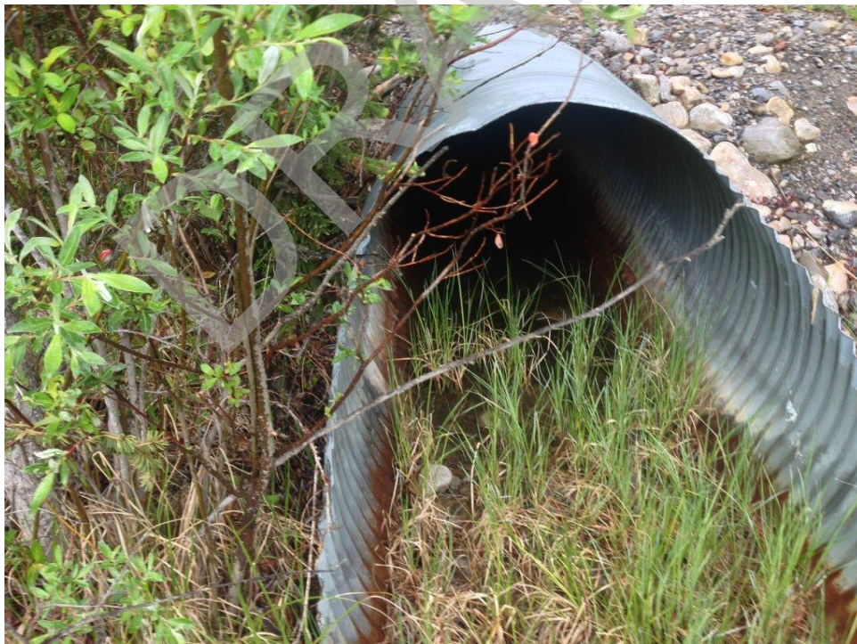
Culvert Photo 36. Side channel of Policeman Creek, 4,877
