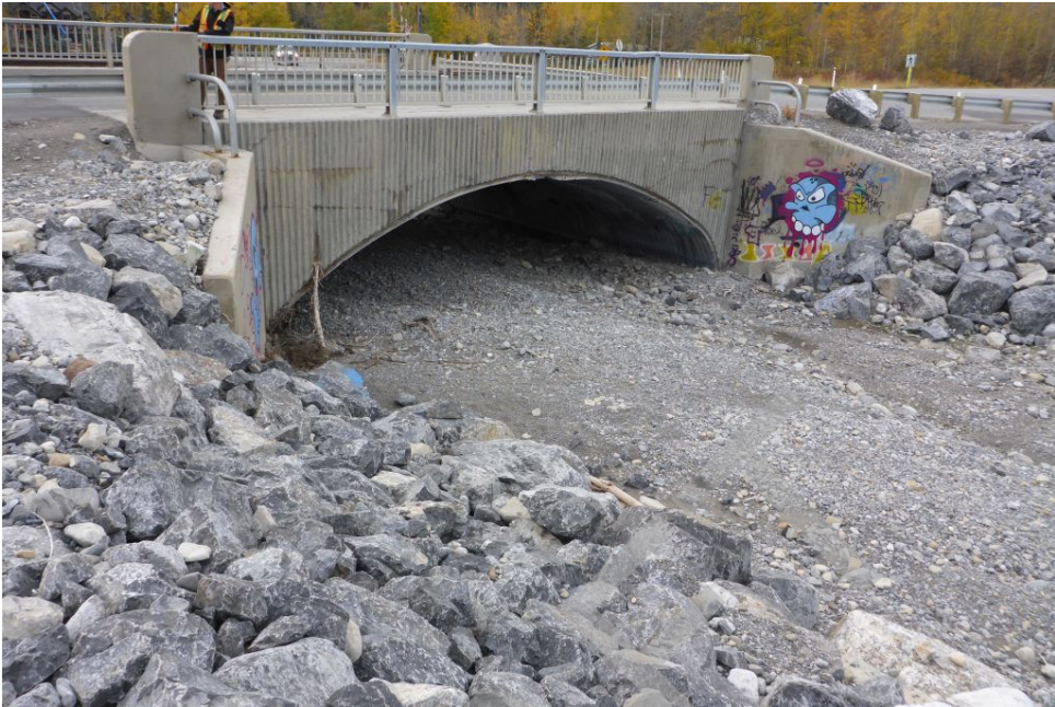
Culvert Photo 22. Exshaw Creek, 206
