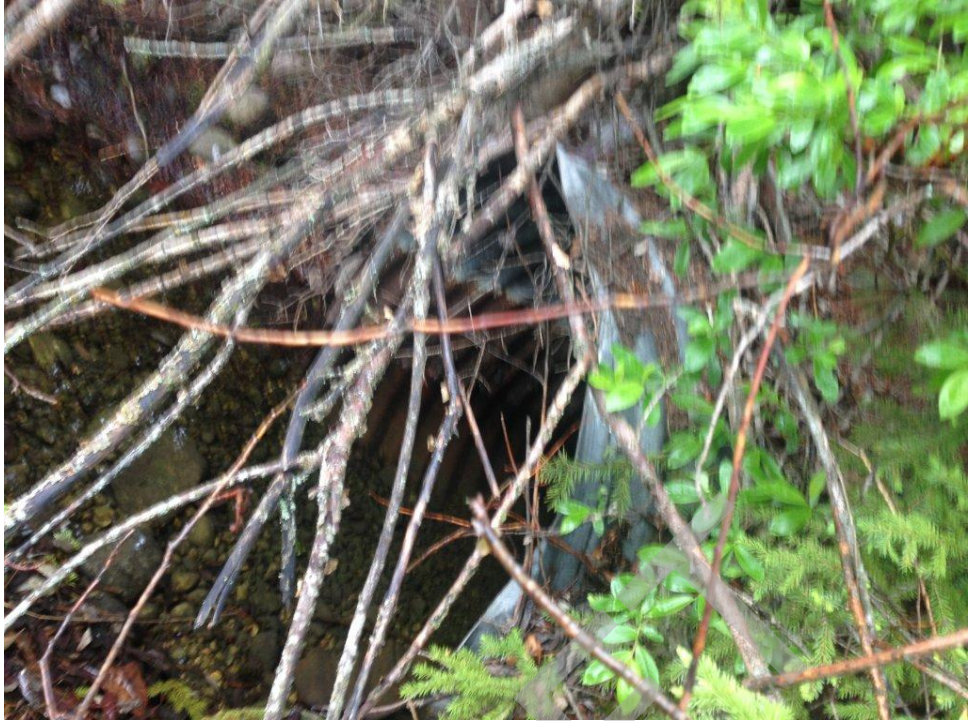
Culvert Photo 37. Side channel of Policeman Creek, 4,877
