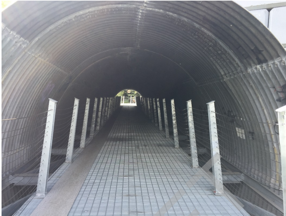
Culvert Photo 16. Bighill Creek, 480
