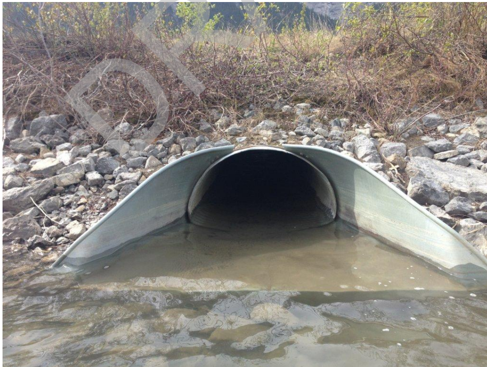
Culvert Photo 2. Bow River, 87,904
