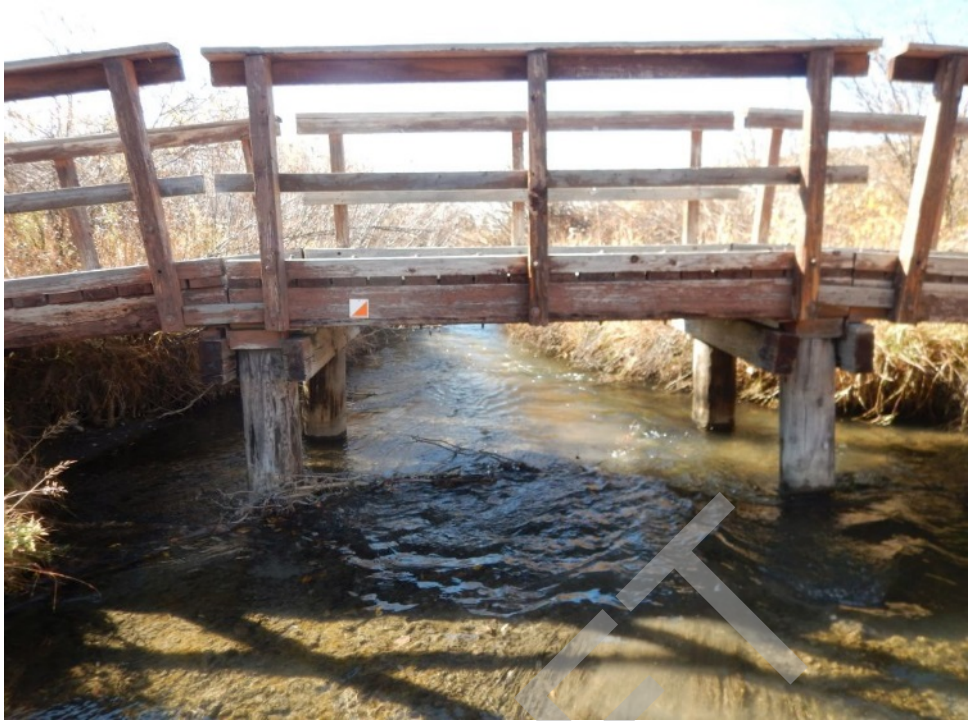
Bridge Photo 63. Bighill Creek, 3,794
