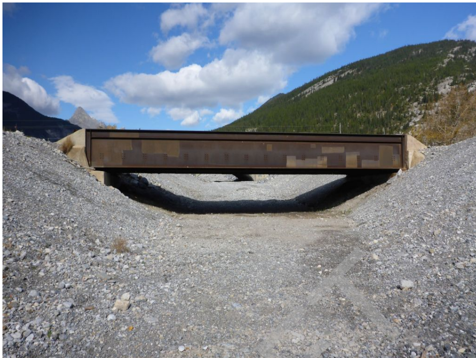
Bridge Photo 76. Exshaw Creek, 155
