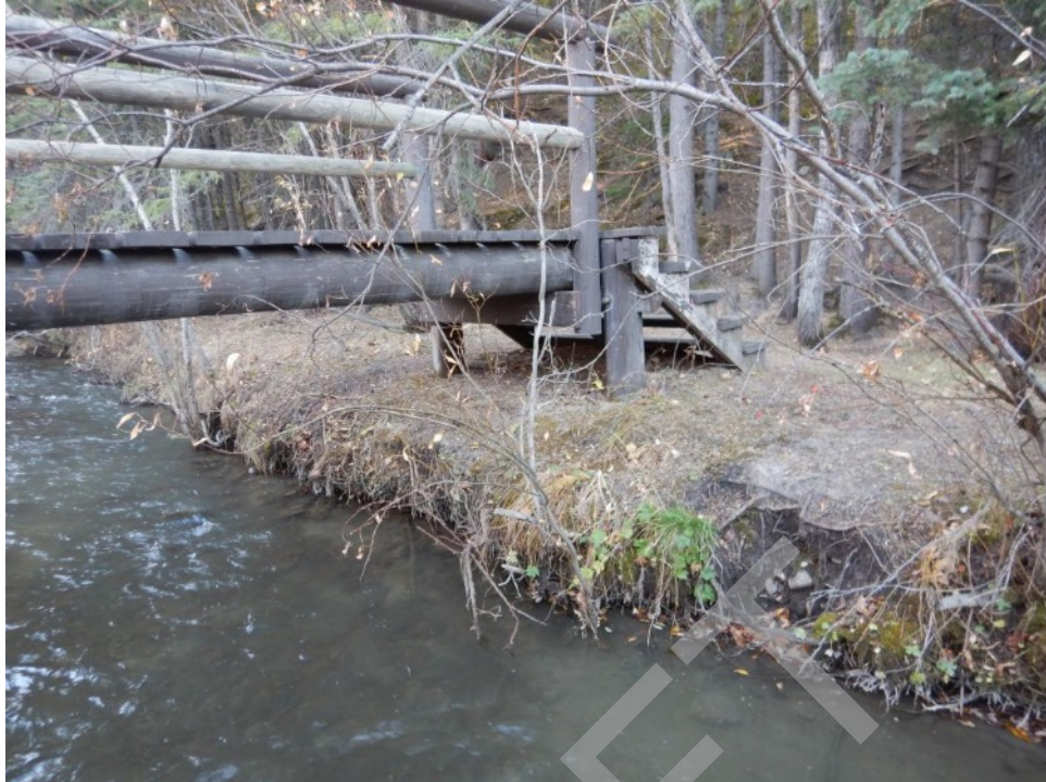
Bridge Photo 65. Bighill Creek, 4,360
