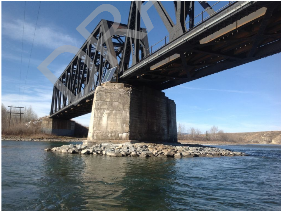
Bridge Photo 10. Bow River, 27,374
