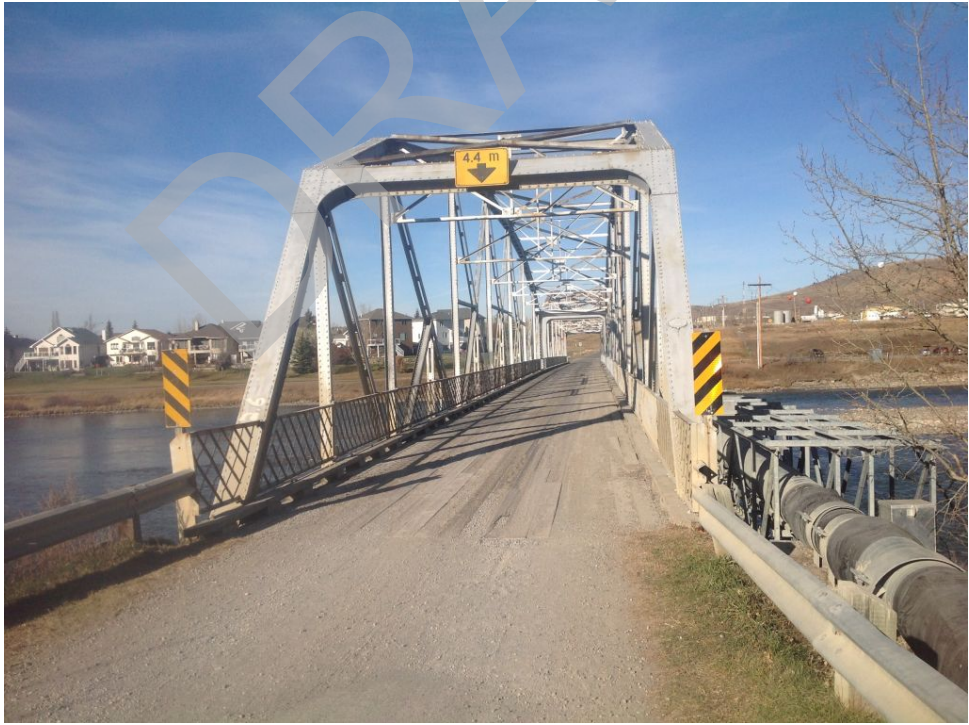
Bridge Photo 4. Bow River, 21,225
