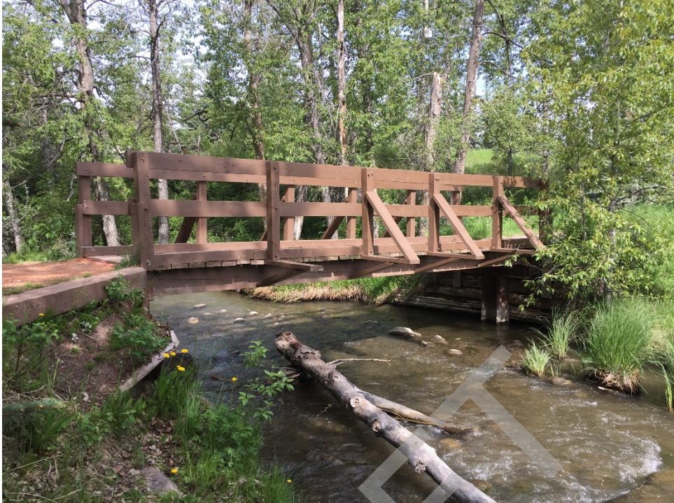
Bridge Photo 43. Bighill Creek, 1,207
