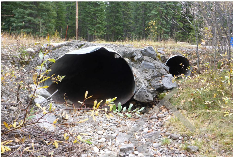
Culvert Photo 23. Policeman Creek, 4,923
