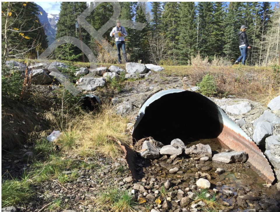
Culvert Photo 24. Policeman Creek, 4,923
