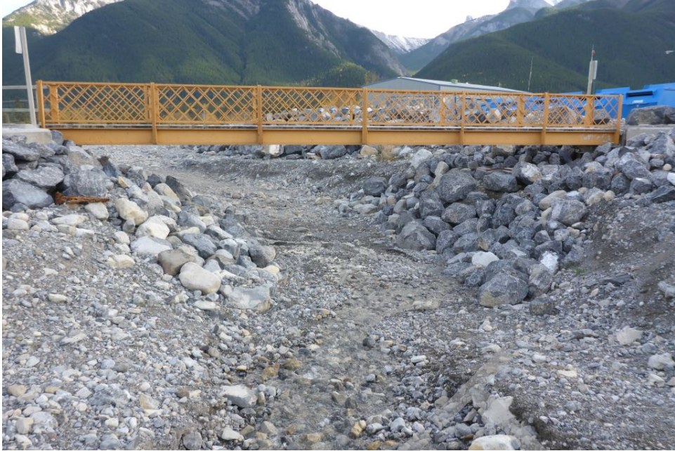
Bridge Photo 78. Exshaw Creek, 451
