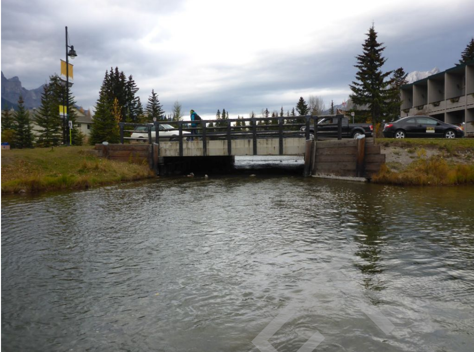
Bridge Photo 85. Policeman Creek, 3,699
