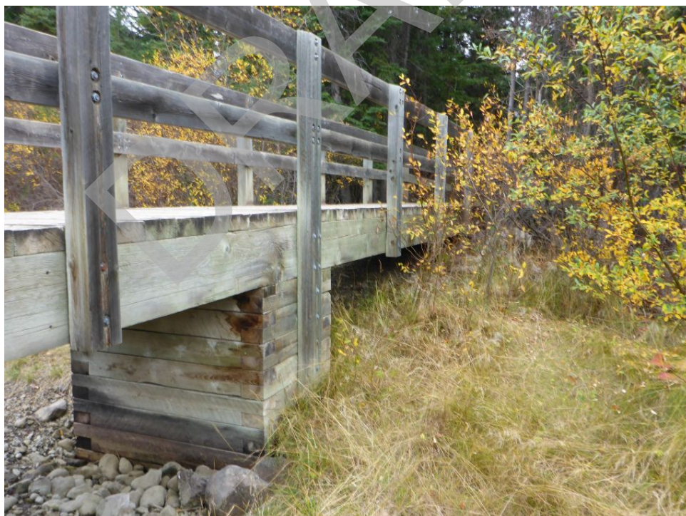
Bridge Photo 92. Policeman Creek, 4,717
