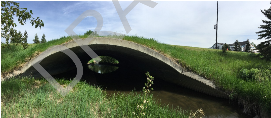
Culvert Photo 19. Bighill Creek, 2,498 (downstream)
