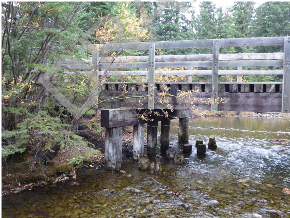
Bridge Photo 88. Policeman Creek, 4,328
