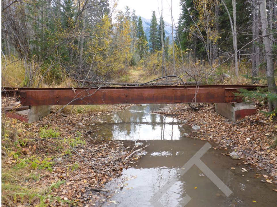
Bridge Photo 103. Policeman Creek, 6,022
