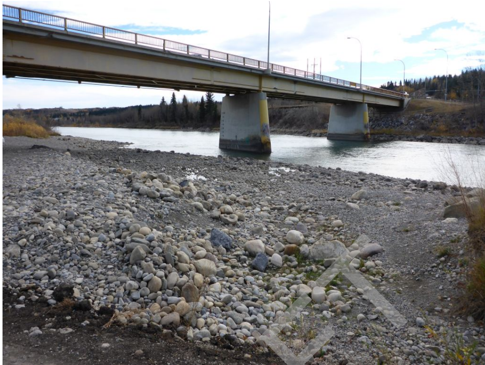
Bridge Photo 5. Bow River, 23,403
