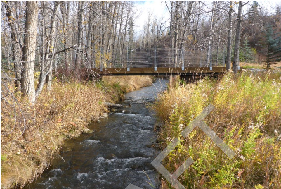
Bridge Photo 33. Bighill Creek, 208
