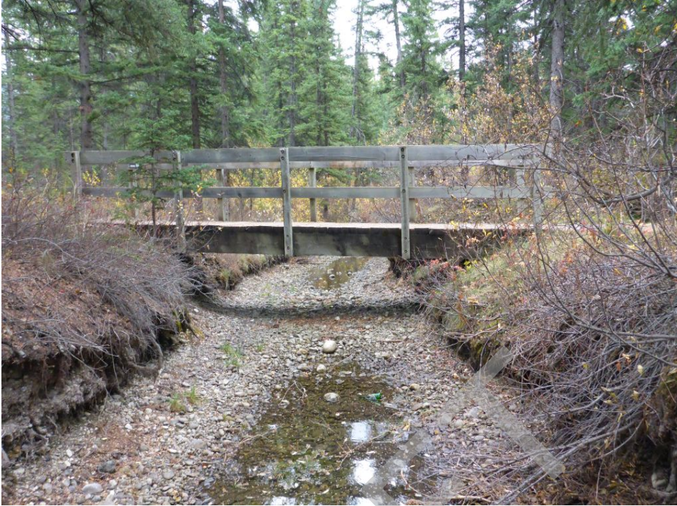
Bridge Photo 93. Policeman Creek, 4,853
