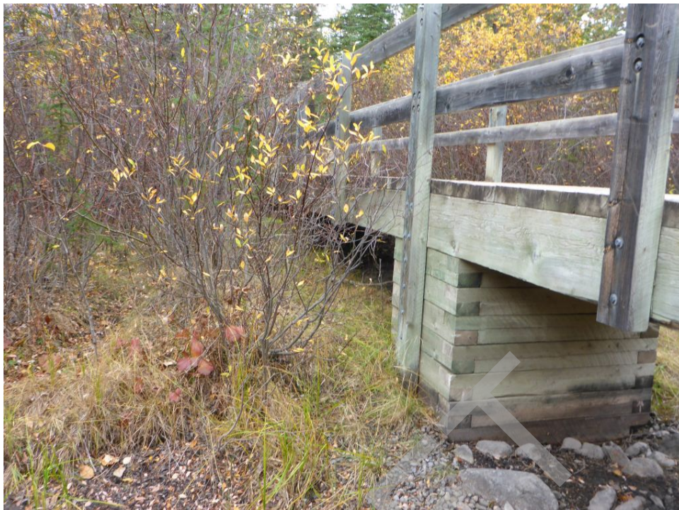
Bridge Photo 91. Policeman Creek, 4,717
