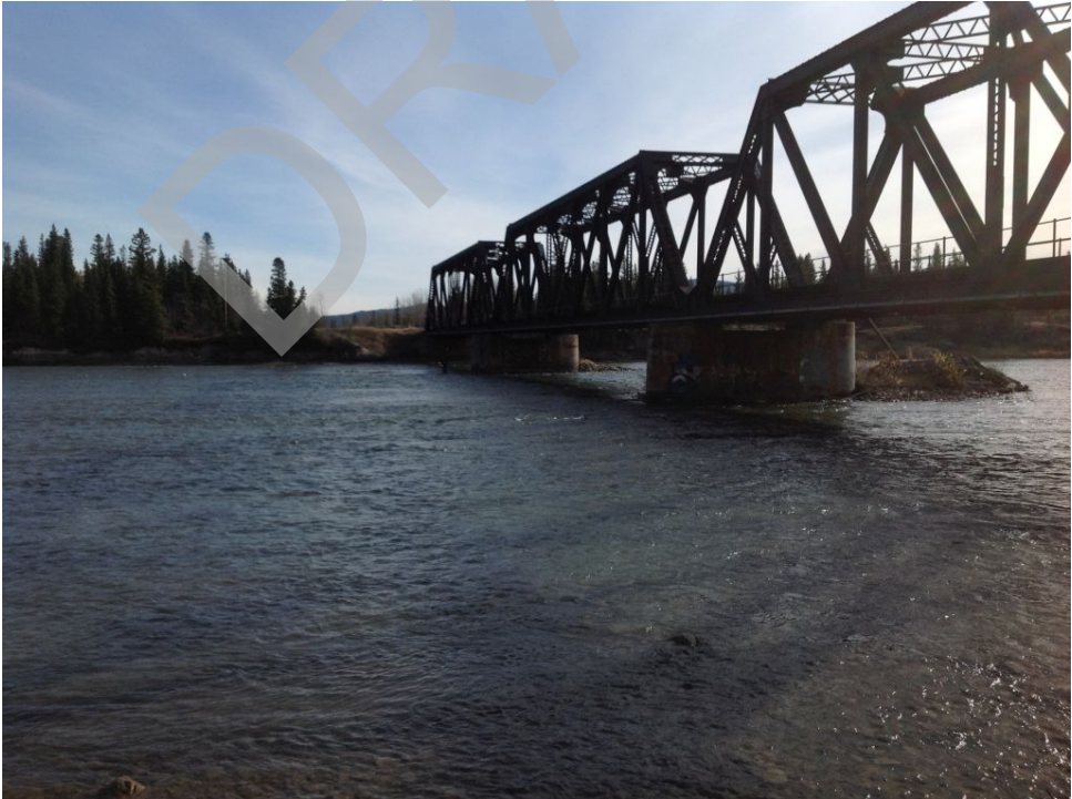
Bridge Photo 16. Bow River, 79,676
