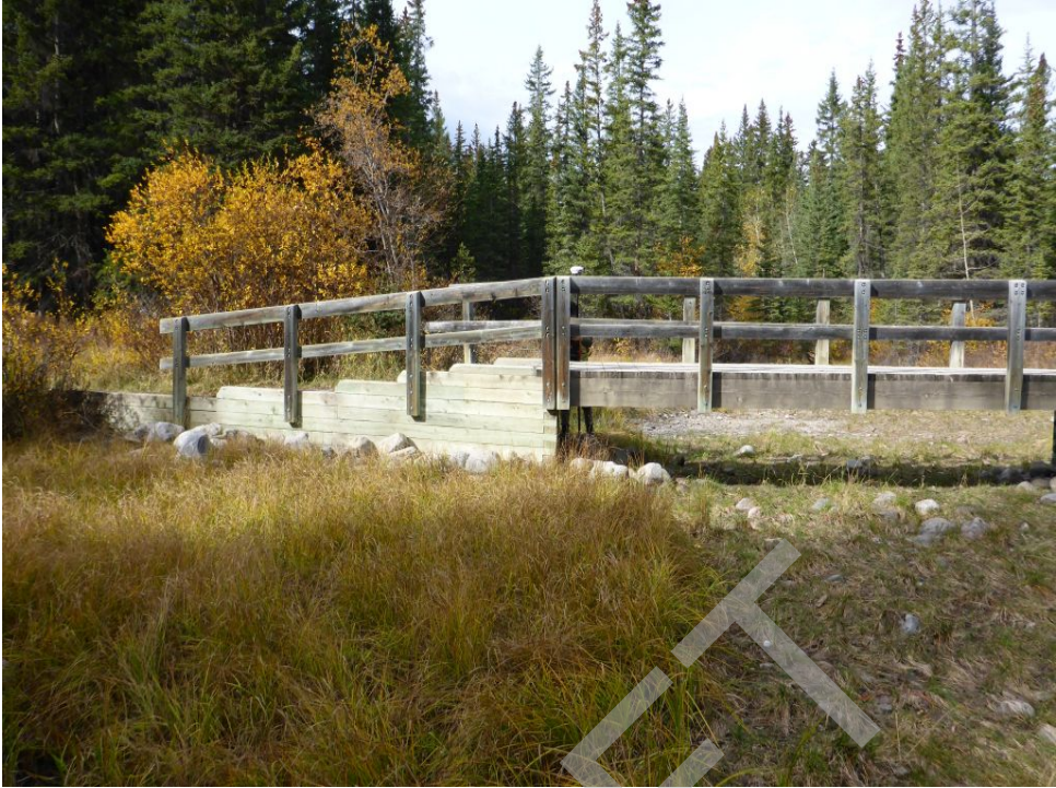
Bridge Photo 97. Policeman Creek, 5,252
