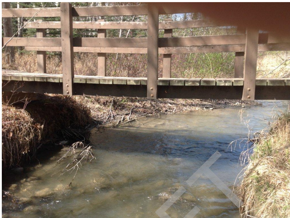
Bridge Photo 37. Bighill Creek, 372
