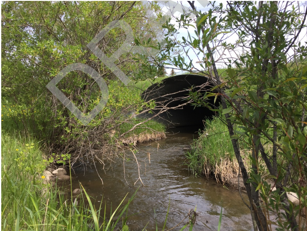
Culvert Photo 17. Bighill Creek, 1,519 (downstream)
