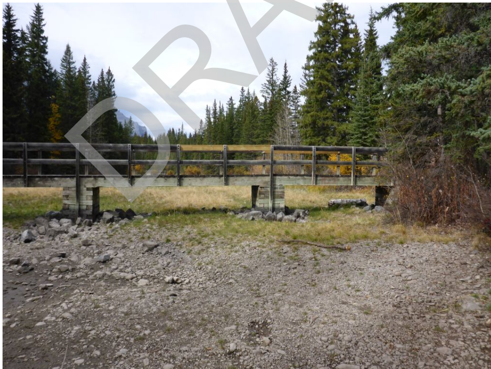
Bridge Photo 96. Policeman Creek, 5,103
