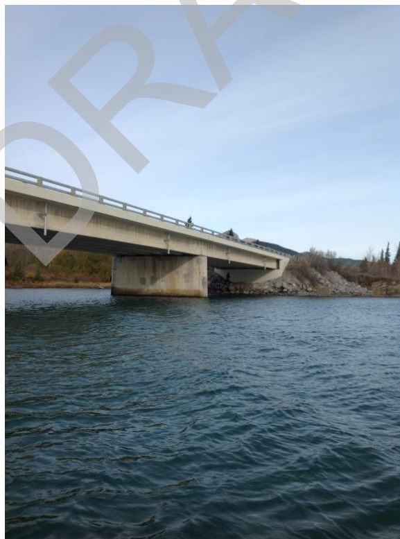
Bridge Photo 14. Bow River, 77,639
