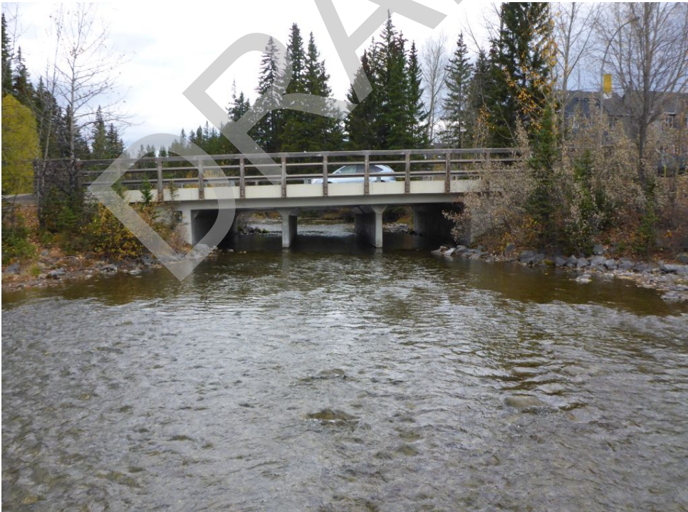
Bridge Photo 86. Policeman Creek, 3,876
