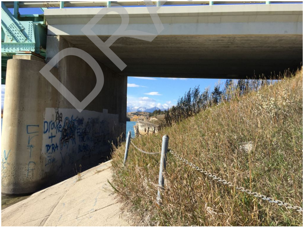
Bridge Photo 12. Bow River, 54,457
