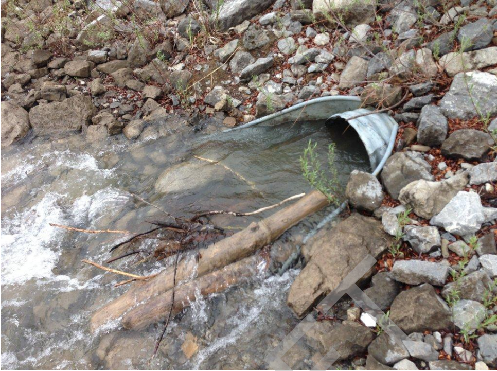
Culvert Photo 7. Bow River, 91,122
