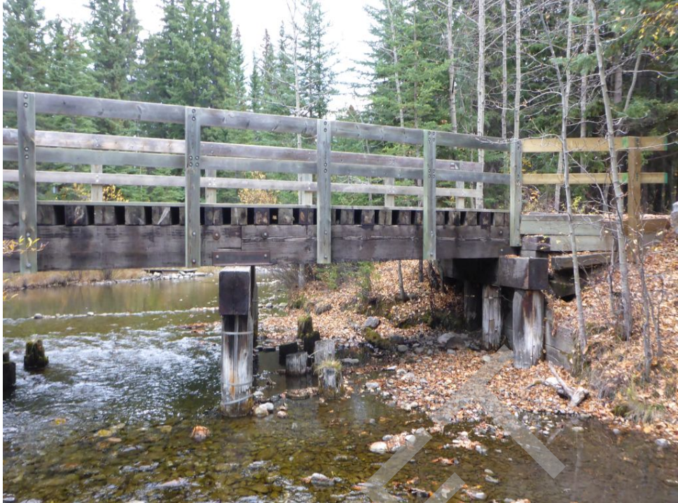
Bridge Photo 89. Policeman Creek, 4,328
