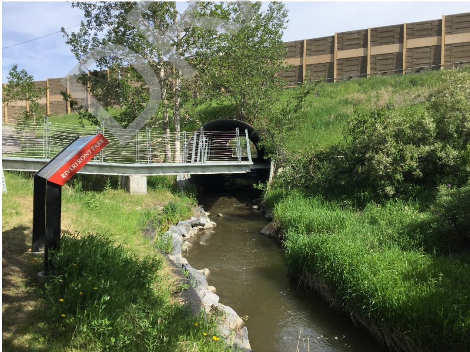
Culvert Photo 15. Bighill Creek, 480 (downstream)
