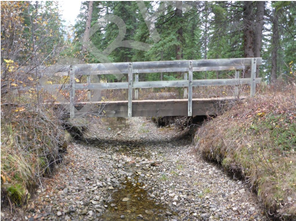
Bridge Photo 94. Policeman Creek, 4,853
