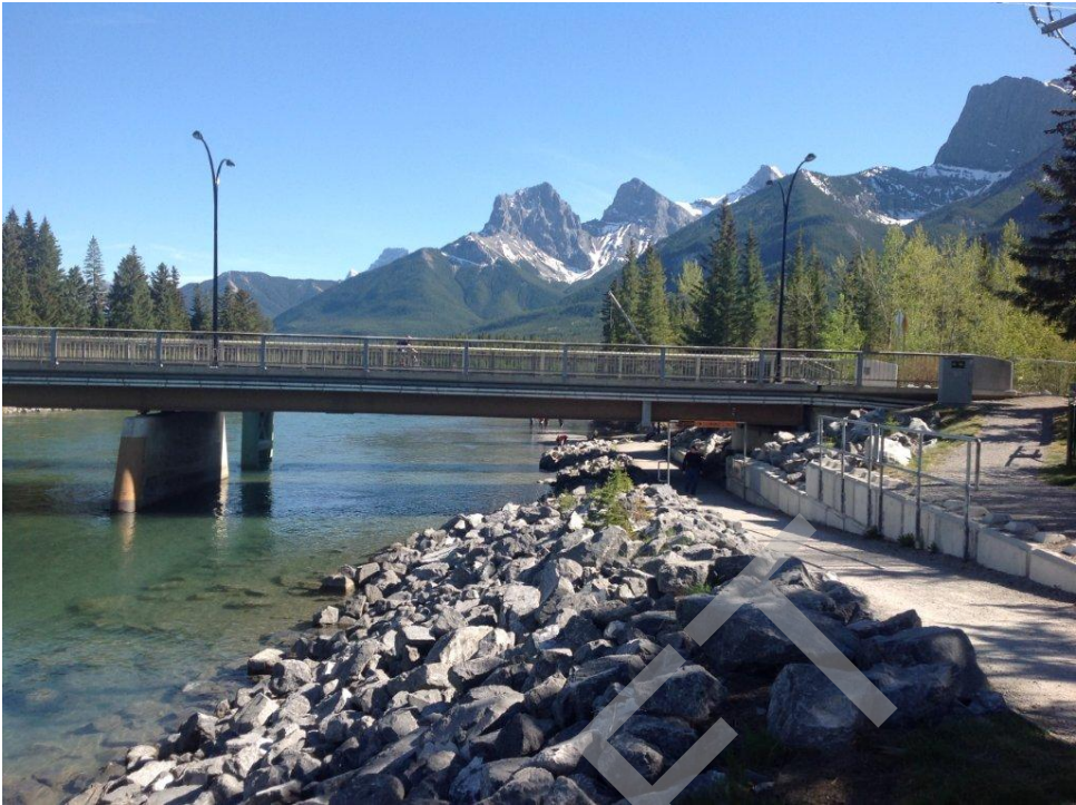
Bridge Photo 23. Bow River, 109,223
