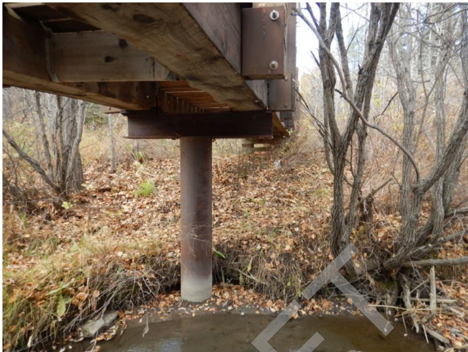
Bridge Photo 41. Bighill Creek, 992
