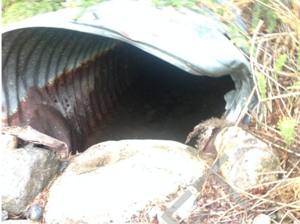
Culvert Photo 35. Side channel of Policeman Creek, 4,877
