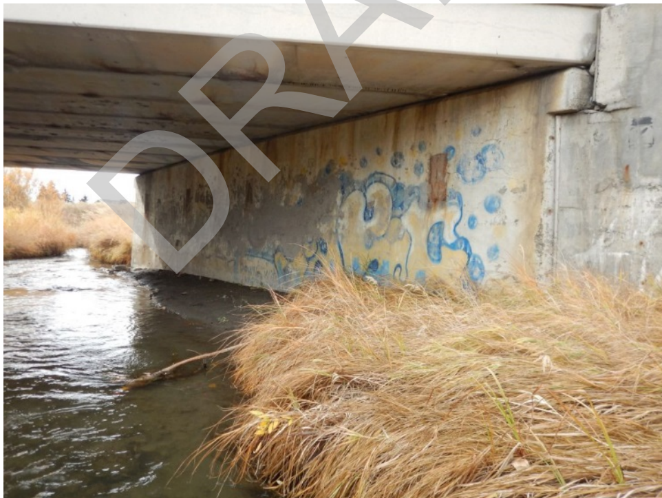
Bridge Photo 58. Bighill Creek, 2,814
