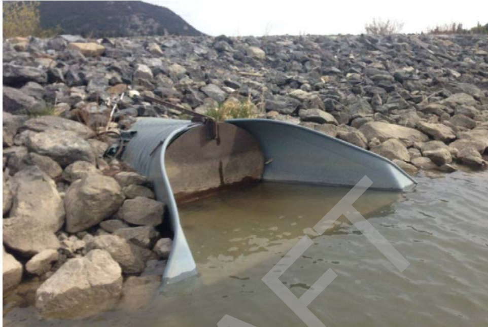
Culvert Photo 1. Bow River, 87,721
