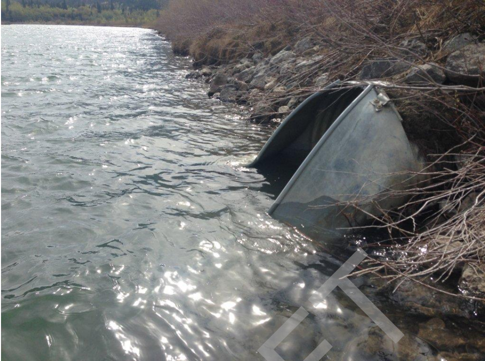
Culvert Photo 3. Bow River, 88,087
