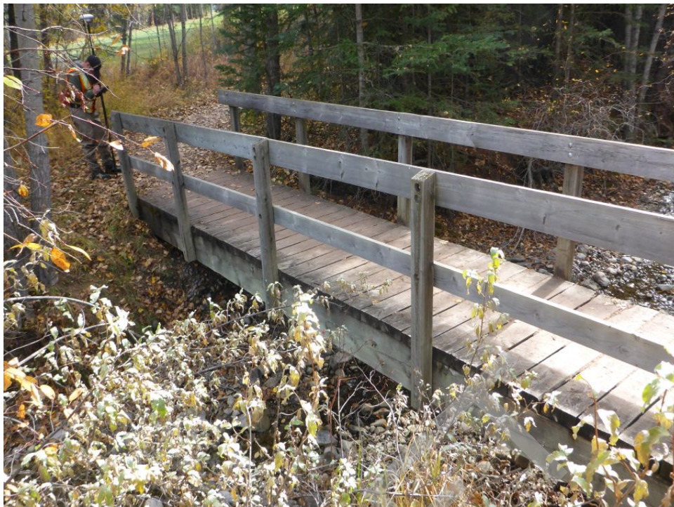
Bridge Photo 99. Policeman Creek, 5,648
