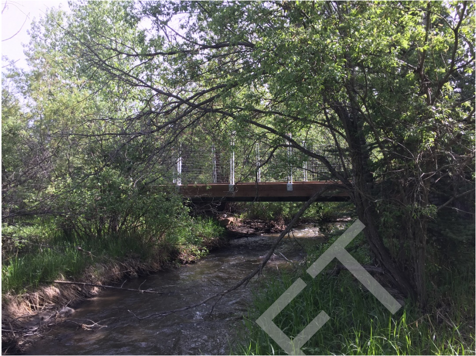
Bridge Photo 39. Bighill Creek, 581
