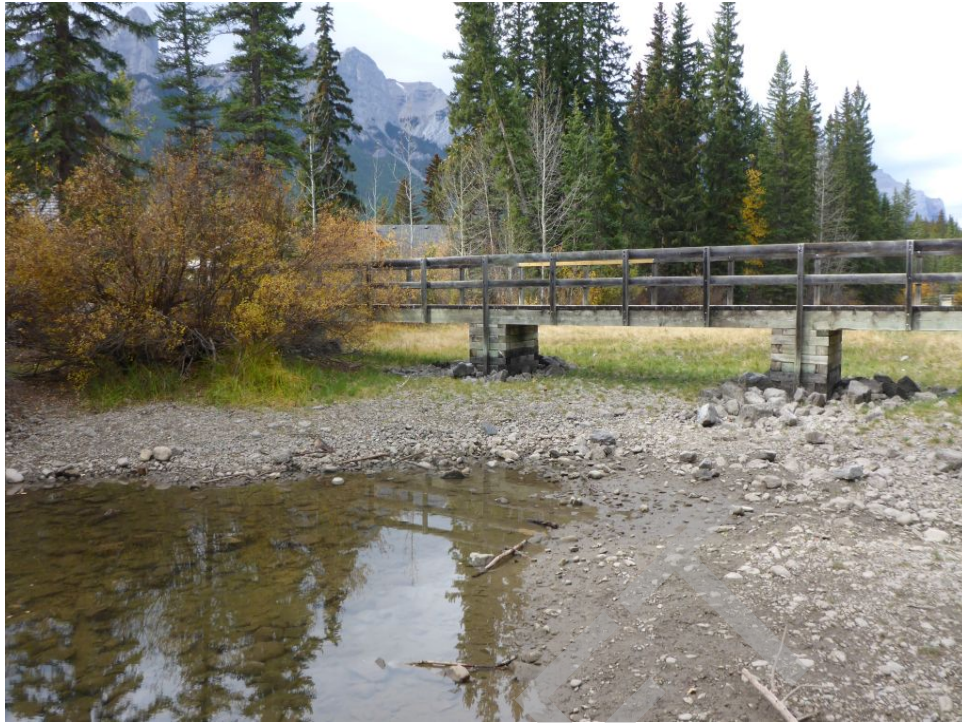
Bridge Photo 95. Policeman Creek, 5,103
