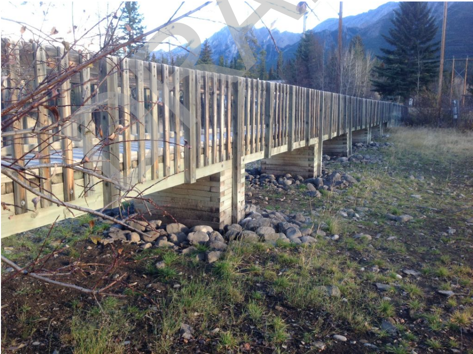
Bridge Photo 106. Side channel of Policeman Creek, 5,331
