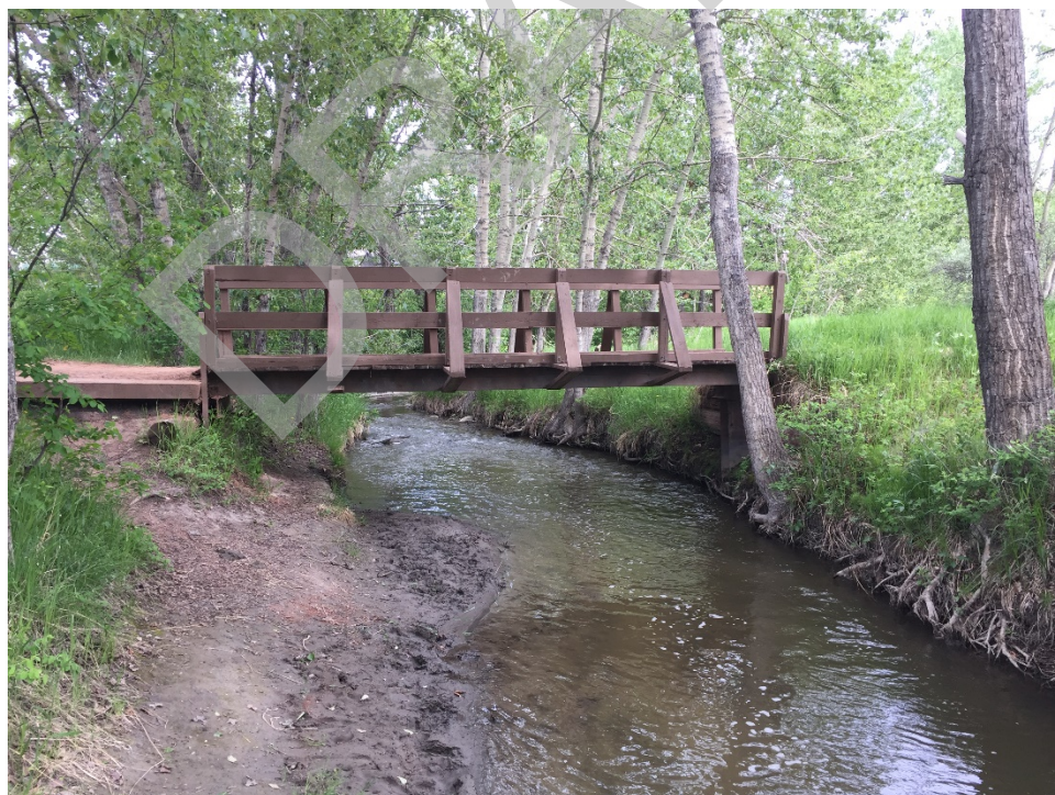
Bridge Photo 46. Bighill Creek, 1,722
