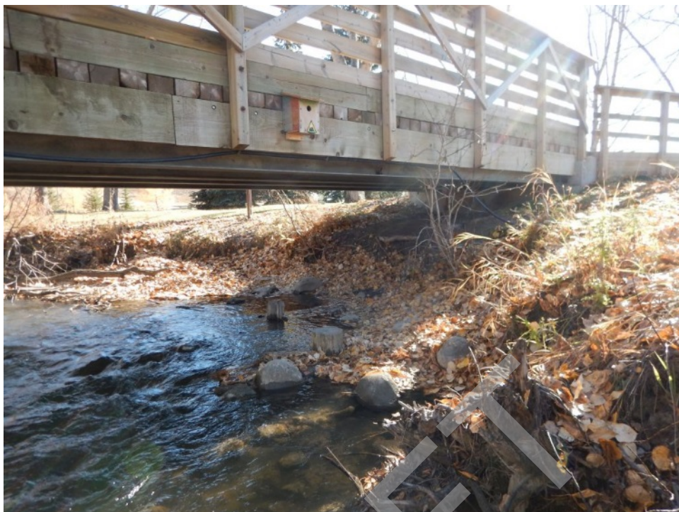
Bridge Photo 61. Bighill Creek, 3,385
