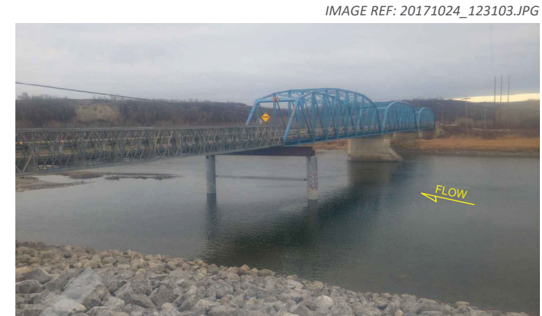
1. View looking downstream from left bank. Note that the construction cofferdam, as shown in the aerial image to the left, had been removed prior to river surveying.
