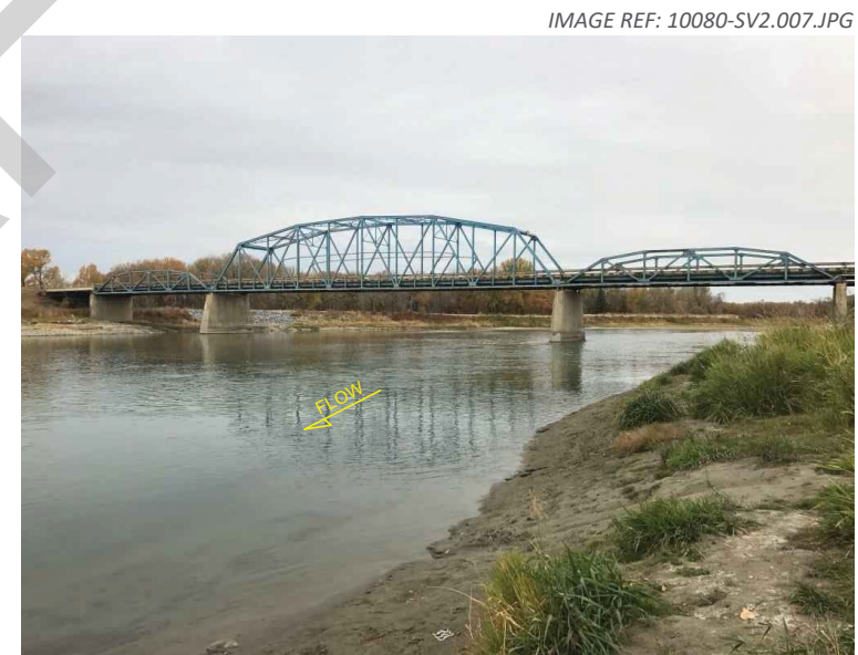
2. View looking upstream from left bank.
