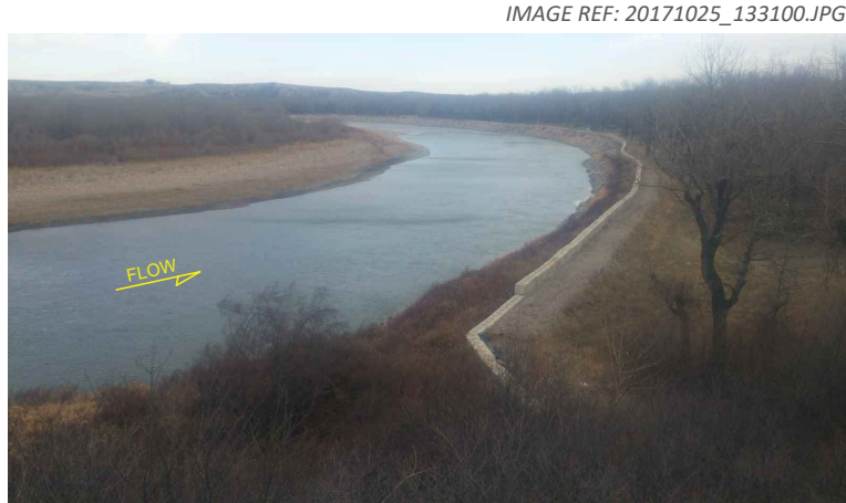
3. View looking downstream from the upstream end of the upper berm.
