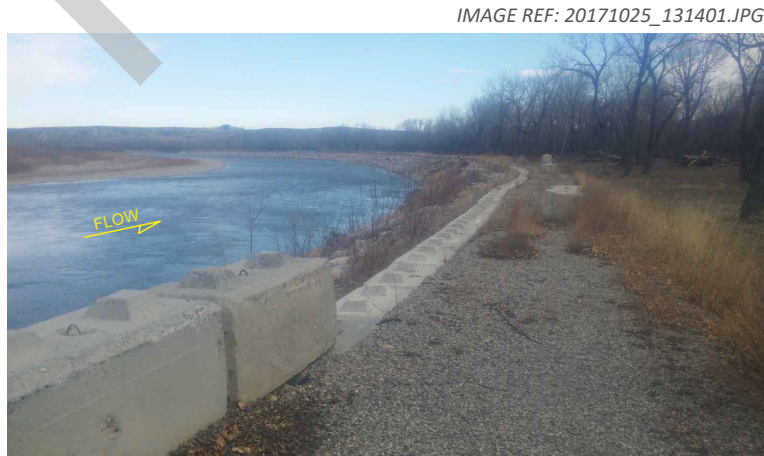
2. View looking downstream at the upper berm midway along its length.
