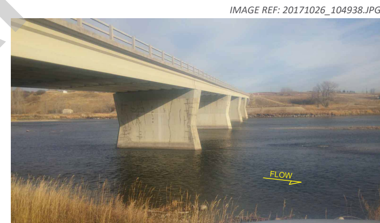
2. View looking across the river from right bank.
