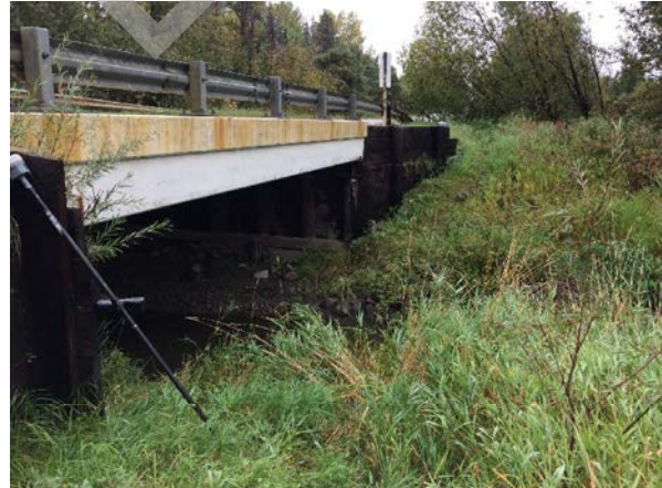
PHOTO 2 LEFT BANK, LOOKING DOWNSTREAM
