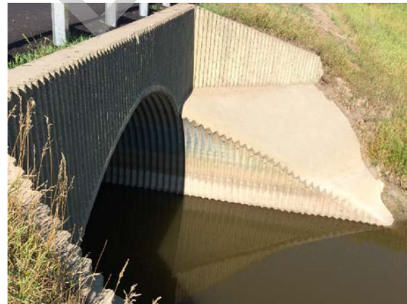
PHOTO 2 LEFT BANK, LOOKING DOWNSTREAM
