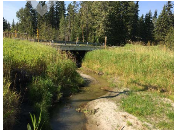
PHOTO 2 LEFT BANK, LOOKING DOWNSTREAM
