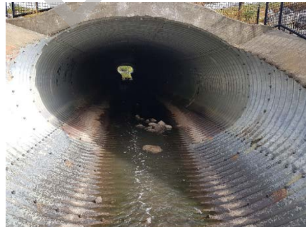
PHOTO 2 UPSTREAM END, LOOKING DOWNSTREAM
