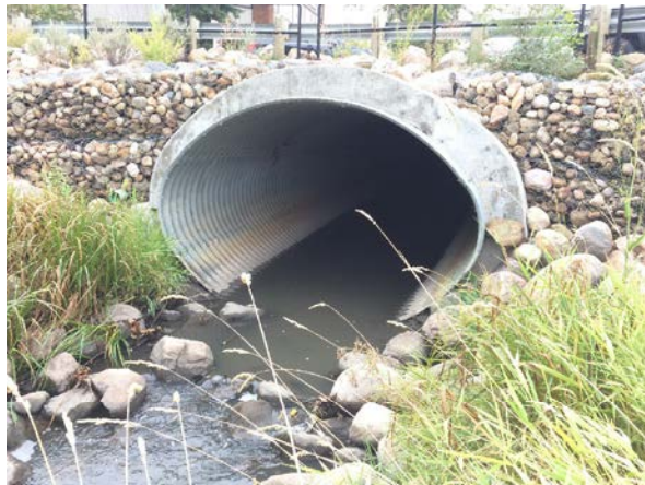
PHOTO 1 LEFT BANK, LOOKING UPSTREAM
