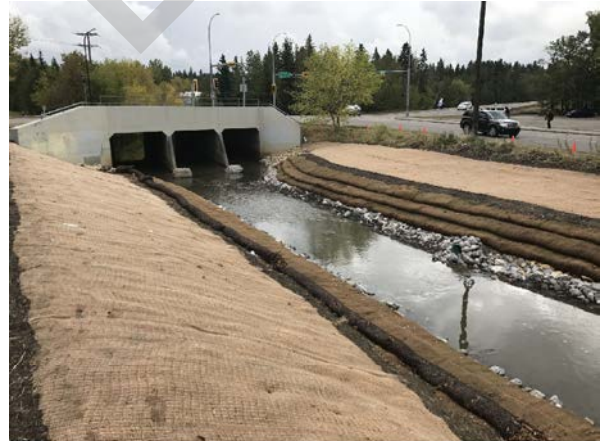
PHOTO 2 LEFT BANK, LOOKING DOWNSTREAM
