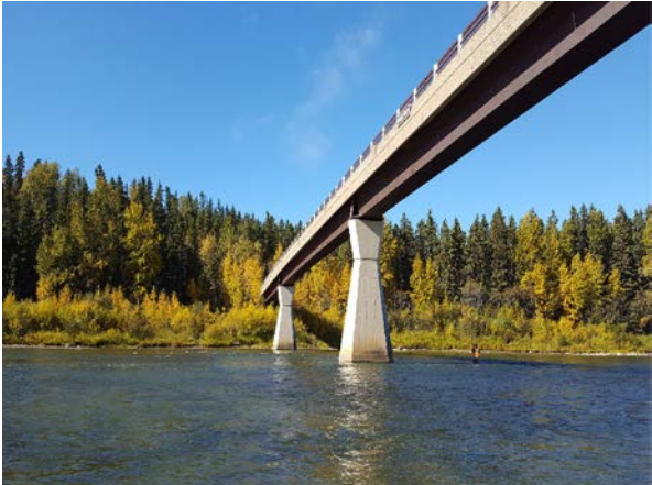
PHOTO 1 LEFT BANK, LOOKING UPSTREAM
