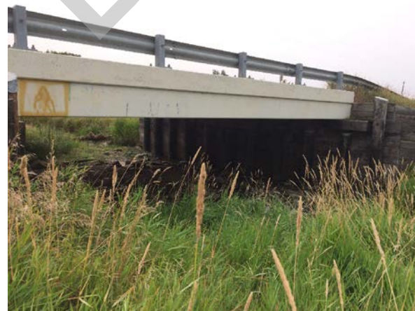
PHOTO 2 LEFT BANK, LOOKING DOWNSTREAM
