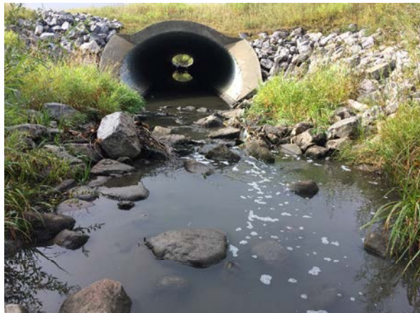
PHOTO 1 DOWNSTREAM END, LOOKING UPSTREAM
