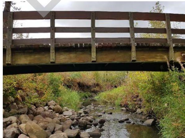
PHOTO 2 LEFT BANK, LOOKING DOWNSTREAM
