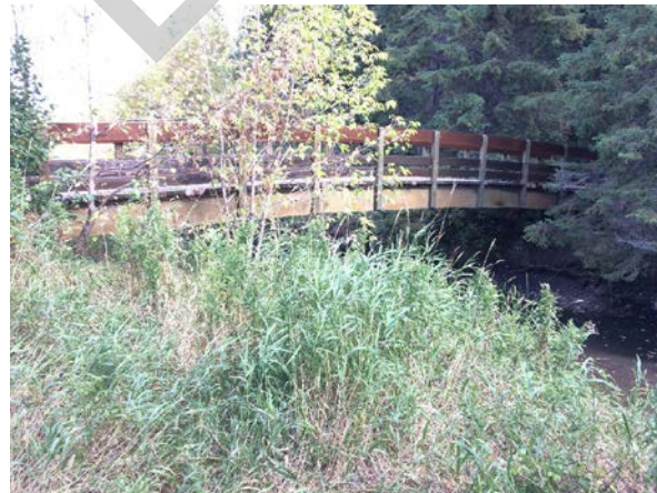
PHOTO 2 LEFT BANK, LOOKING DOWNSTREAM
