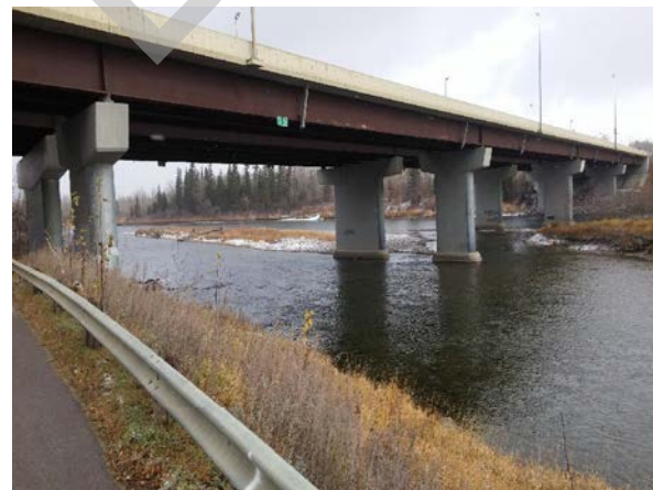
PHOTO 2 LEFT BANK, LOOKING DOWNSTREAM
