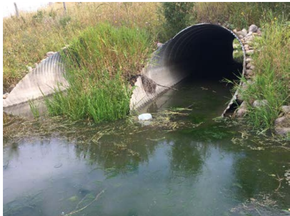
PHOTO 1 LEFT BANK, LOOKING UPSTREAM
