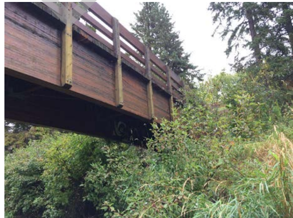
PHOTO 2 LEFT BANK, LOOKING DOWNSTREAM
