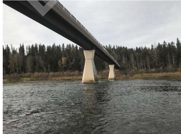
PHOTO 2 LEFT BANK, LOOKING DOWNSTREAM
