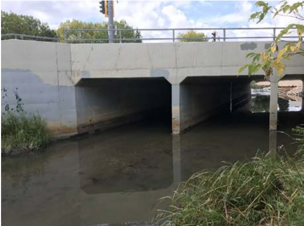
PHOTO 1 LEFT BANK, LOOKING UPSTREAM
