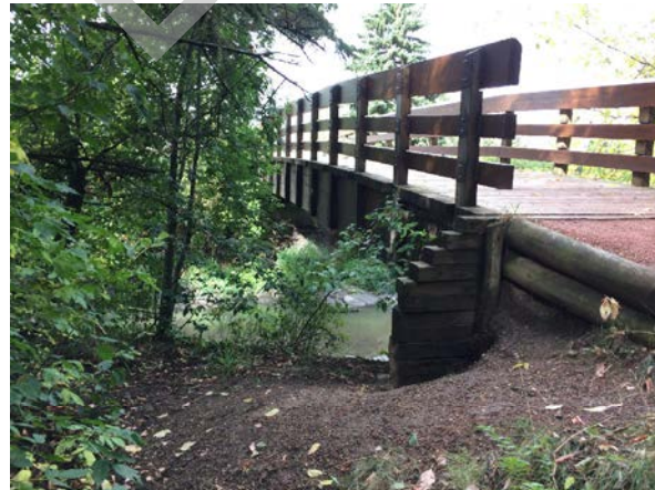
PHOTO 2 BRIDGE RIGHT BANK
