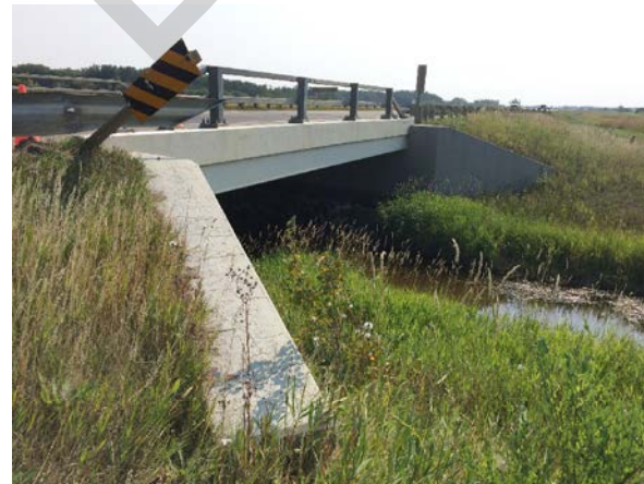
PHOTO 2 LEFT BANK, LOOKING DOWNSTREAM
