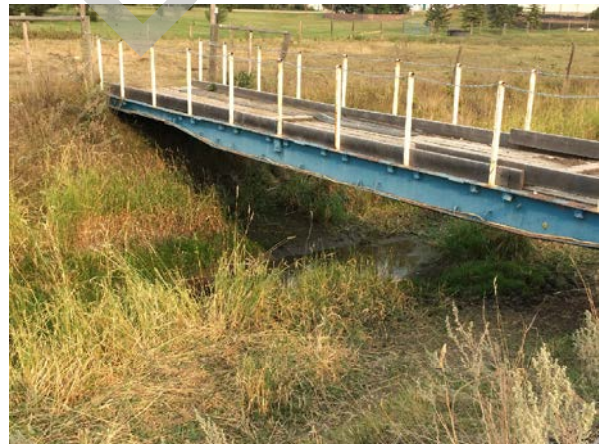
PHOTO 2 RIGHT BANK, LOOKING DOWNSTREAM
