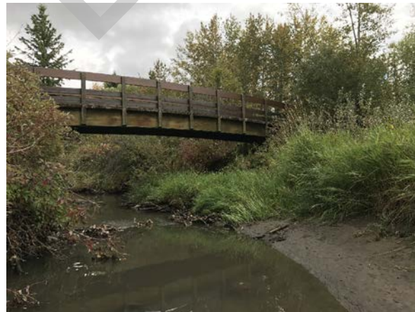
PHOTO 2 LEFT BANK, LOOKING DOWNSTREAM
