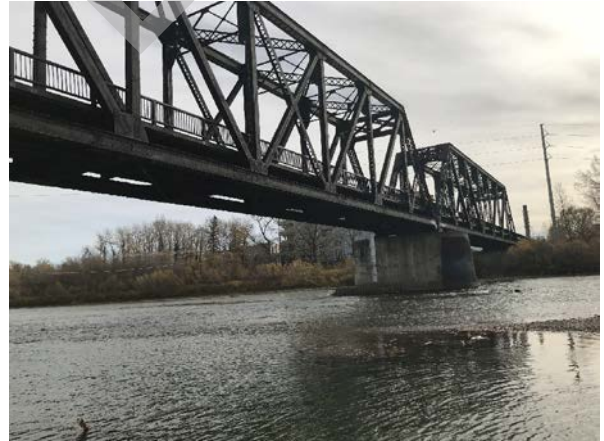
PHOTO 2 LEFT BANK, LOOKING DOWNSTREAM
