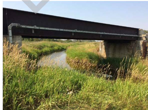
PHOTO 2 LEFT BANK, LOOKING DOWNSTREAM
