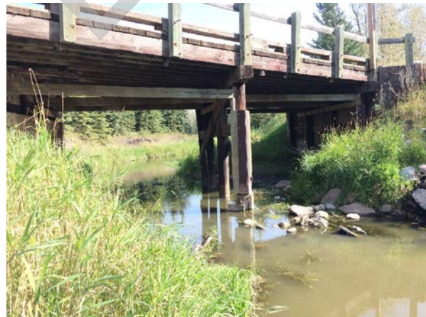
PHOTO 2 LEFT BANK, LOOKING DOWNSTREAM
