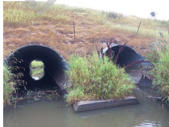
PHOTO 2 LEFT BANK, LOOKING DOWNSTREAM
