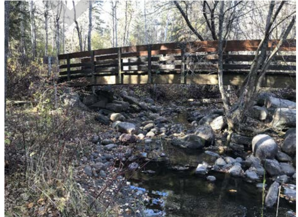
PHOTO 2 LEFT BANK, LOOKING DOWNSTREAM
