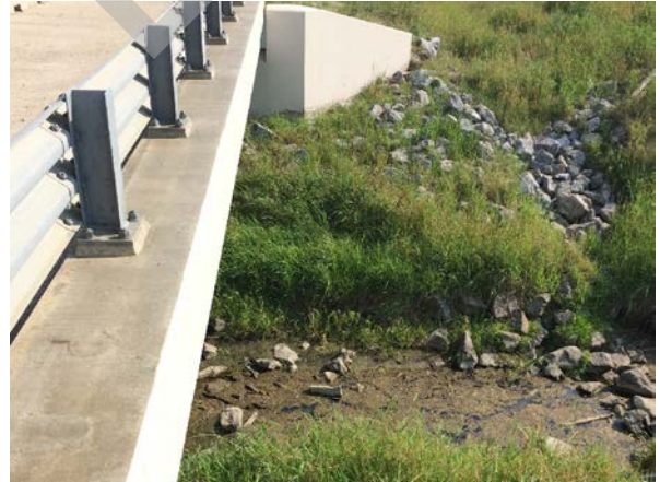
PHOTO 2 RIGHT BANK ABUTMENT
