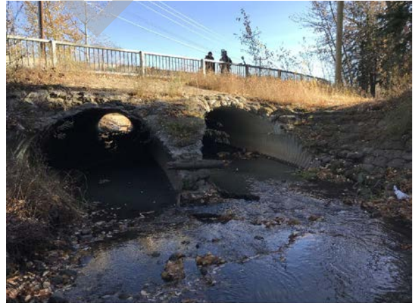
PHOTO 2 LEFT BANK, LOOKING DOWNSTREAM
