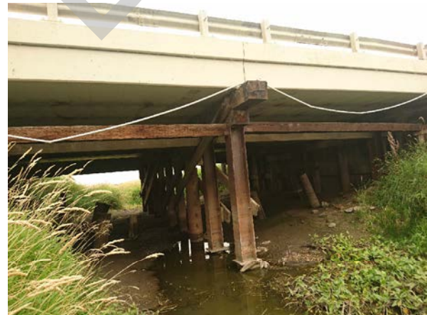
PHOTO 2 LEFT BANK, LOOKING DOWNSTREAM
