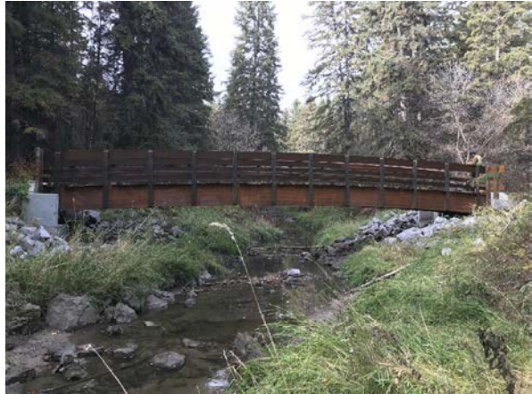
PHOTO 1 LEFT BANK, LOOKING UPSTREAM
