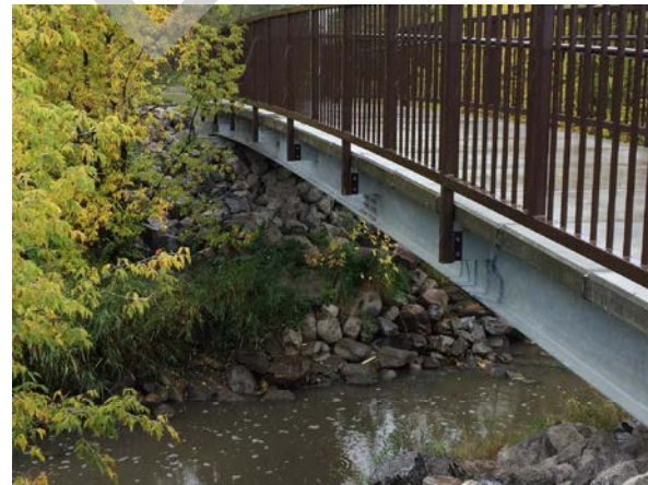
PHOTO 2 RIGHT BANK, LOOKING DOWNSTREAM
