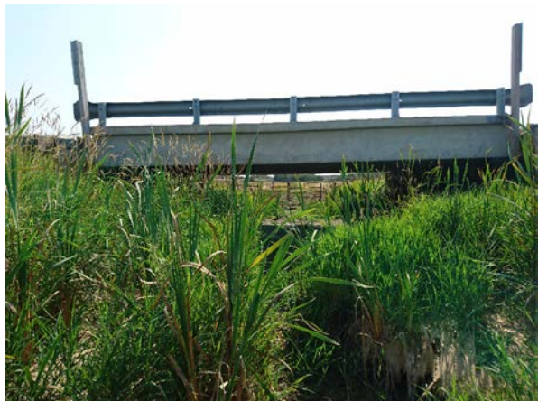
PHOTO 1 DOWNSTREAM END, LOOKING UPSTREAM
