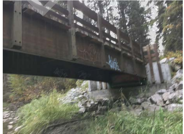
PHOTO 2 RIGHT BANK ABUTMENT
