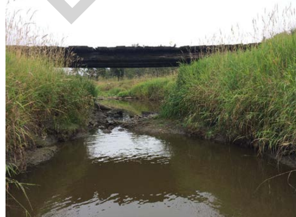
PHOTO 2 UPSTREAM END, LOOKING DOWNSTREAM
