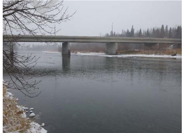
PHOTO 2 LEFT BANK, LOOKING DOWNSTREAM
