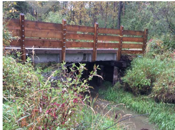
PHOTO 2 LEFT BANK, LOOKING DOWNSTREAM
