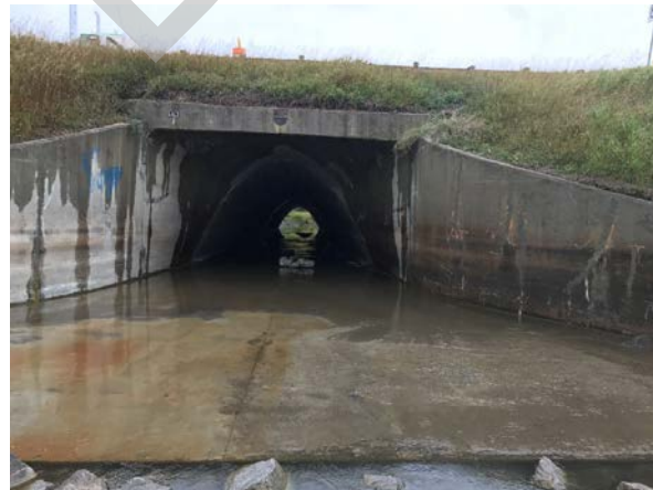
PHOTO 2 UPSTREAM END, LOOKING DOWNSTREAM
