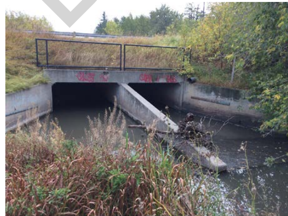
PHOTO 2 LEFT BANK, LOOKING DOWNSTREAM
