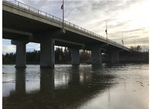
PHOTO 2 LEFT BANK, LOOKING DOWNSTREAM
