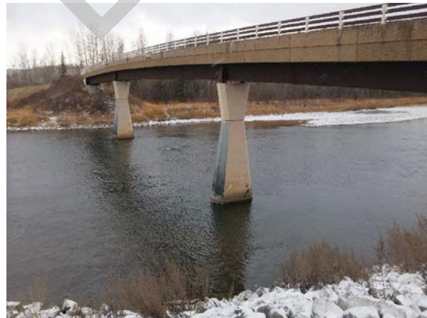
PHOTO 2 RIGHT BANK, LOOKING DOWNSTREAM
