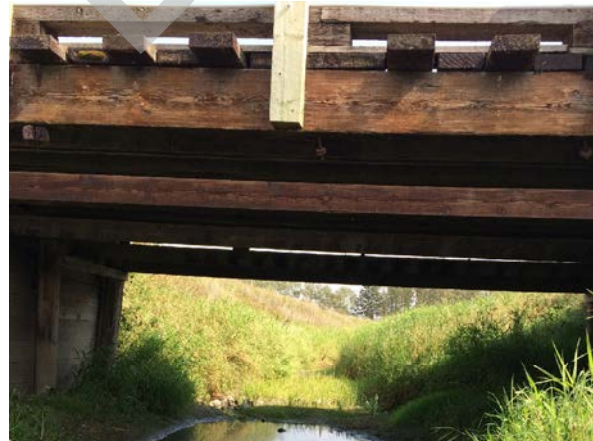
PHOTO 2 UPSTREAM END, LOOKING DOWNSTREAM
