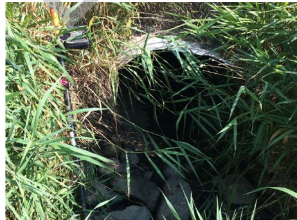
PHOTO 2 UPSTREAM END, LOOKING DOWNSTREAM
