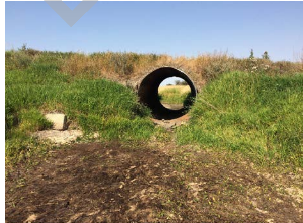
PHOTO 2 UPSTREAM END, LOOKING DOWNSTREAM
