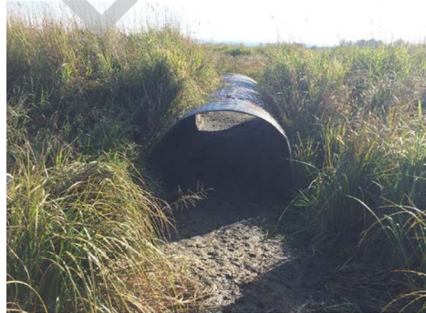
PHOTO 2 UPSTREAM END, LOOKING DOWNSTREAM
