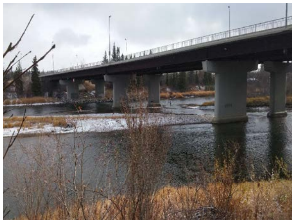
PHOTO 1 LEFT BANK, LOOKING UPSTREAM
