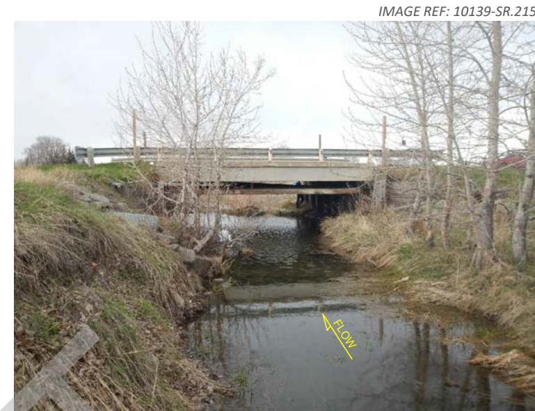
1. View looking downstream from left bank.
