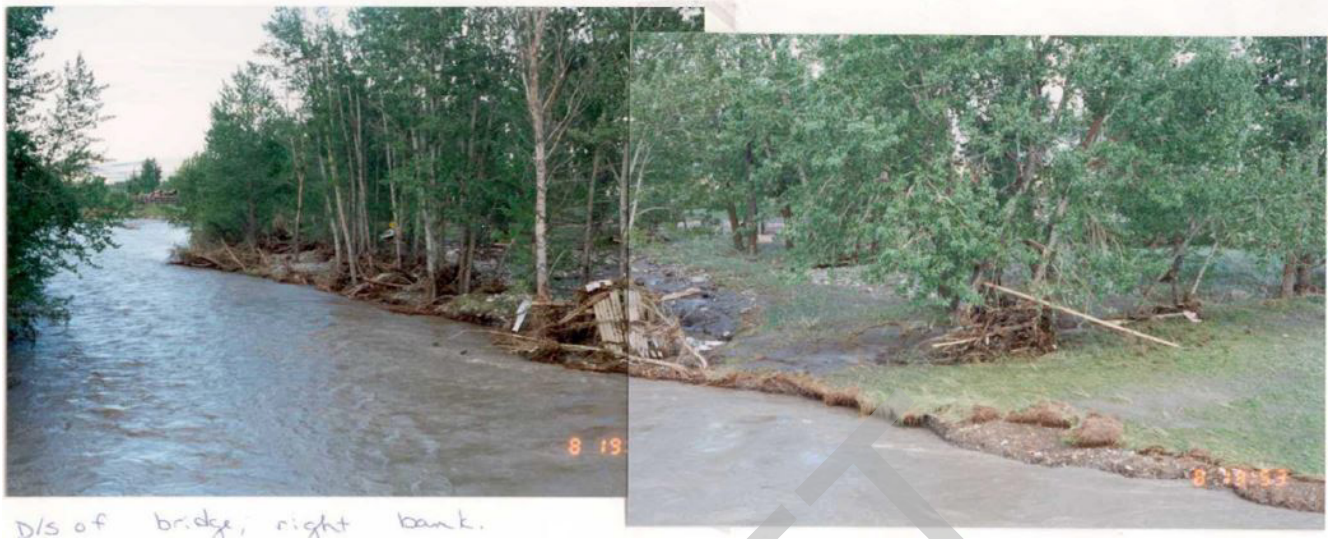
Figure IV.7 Looking Downstream of Highway 6 Bridge
