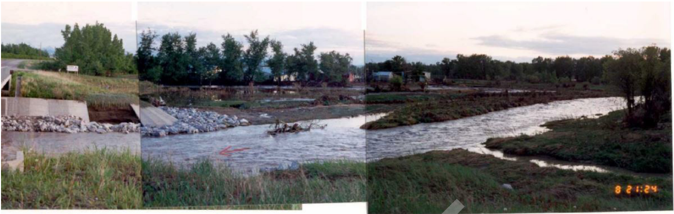
Figure IV.10 Flood Damage looking Upstream from Highway 785 Bridge
