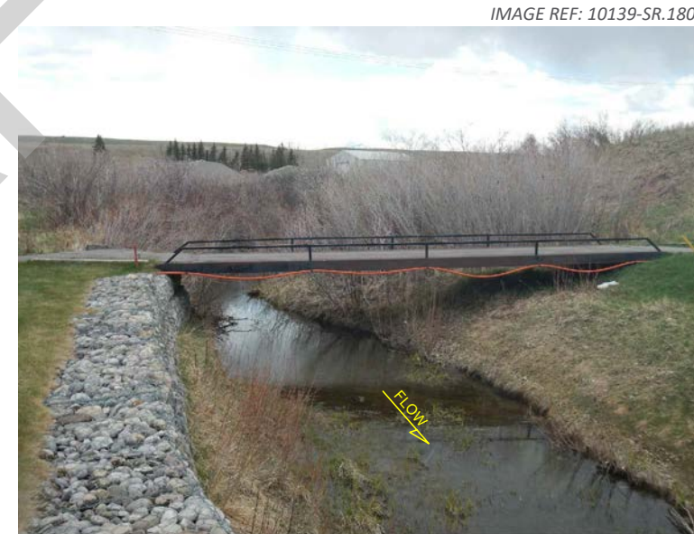
2. View looking upstream from the top of the right bank revetment.
