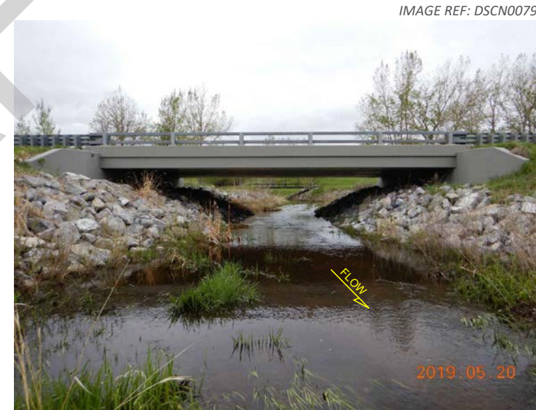
2. View looking upstream from right bank.
