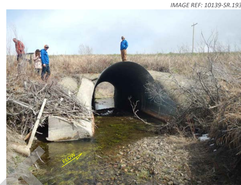
1. View looking downstream from left bank.
