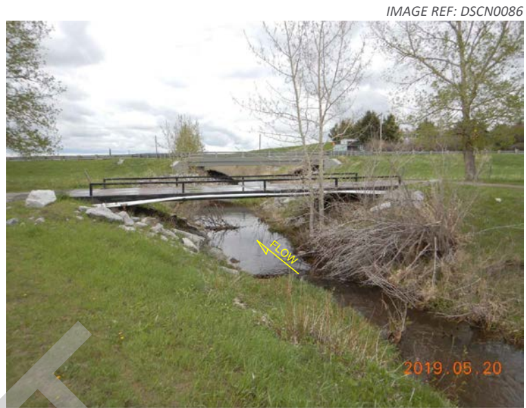
1. View looking downstream from left bank.
