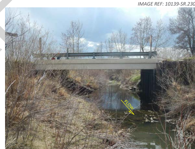
2. View looking upstream from right bank.
