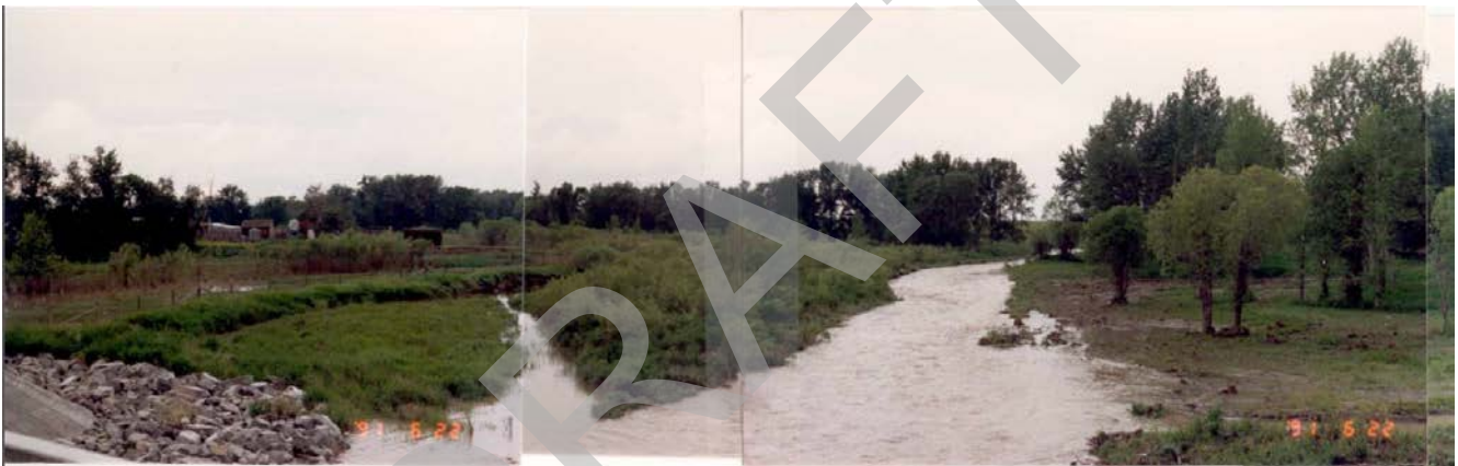
Figure IV.11 Washout Identified on Township Road 301 Bridge Over Kettles Creek
