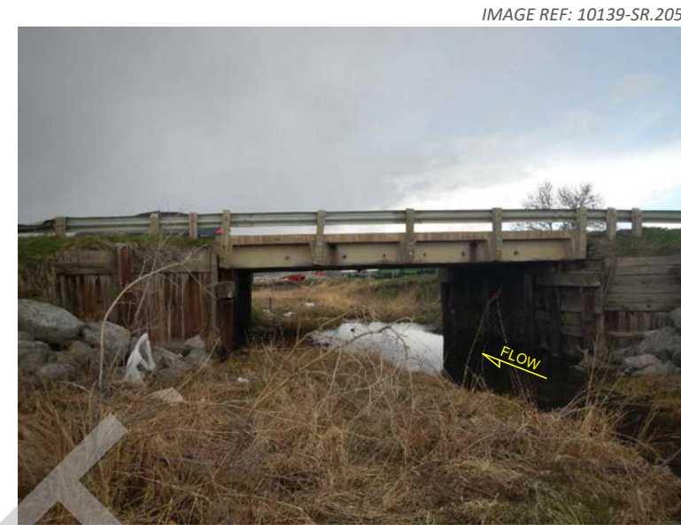
1. View looking downstream from left bank.
