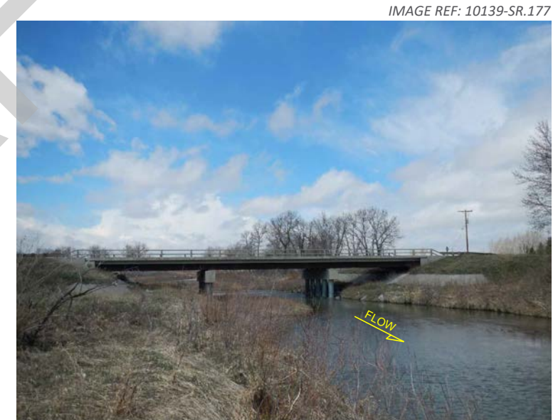
2. View looking upstream from right bank.
