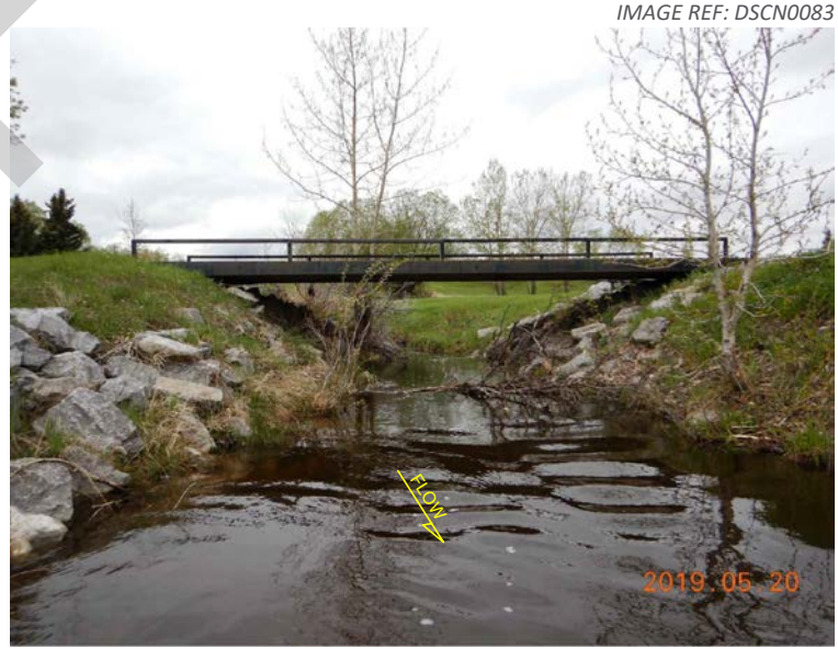
2. View looking upstream from right bank.
