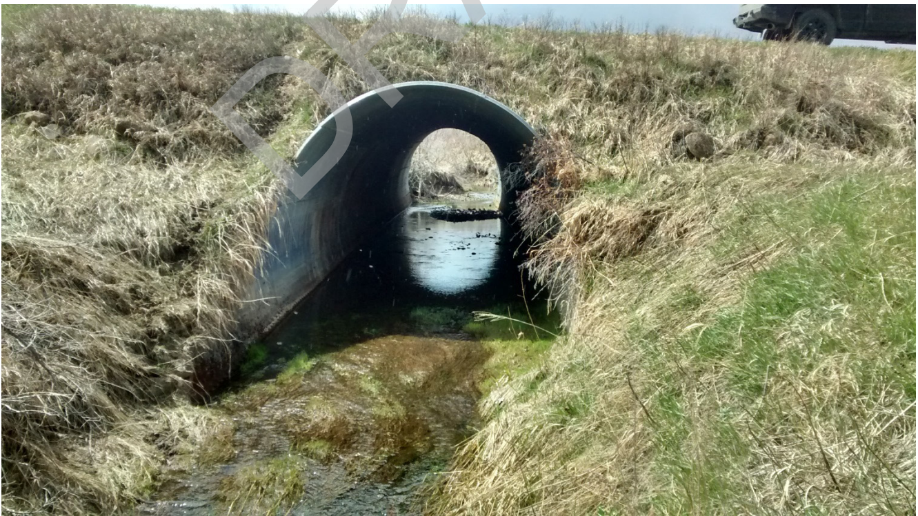
Photograph 40 Pipe Arch Culvert under Township Road 302, Location 22
