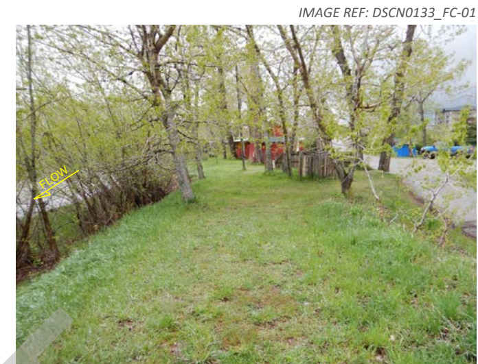
1. View looking upstream at the berm approximately midway along its length.
