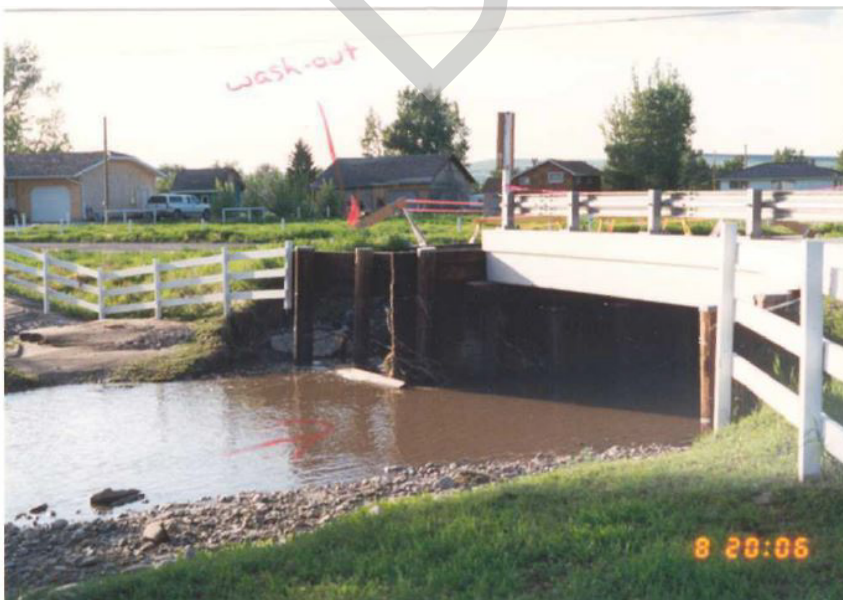
Figure IV.11 Washout Identified on Township Road 301 Bridge Over Kettles Creek
