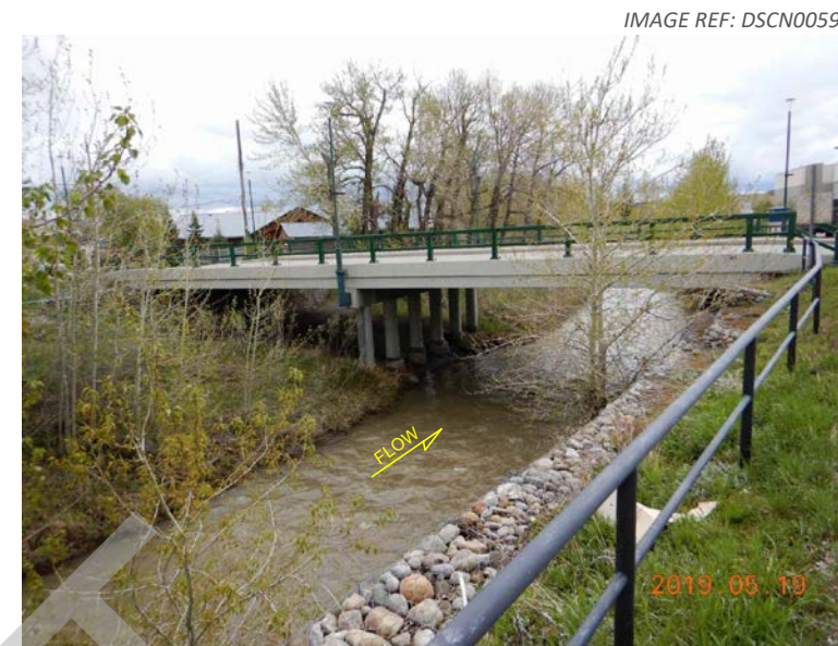
1. View looking downstream from the top of the right bank revetment.
