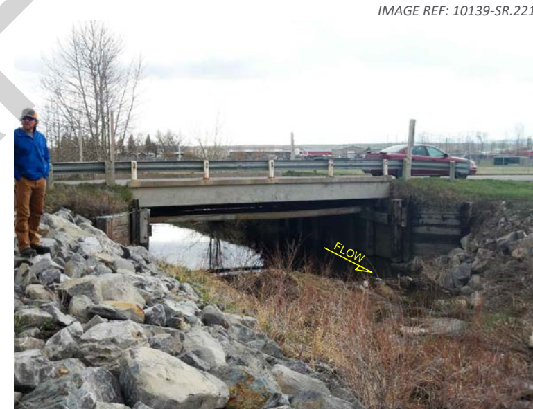
2. View looking upstream from right bank.
