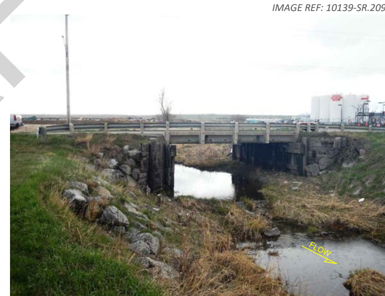
2. View looking upstream from right bank.
