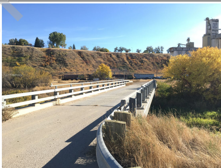
Bridge deck from the left bank approach
