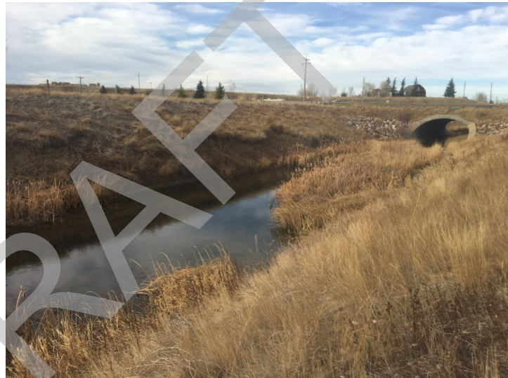
Upstream view from the right bank
