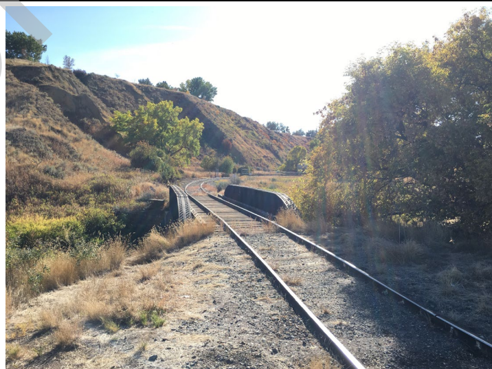
Bridge deck from the left bank approach
