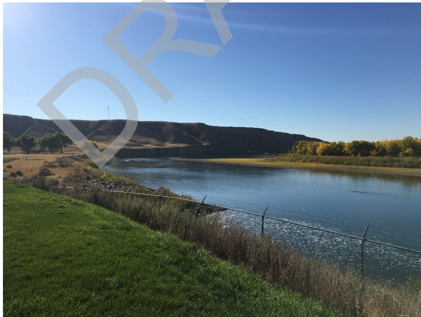
South Saskatchewan River (upstream view) from the wastewater treatment plant just downstream of planned cross section 57.
