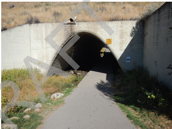
Upstream view of south culvert from trail
