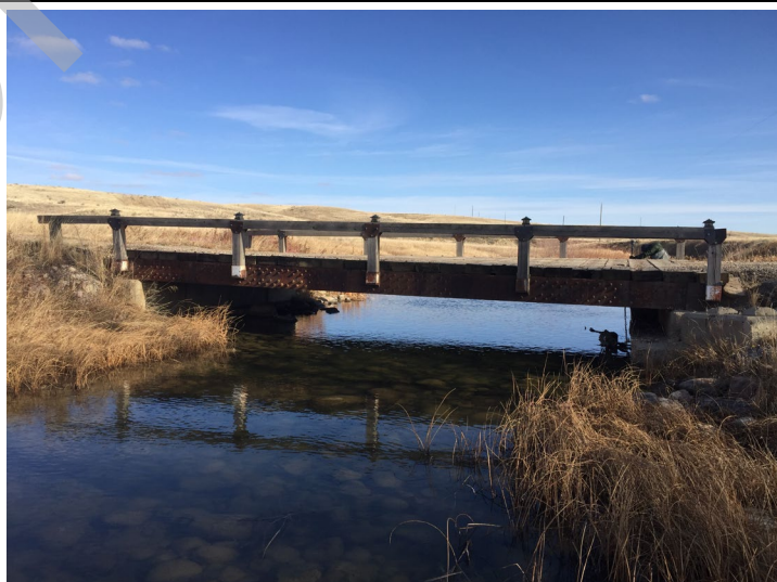
Downstream view from the left water edge
