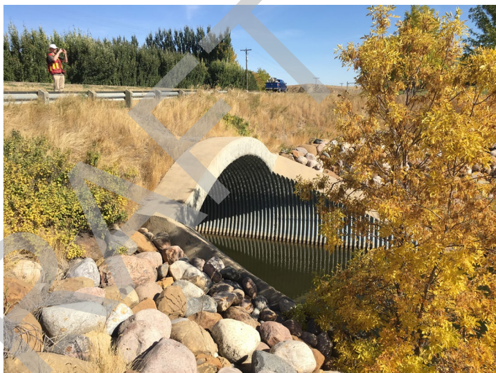
Upstream view of culvert from left bank
