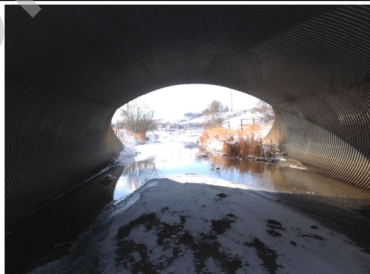
Culvert barrel looking upstream
