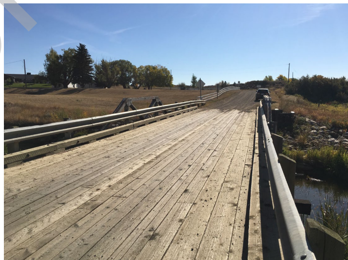
Bridge deck from the right bank approach
