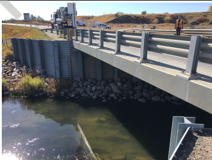
Downstream view from the left abutment
