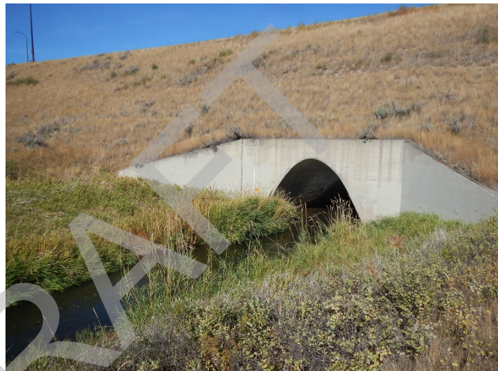
Upstream view of north culvert from right bank
