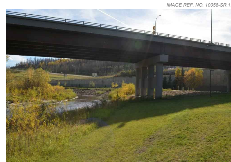
2. View looking downstream from right bank.
