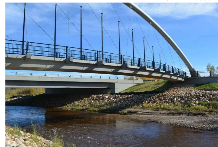
2. Pedestrian bridge in foreground. View looking downstream from left bank.
