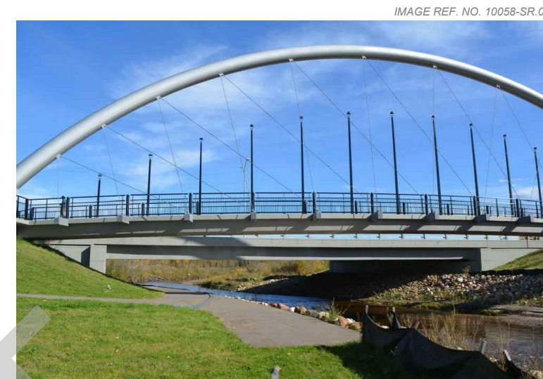
1. View looking downstream from left bank. Road bridge in background.
