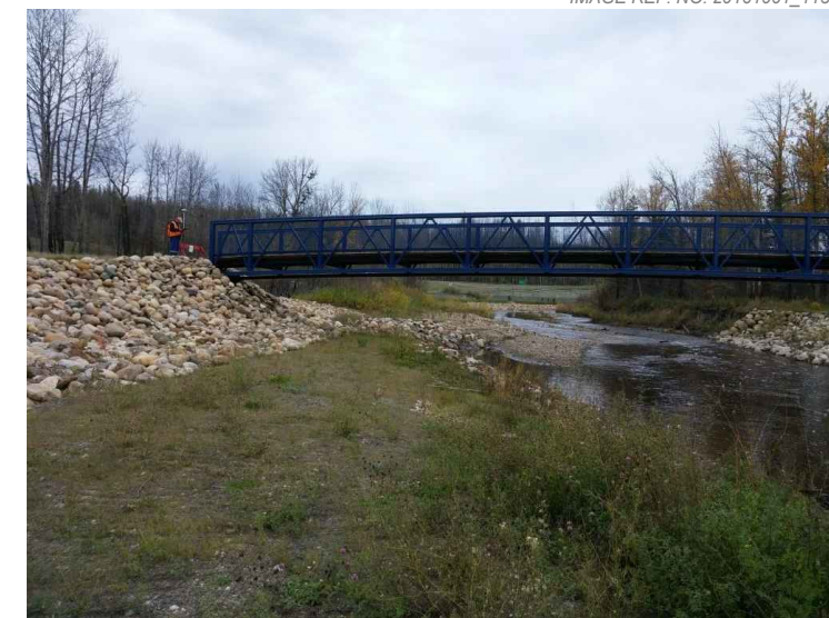
2. View looking upstream from right bank.
