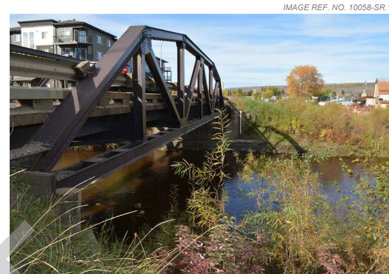
1. View looking from right bank. Flow is from left to right.
