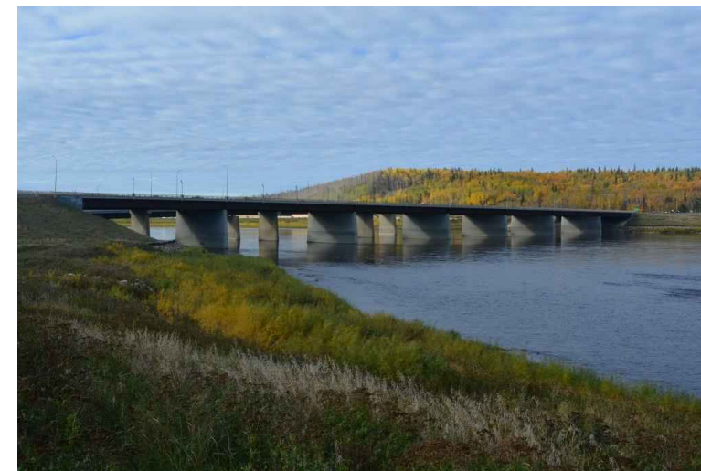
2. View looking upstream from right bank.
