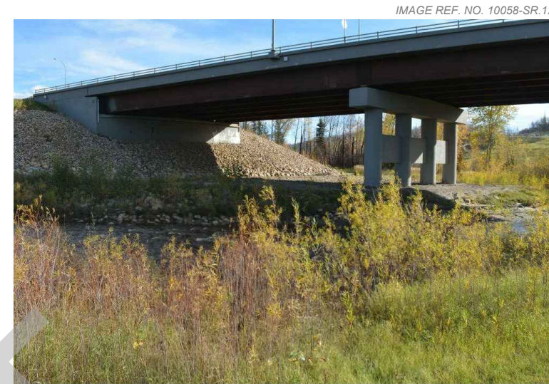
1. View looking downstream from right bank.
