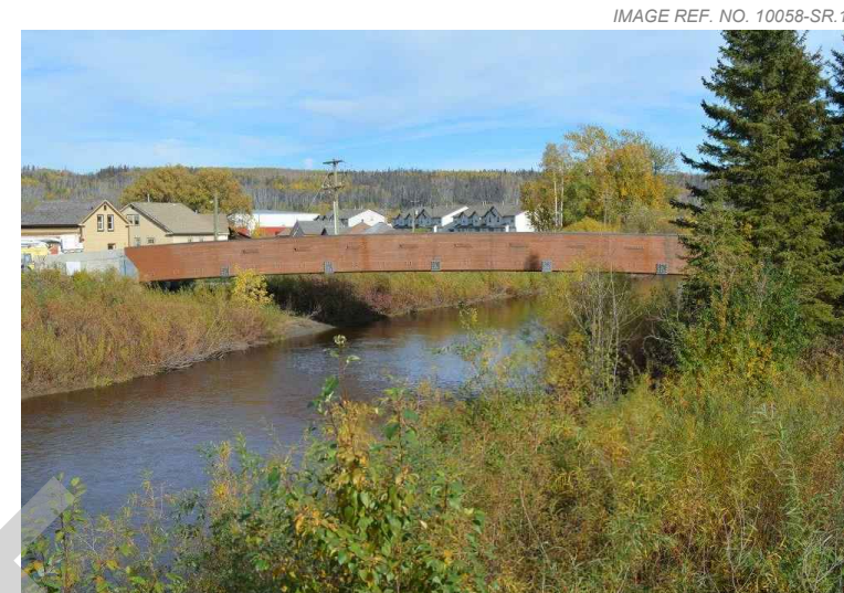
1. View looking downstream from right bank.
