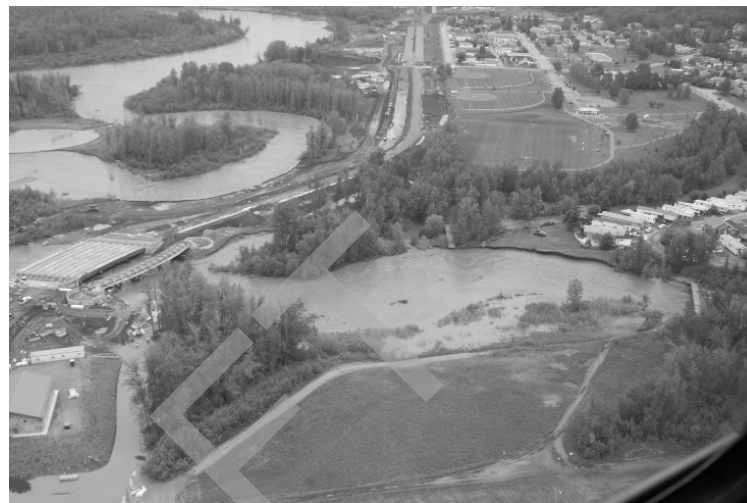
Figure 3: Aerial View showing the Hangingstone Confluence and Saline Creek Drive during the 2013 Flood
