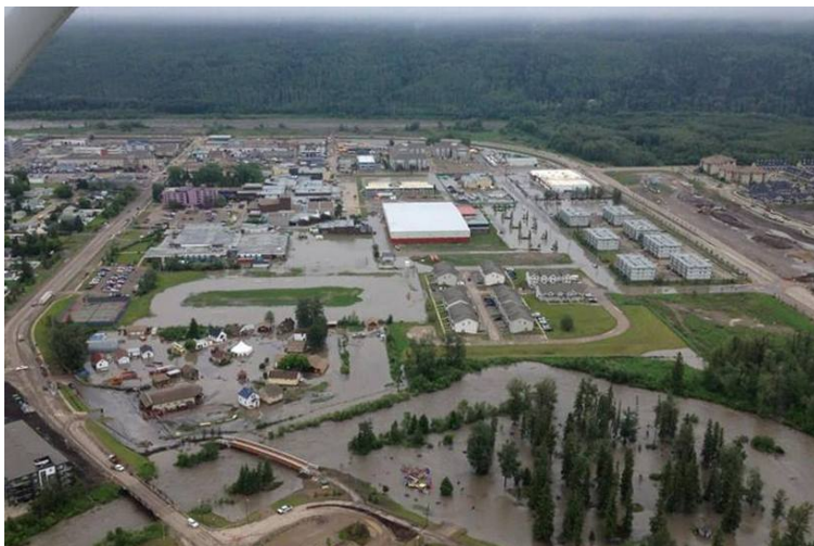
Figure 2: Aerial View of Inundation along the Lower Hangingstone during the 2013 Flood
