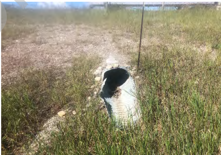
Downstream Side of Bridge
