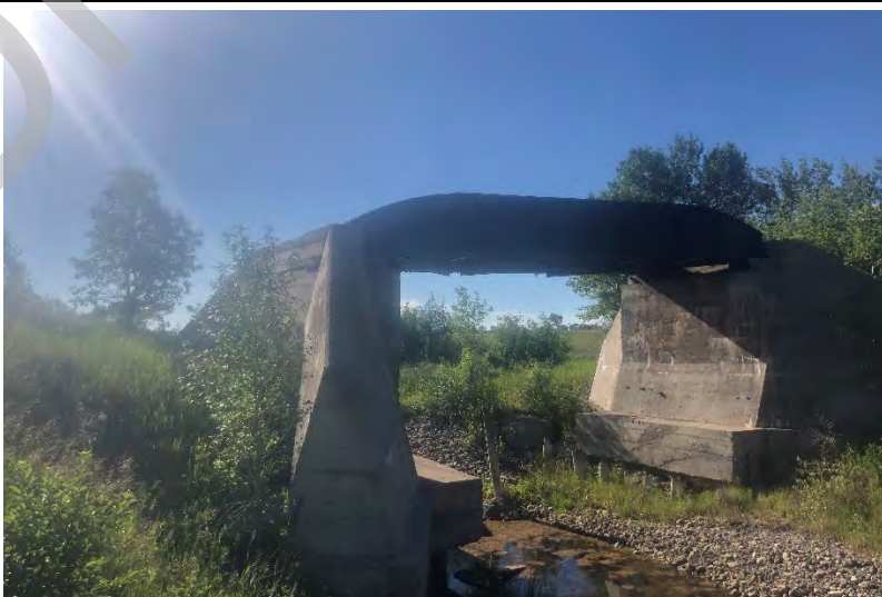
Downstream Side of Bridge
