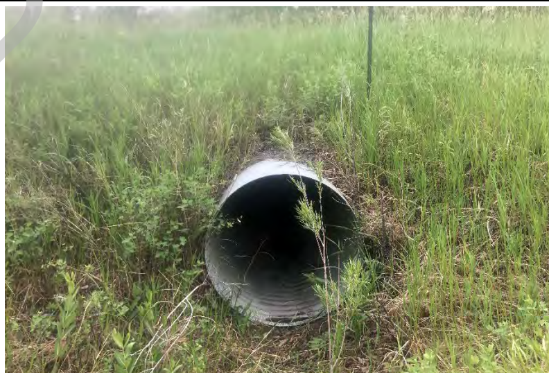
Downstream Side of Bridge
