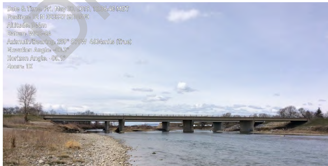
Downstrea m Side of Bridge
