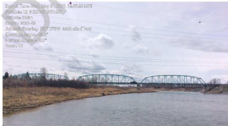
Downstream Side of Bridge
