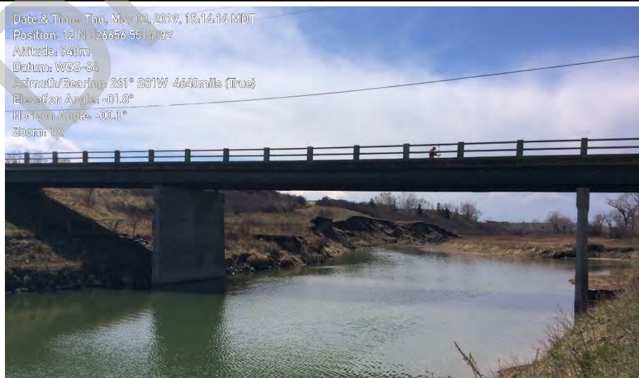
Downstream Side of Bridge
