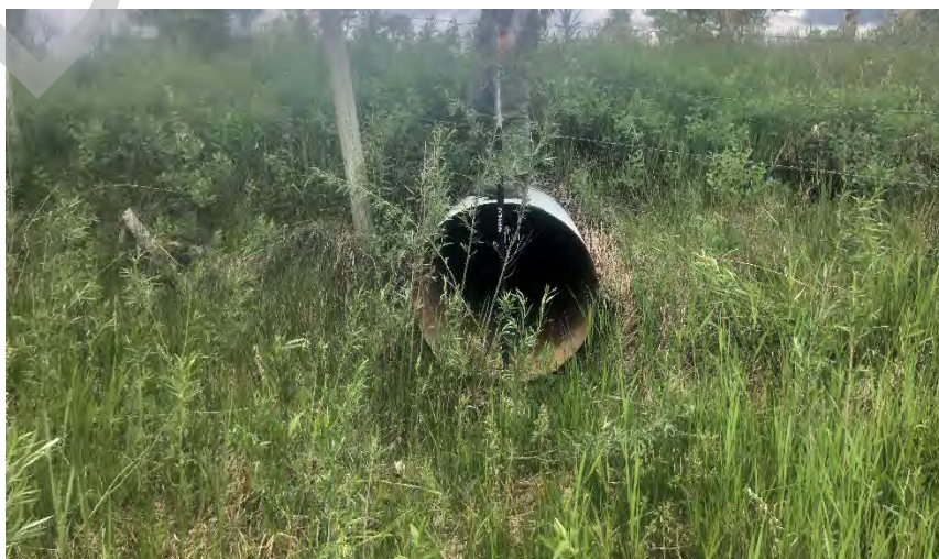
Downstream Side of Bridge
