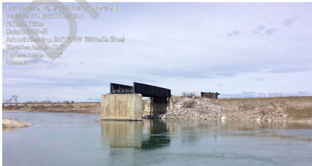
Downstream Side of Bridge
