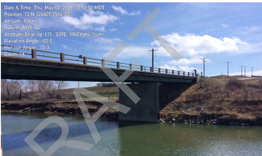
Upstream Side of Bridge
