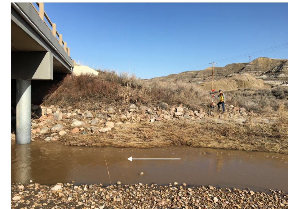
6. Surveying HWM upstream of Highway 10 Bridge along Willow Creek.
