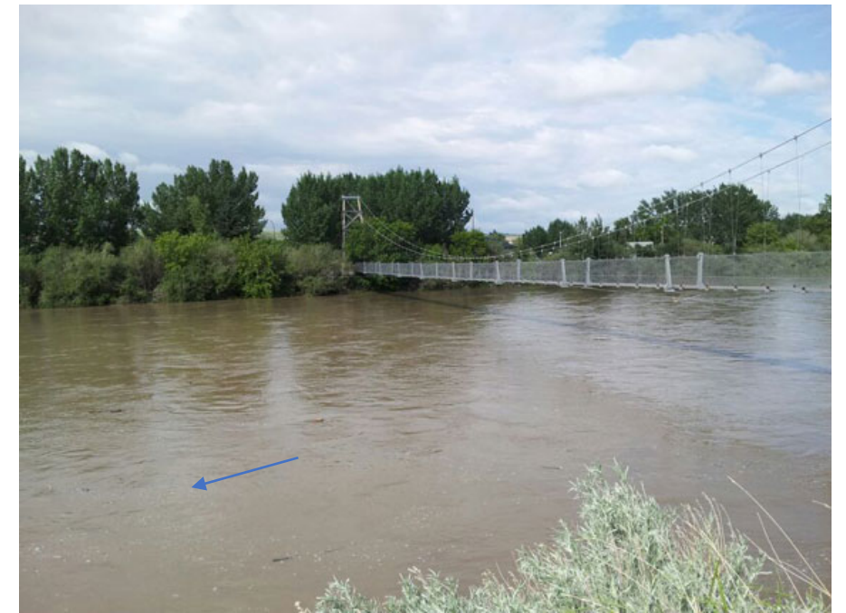
3. Star Mine Suspension Bridge in the Town of Drumheller.
