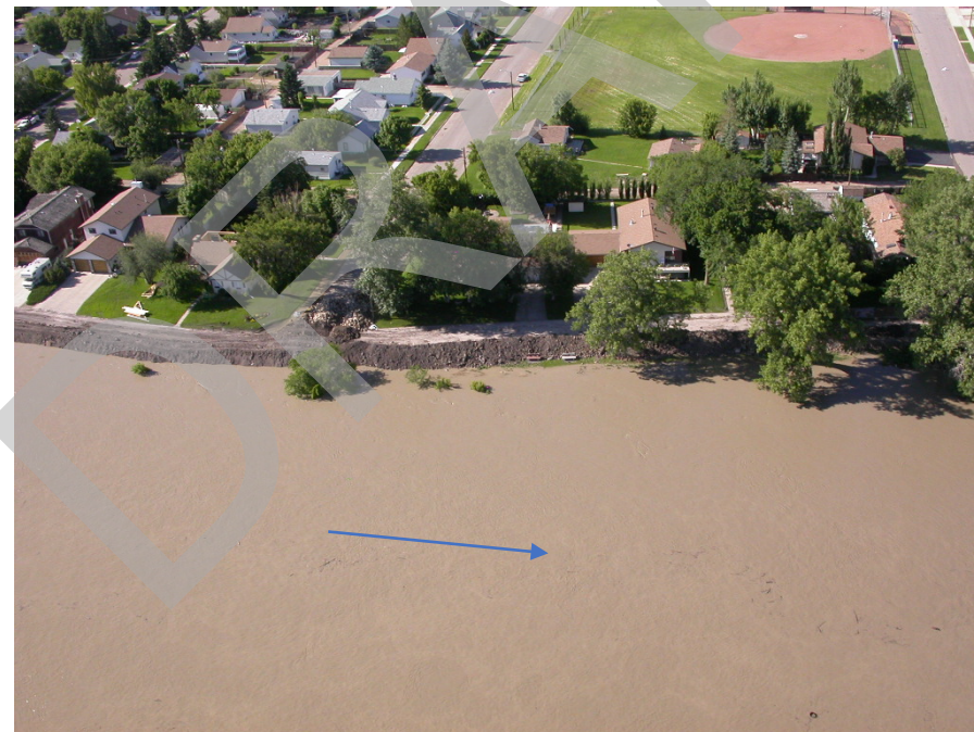
5. Temporary dike at 18th Street in the Midland area of the Town of Drumheller.
