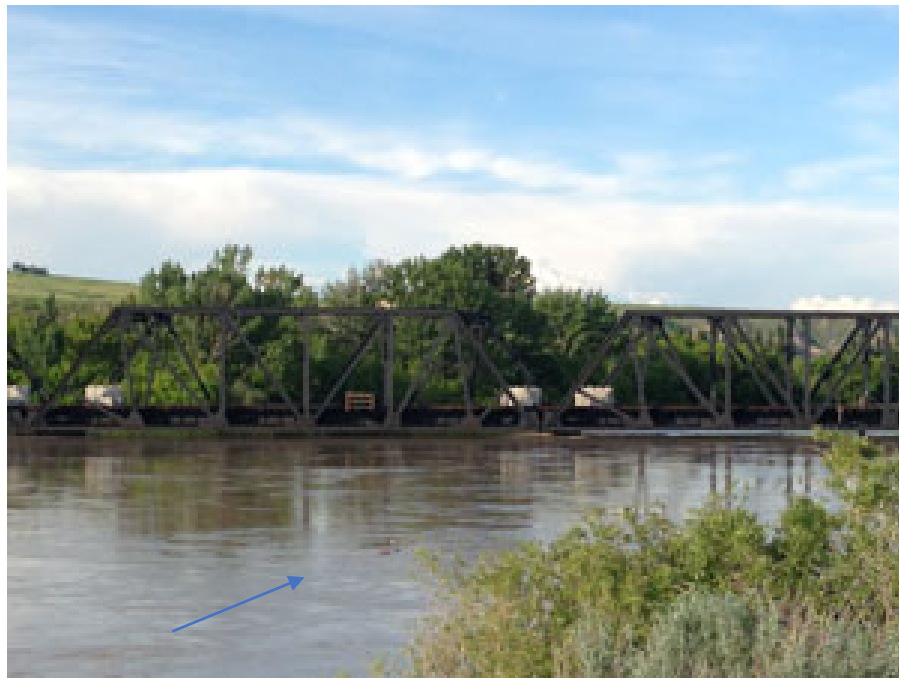
1. Newcastle Mine Railway Bridge in the Town of Drumheller.
