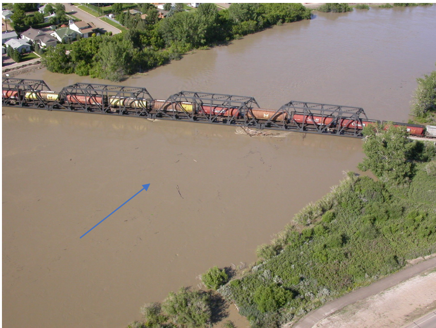
4. Newcastle Mine Railway Bridge in the Town of Drumheller.
