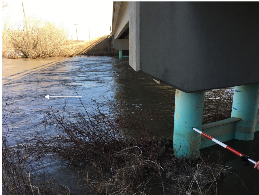
1. Surveying HWM at Highway 575 Bridge along Kneehills Creek.
