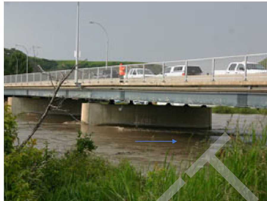
2. Highway 56 Bridge in the Town of Drumheller.
