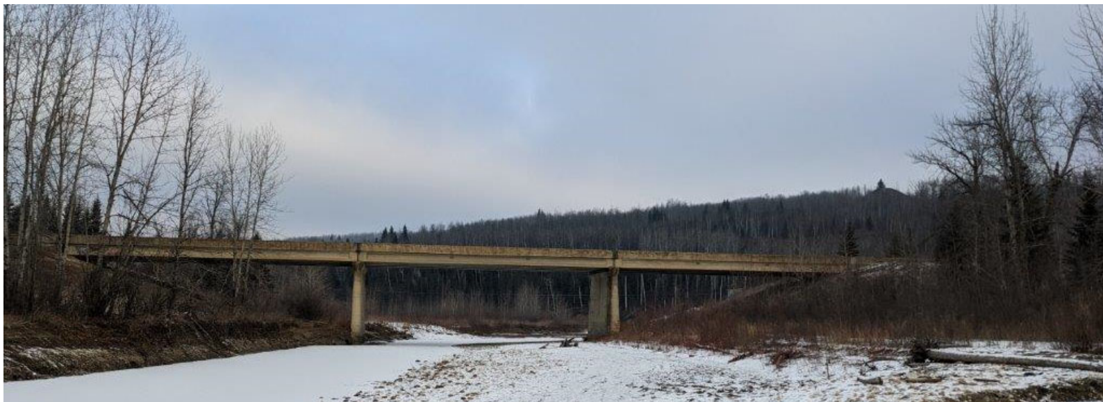
Highway 64 Clear River Bridge Looking North
