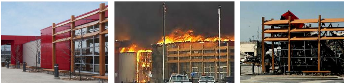
Figure 1.17 Slave Lake Government Centre and Library – Building pre-fire, during fire and post fire
