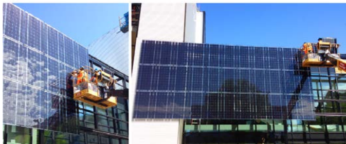
Figure 9 – Integrated solar panels – PAW Building, University of Alberta
