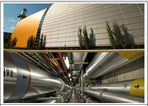
Figure 10 – University of Alberta's North Heating and Cooling Plant (above) and mechanical distribution network in underground utility corridors (below) – Photo credits – University of Alberta.
