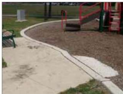
Curb ramp into play space where there is a level change between accessible route and play space.
