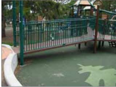
Ramp connected to elevated play components.
