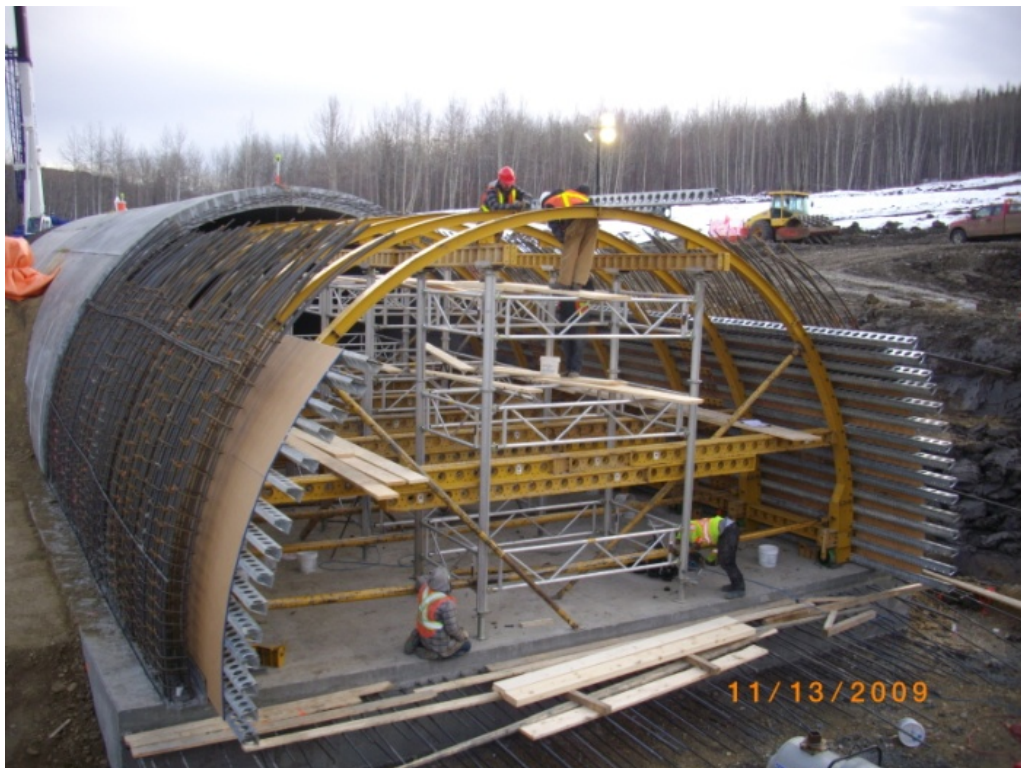
Figure 10: Setting Steel Arch Formwork and Scaffolding on Completed Base Slab
