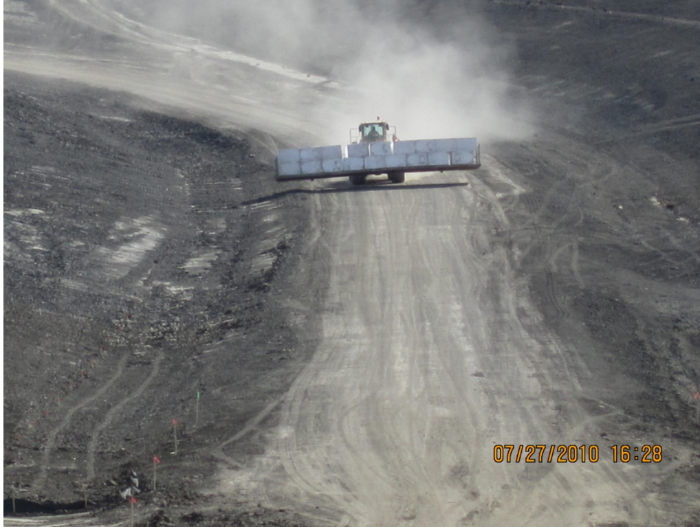
Figure 12: Wheel Loader with Attachment Transporting EPS Geofoam for Placement
