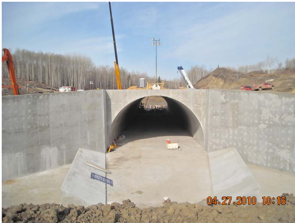
Figure 11: Nearly Completed Ksituan River Culvert
