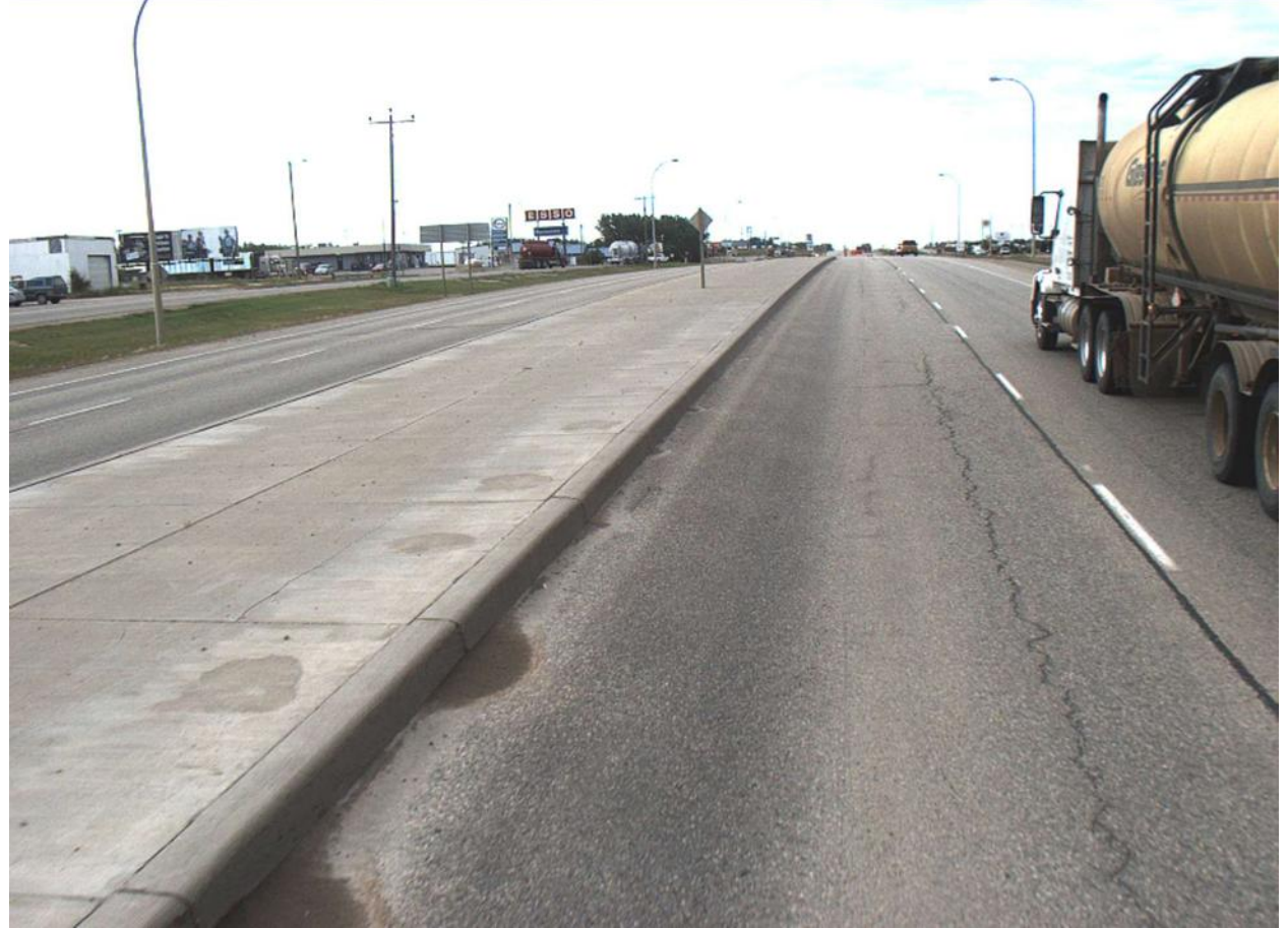
Town of Valleyview - Median with Barrier Curb
