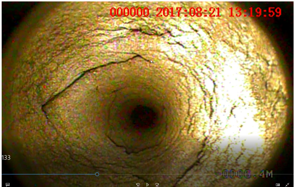
Figure 6. Image from 2017 downhole-video-camera survey of metal-capped borehole
