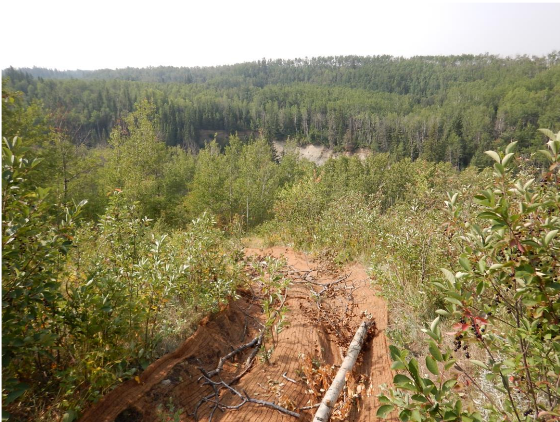
Figure 9. Erosion control blanket and woody debris on old trail (view from top of bank)
