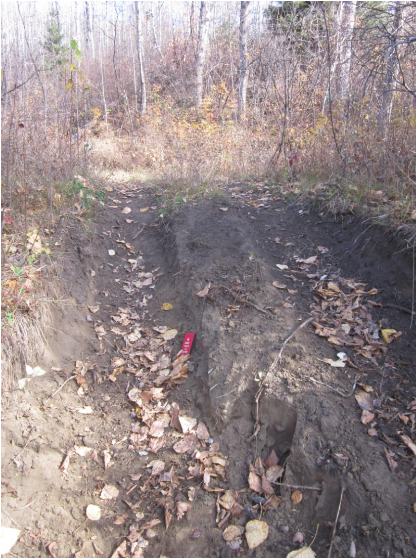
Figure 4. Deeply eroded OHV trail (red phone for size reference)
