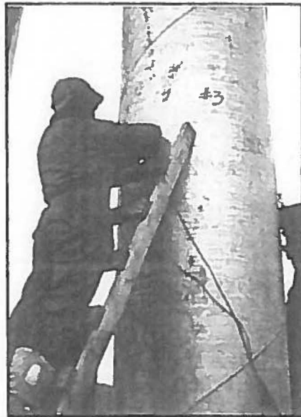
Figure 6. Attaching Strain Gauges and Accelerometers to Pile # 3
