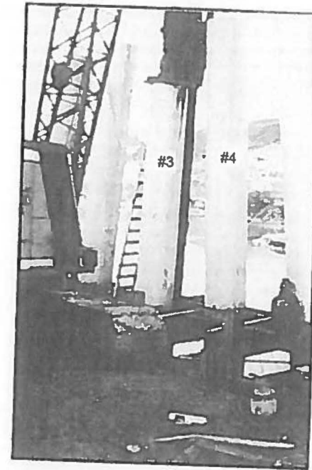
Figure 7. Pile Driving in Progress
