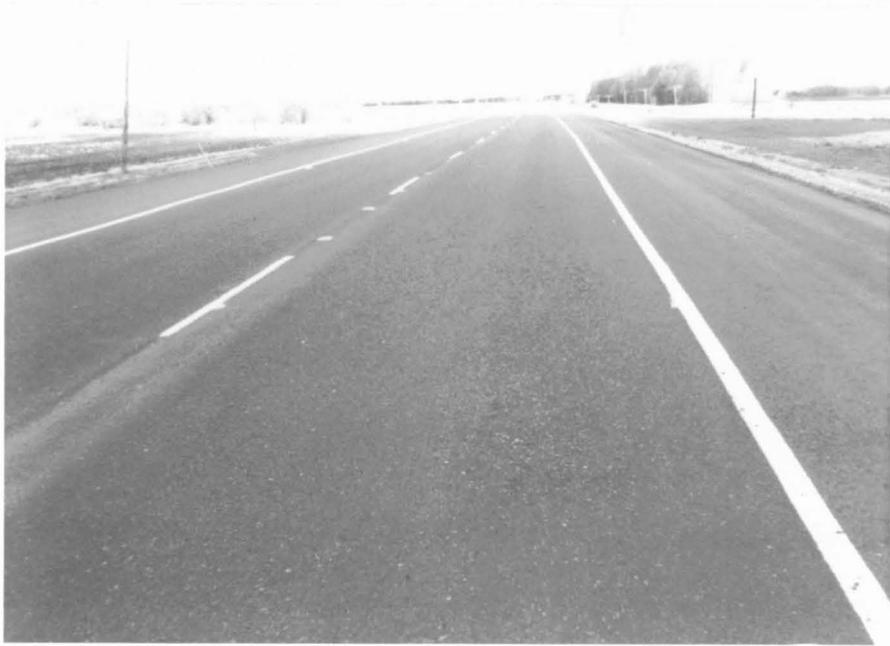
**Figure 5: Pavement Surface Texture Due to Loss of Fine Aggregate**
