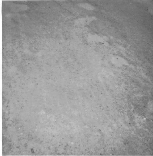
**Figure 7: Severe Ravelling**
