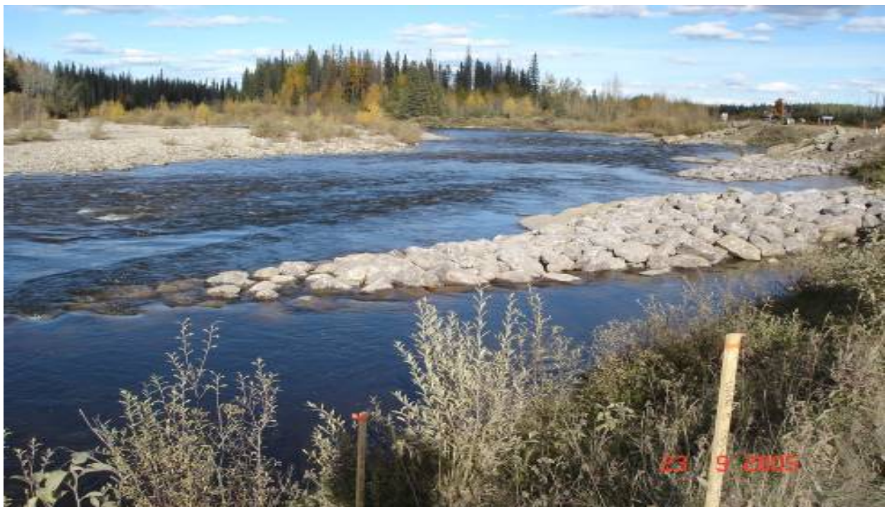
Photo 3 Construction of Redirective Vanes
