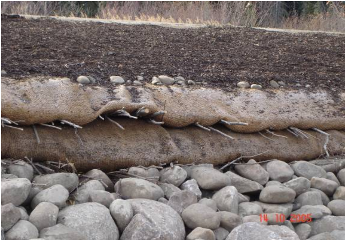
Photo 7 Vegetated Mechanically Stabilized Earth
