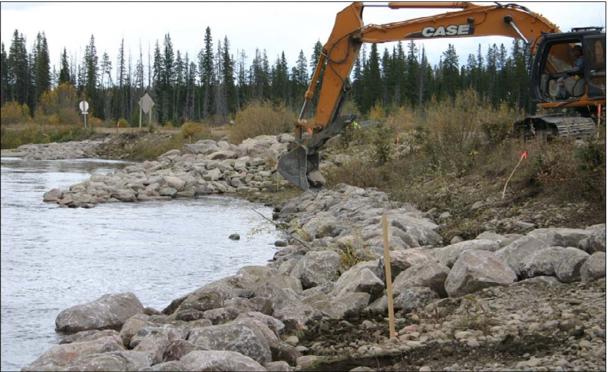
Photo 4 Construction of Longitudinal Peak Stone Toe Protection
