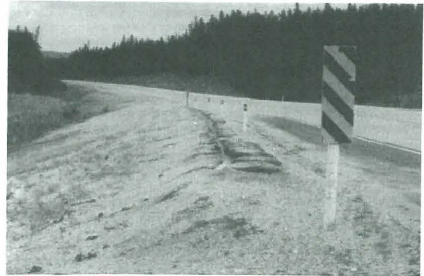
Figure 9. Recent Photograph of Pile Wall and the Highway
