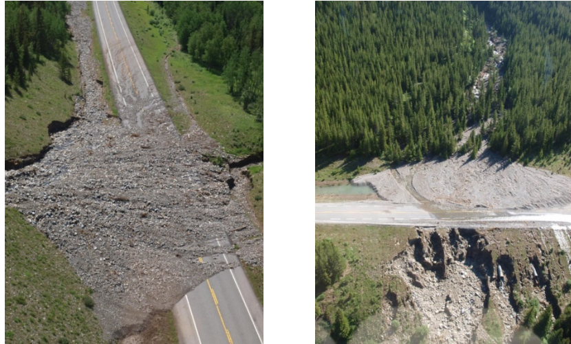
Figures 3 and 4: Debris Flow Causing Road Blockage, Culvert Plugging and Erosion (Highway 40)
