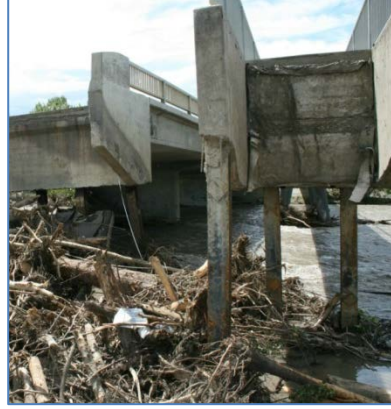
Figures 7 and 8: Loss of Headslope at Bridge Locations (Elbow River, Hwy 66 and Sheep River, Hwy 22)
