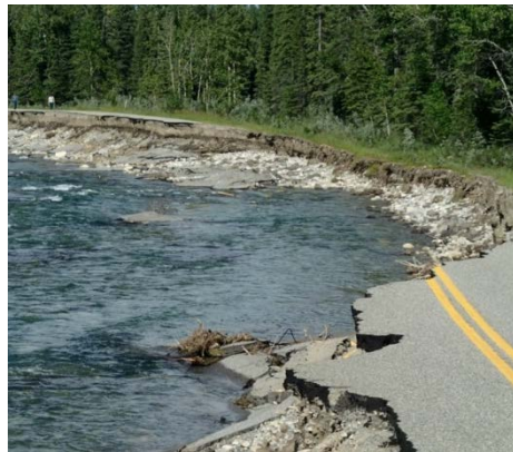
Figures 9 and 10: Examples of Complete and Partial Road Washout (Highway 758 Elbow River, Hwy 40, Highwood River)
