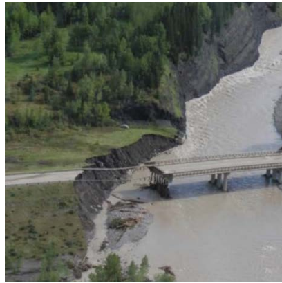
Figures 7 and 8: Loss of Headslope at Bridge Locations (Elbow River, Hwy 66 and Sheep River, Hwy 22)
