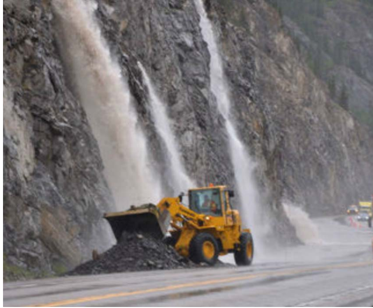
Figure 12: Example of Rock Cut Flushed by Rainfall (Highway 3)
