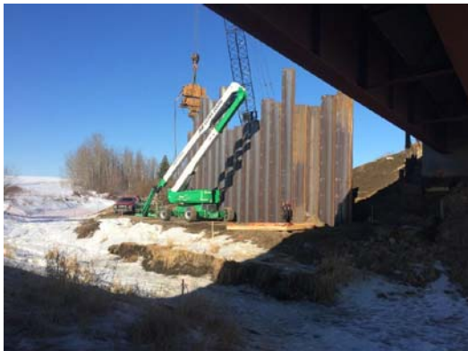
Figure 6b. Installation of Sheet Pile Wall 'A'
