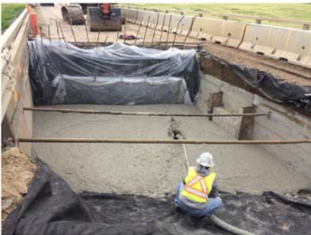
Figure 10. Placement of Cellular Concrete
