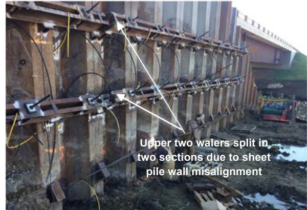
Figure 7. Waler Installations on Pile Wall 'B'
