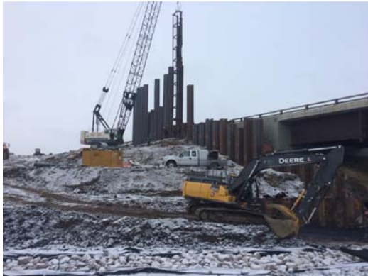
Figure 6c. Installation of Sheet Pile Wall 'B'
