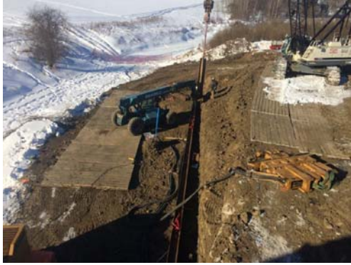
Figure 6a. Guide Beam Installation
