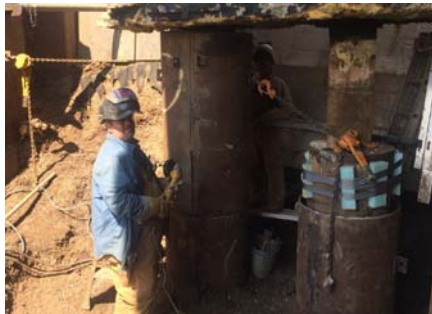
Figure 9. Installing Casings Around Impacted Piles
