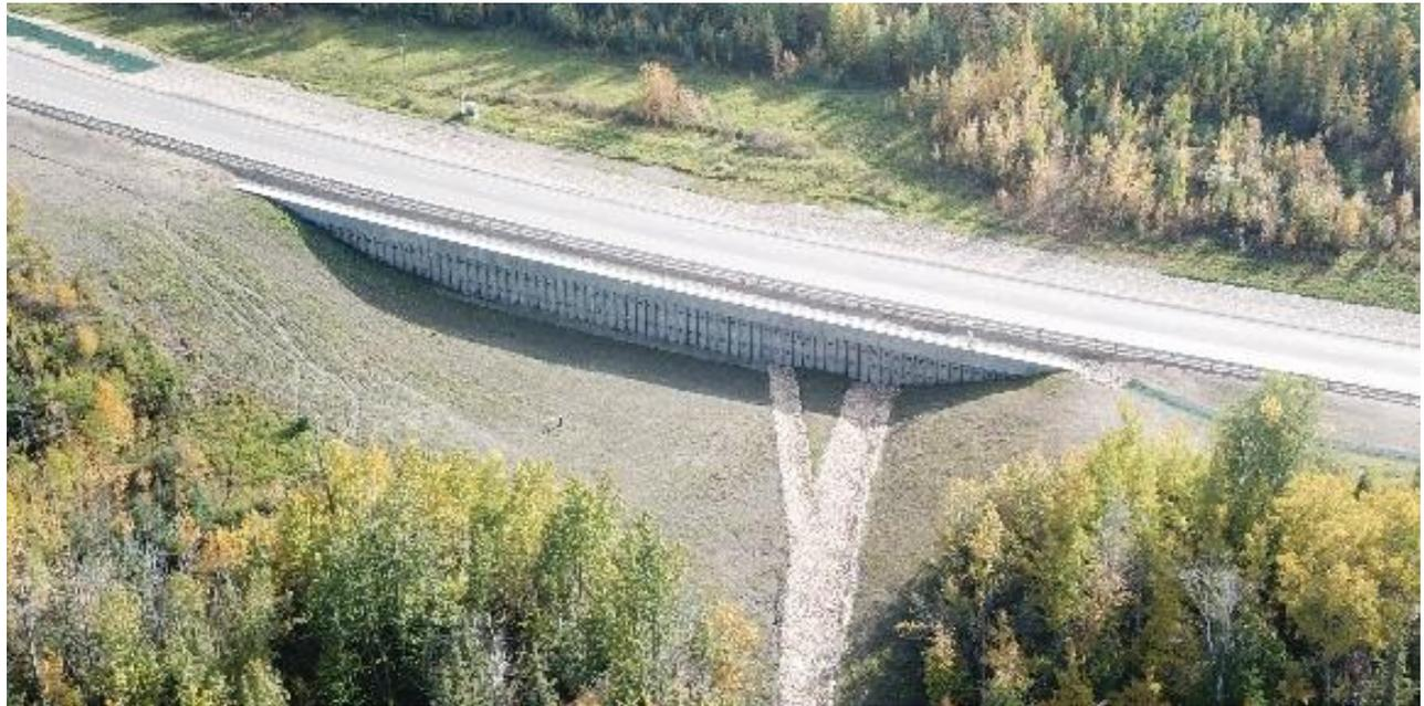
Figure 4 Drone view of the completed pile wall
