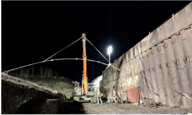
Figure 3. Nighttime anchor installation
