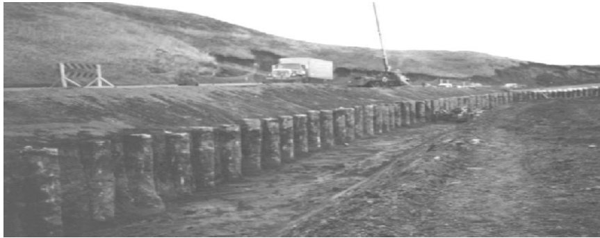
FIG.7. Installed Vertical Piles
