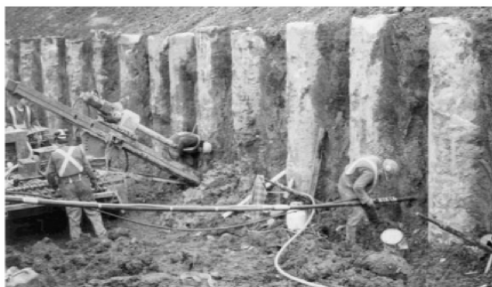
FIG.8. Installation of Tie-Backs
