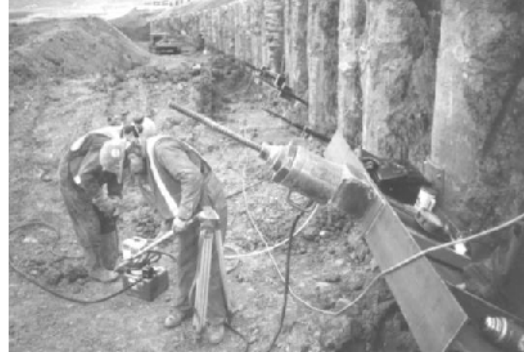
FIG.11. Tie-back test Set-up
