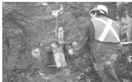
FIG.9. Installation of Waler Seat
