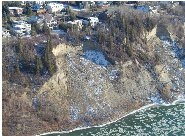
Figure 2. Landslides threatening luxury homes on the North Saskatchewan River in southwest Edmonton
