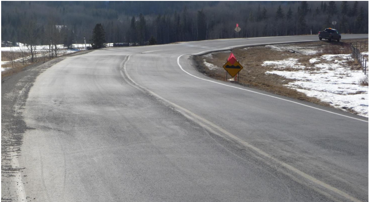
Figure 3. Photo of roadway looking SW, 2016
