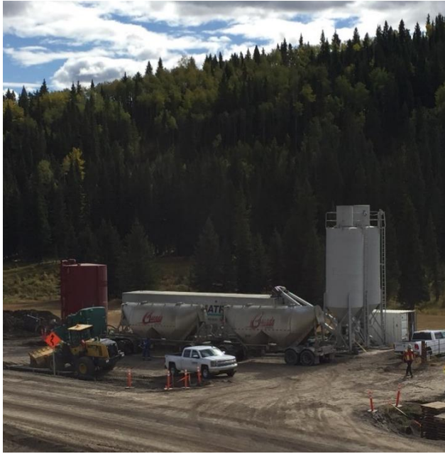
Figure 7. Photo of Dry mix unit with cement bulker onsite
