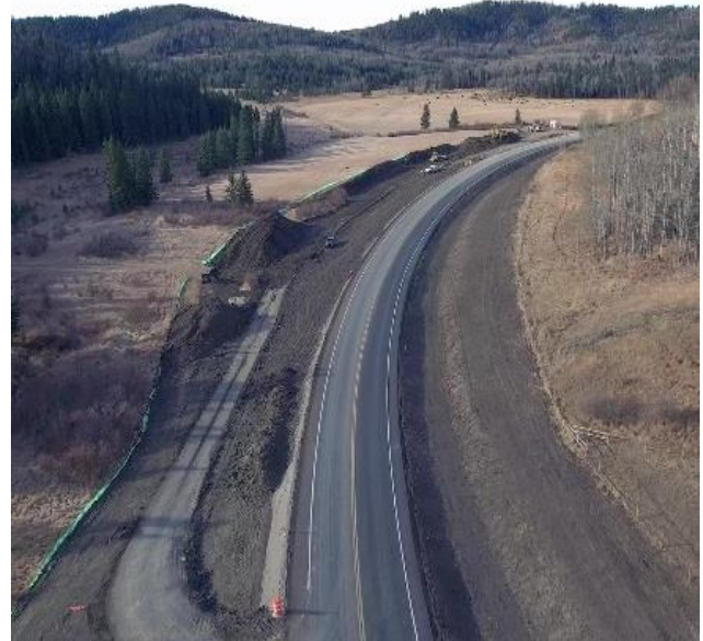
Figure 10. Photo after placement of asphalt
