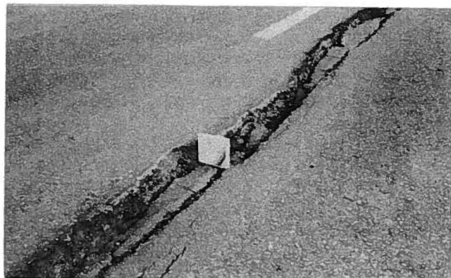
Photo 3: Cracking and Displacement of Roadway
