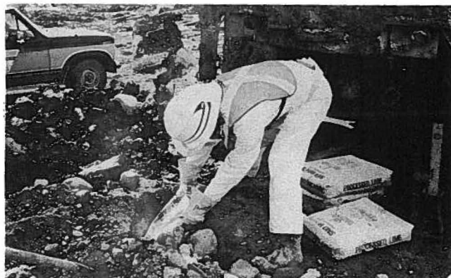
Photo 4: Addition Of Lime To Form Base Plug
