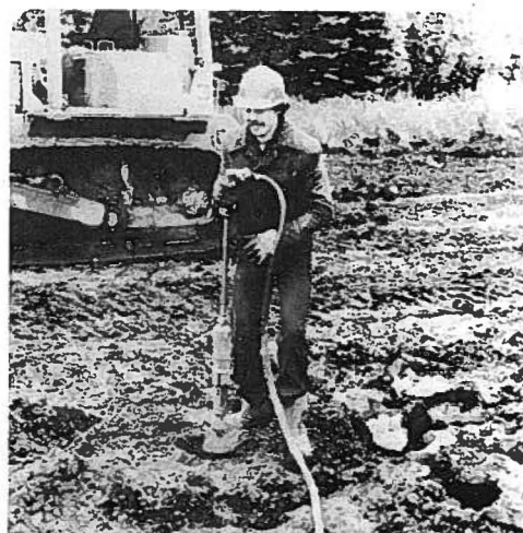
Photo 2: Hand Tamper For Surface Compaction
