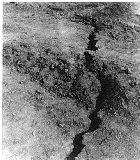
Photo 12: Cracks In Headslope
