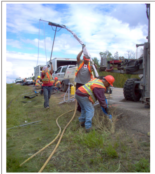
Photo 3. Containment unit assembly and installation
