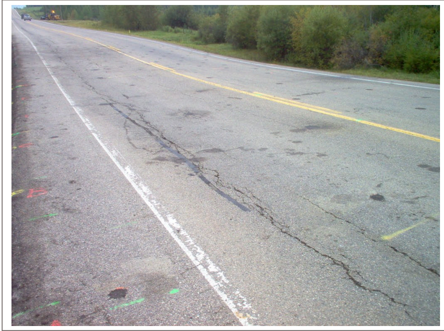
Photo 6. Site after foam injection, looking south. Notice asphalt patched injection points
